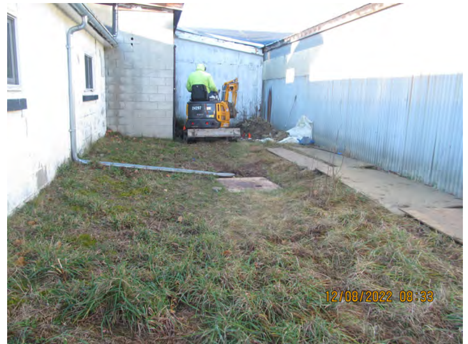
excavating to find sewer line
