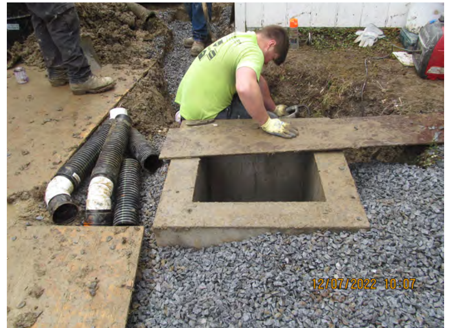
core drill cb02 for lines
