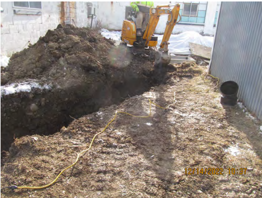
excavation to CB07
