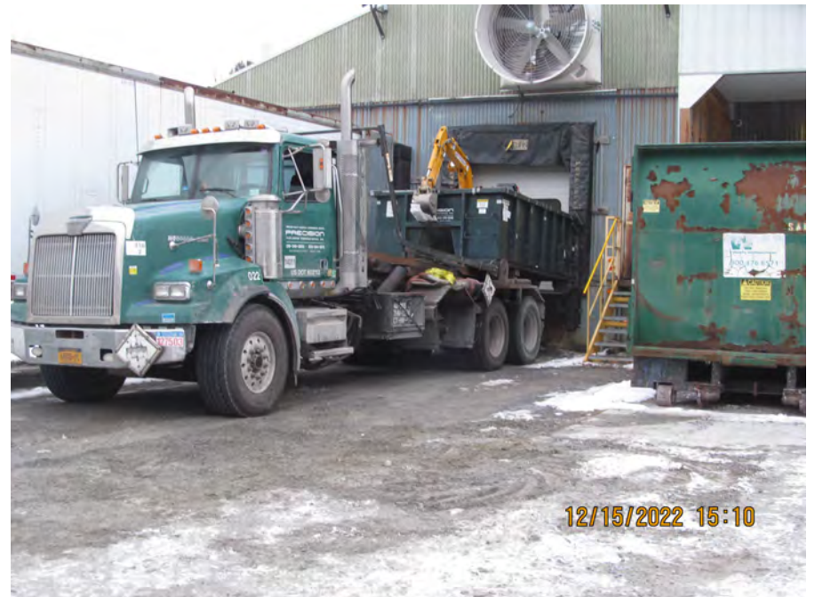
pull exc out for line pit
