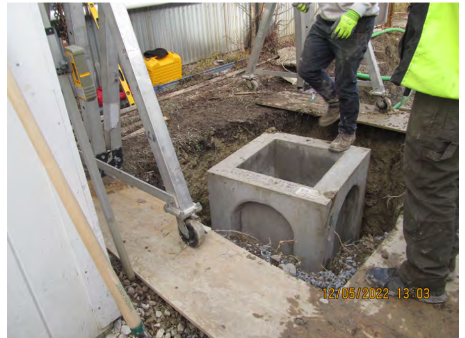
CB02 in place
