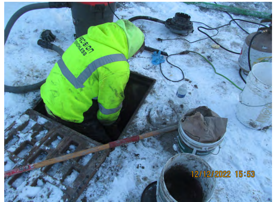
plugging hole cb9
