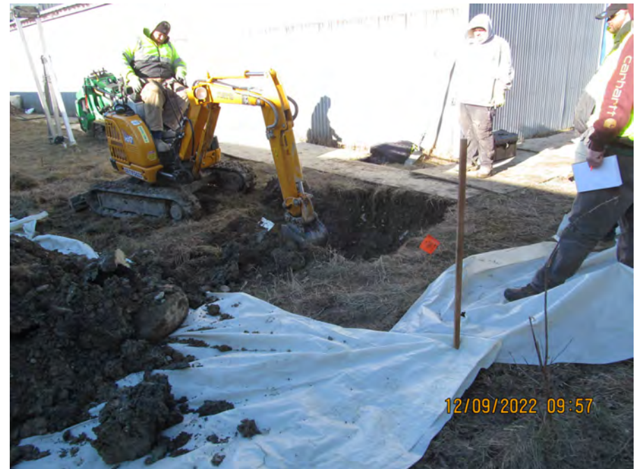
separate material form exc
