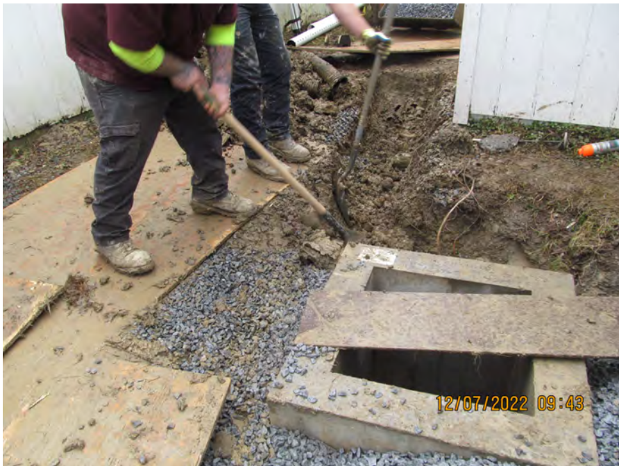
hand dig for 4 inch lines
