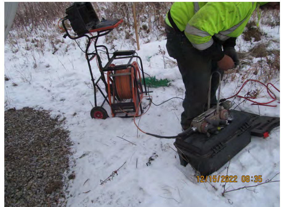
camera survey 6 inch line from discharge
