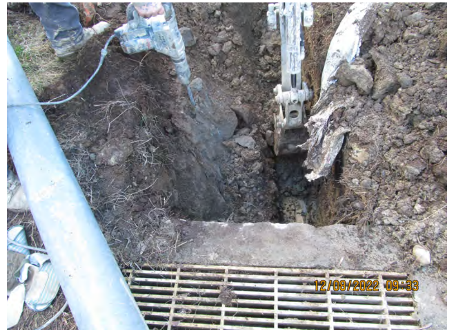
removing grout from cmp
