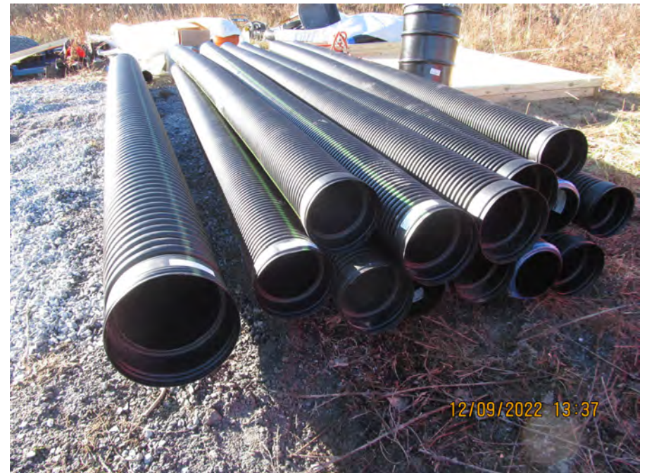
pipe delivery from ej prescott
