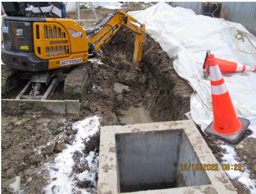
cleaning out slough material
