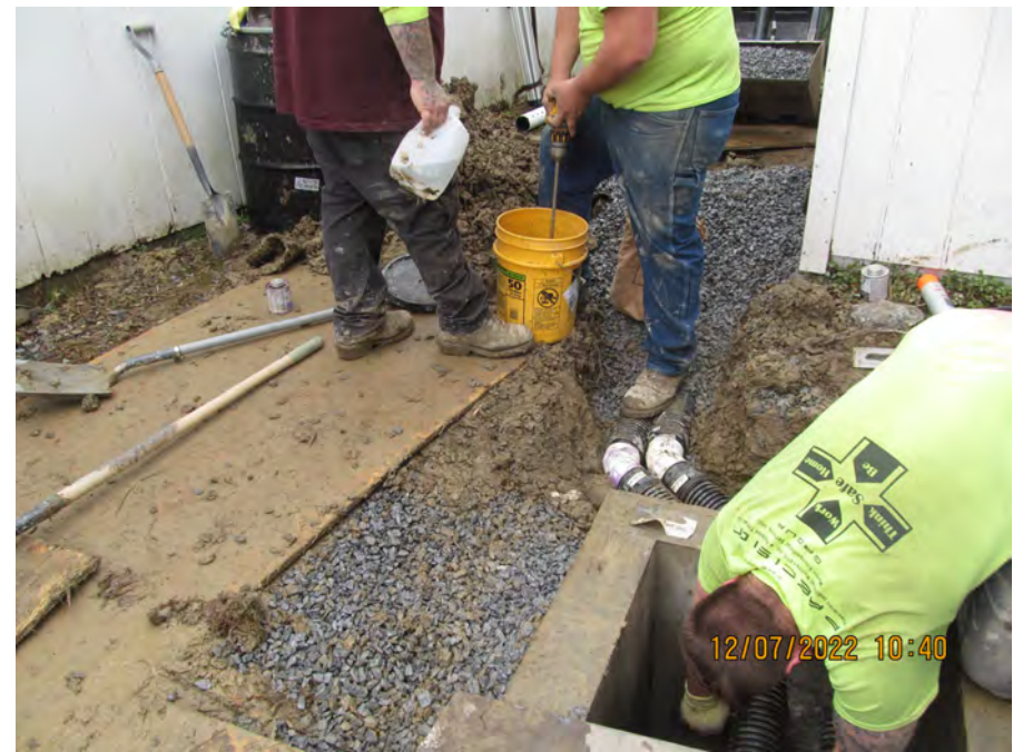
grouting lines into place
