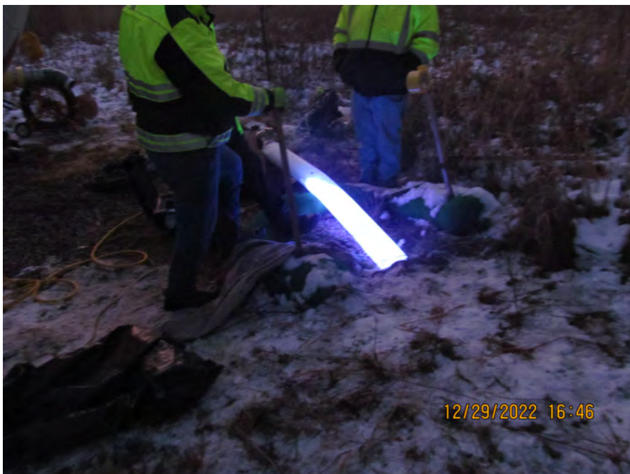
curing last section
