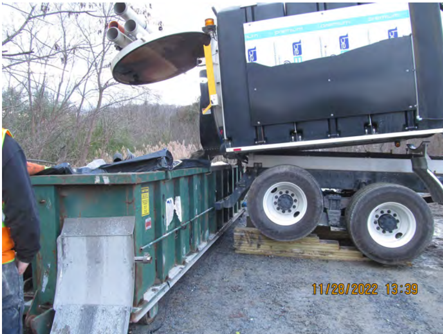
vac truck decon into rolloff
