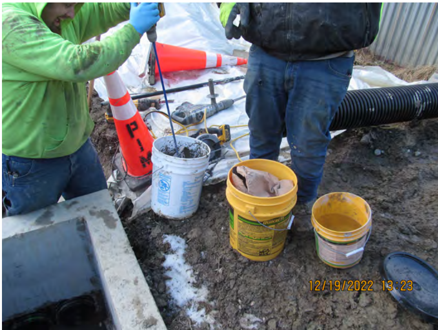
grout for pipes cb7
