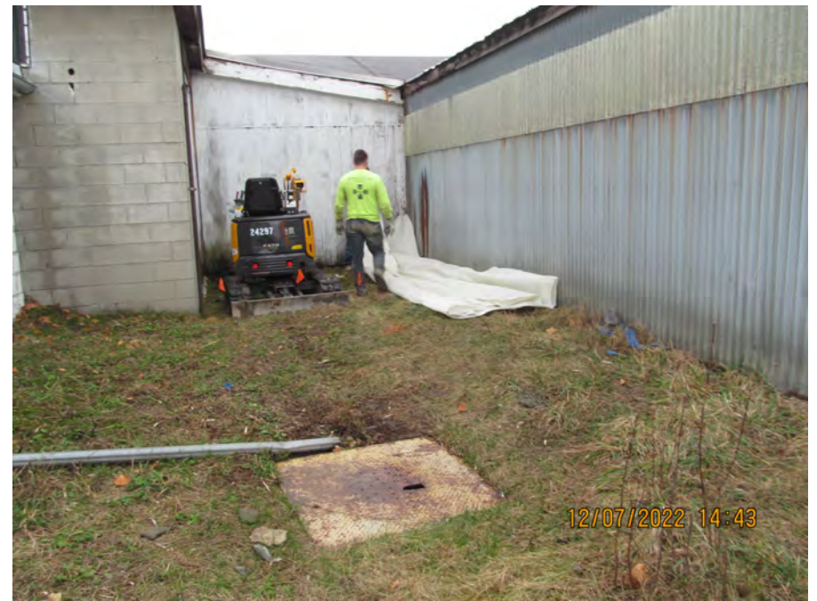
placing poly for spoils
