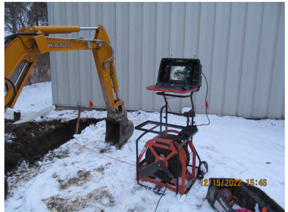
camera survey 6 inch line from inlet
