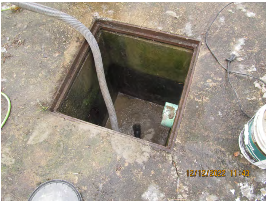
checking leaks cb4
