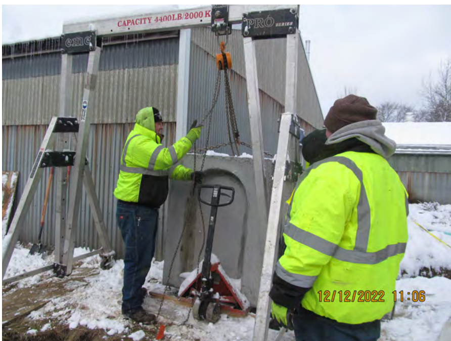
moving cb7 into place
