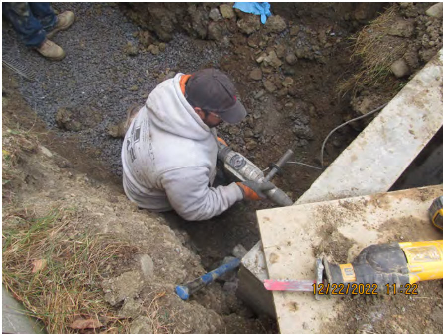
core drill 12 inch outlet cb8
