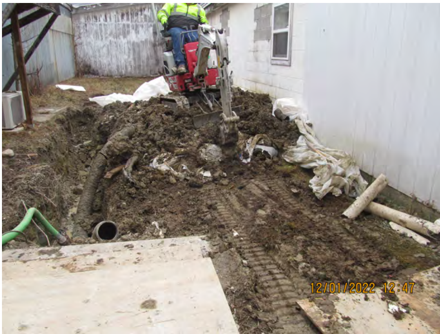
continue to excavate and loadout spoils
