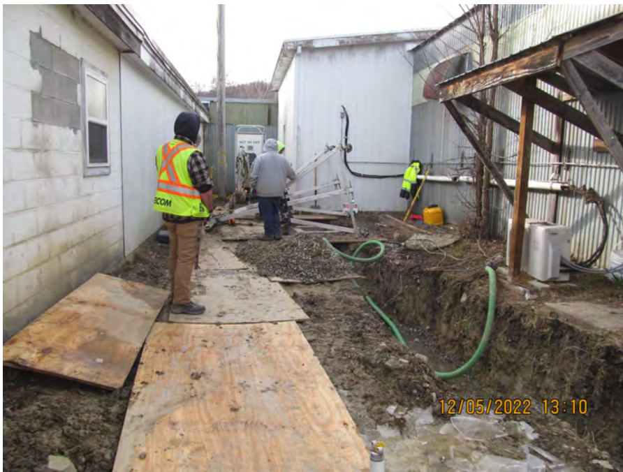
break down frame and chain fall
