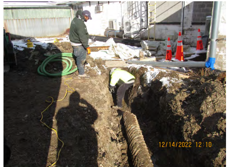
continue core drilling to widen outlet
