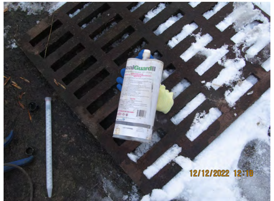
grout cb4 for stopping leaks
