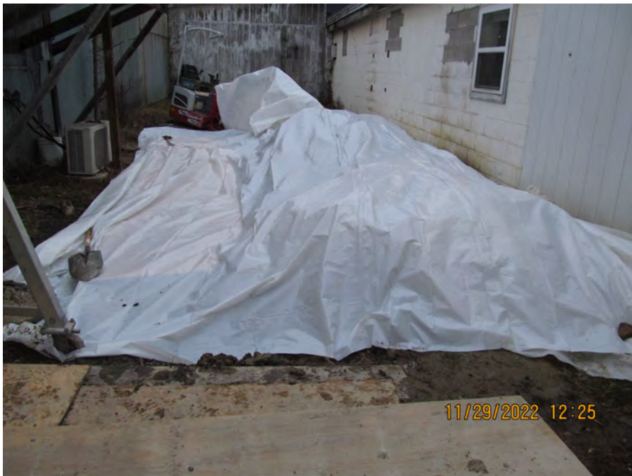
plastic cover trench and spoil pile
