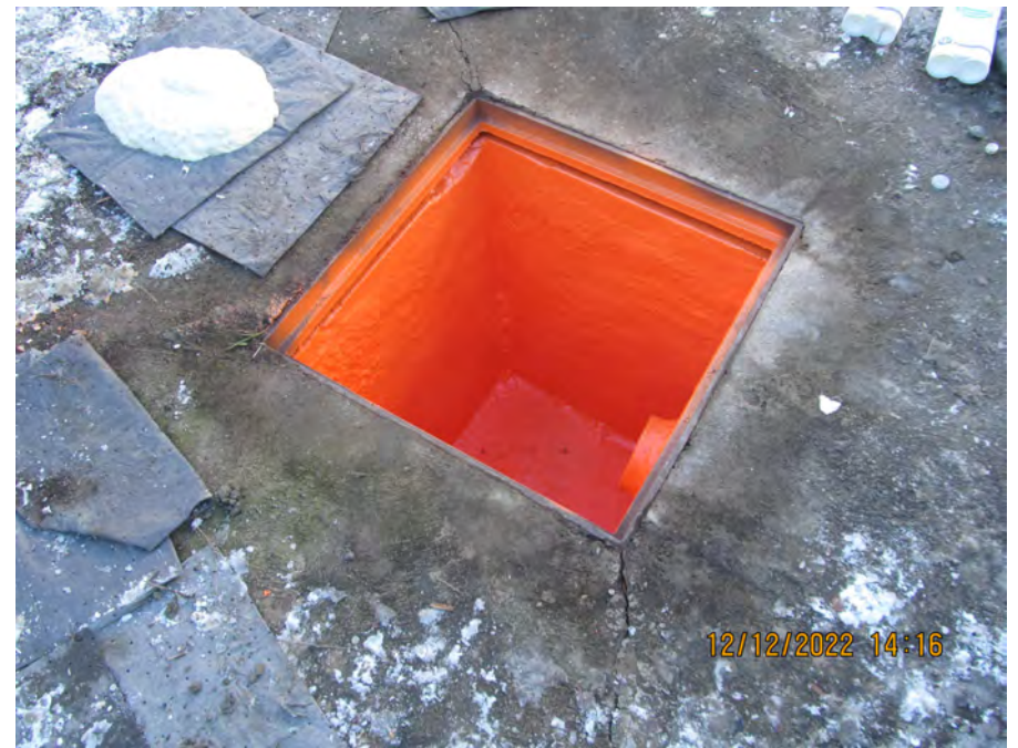
cb4 liner installed
