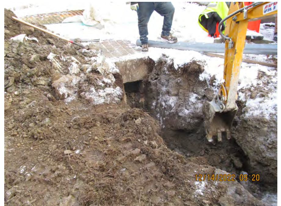
removed cmp section and excavation
