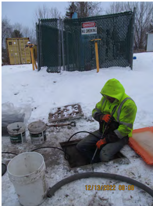
drying catch basin for install
