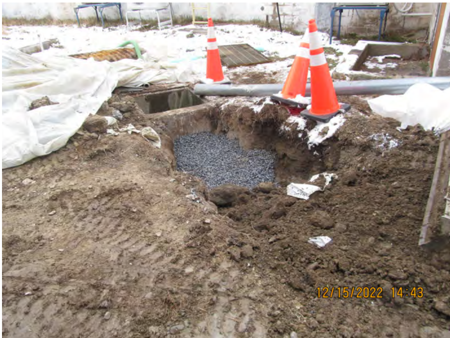
cb6 stone and backfill end
