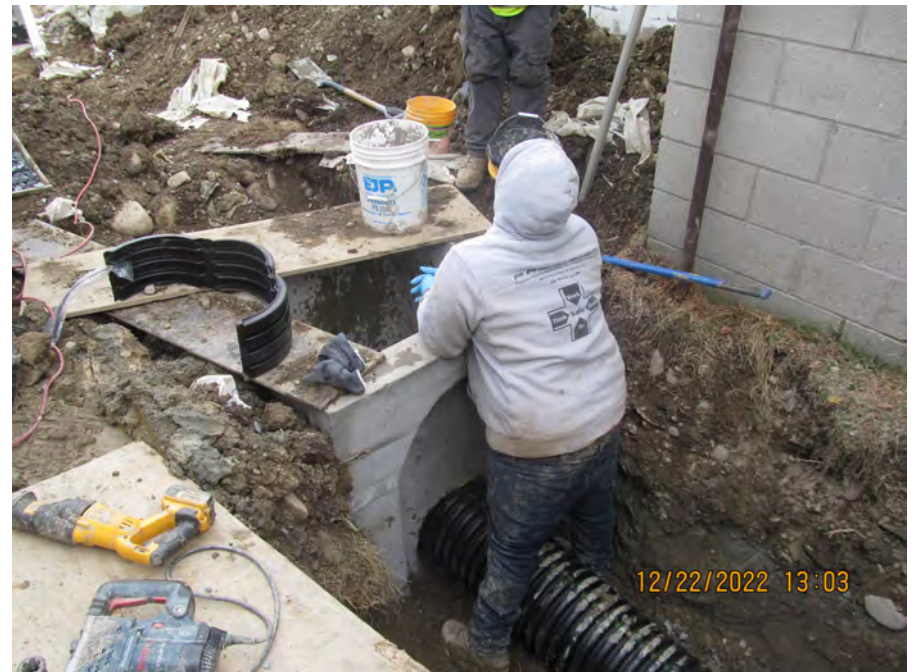
grouting outlet cb8
