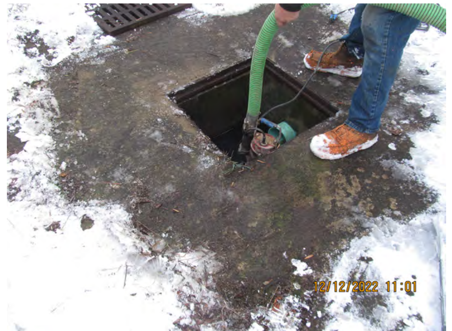
pumping out cb4
