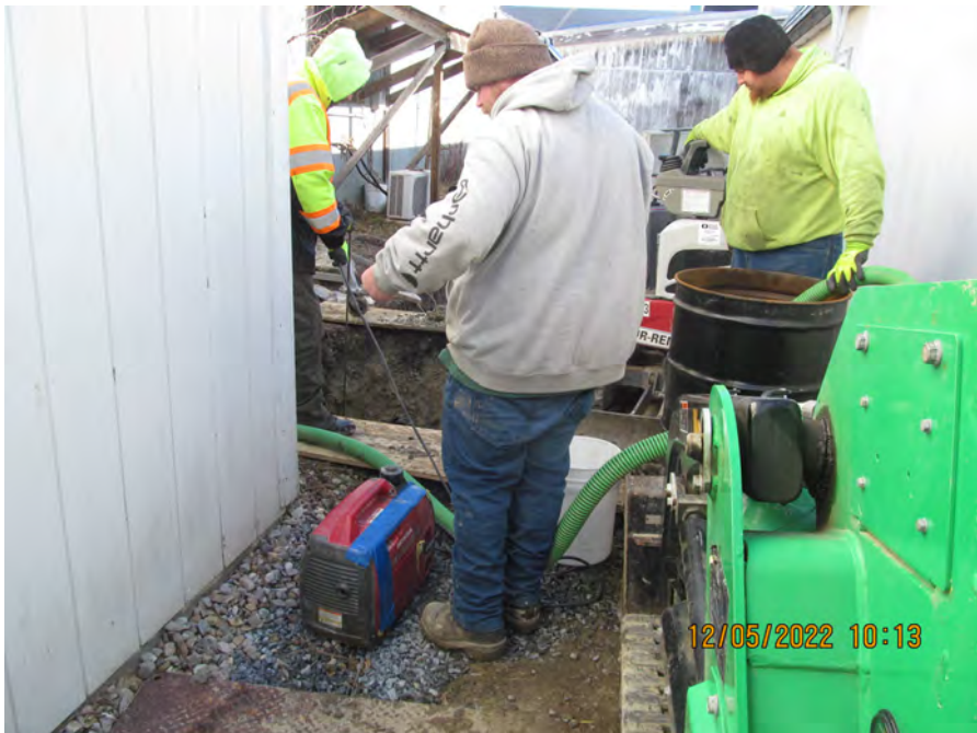
pumpout CB02 location to check depth
