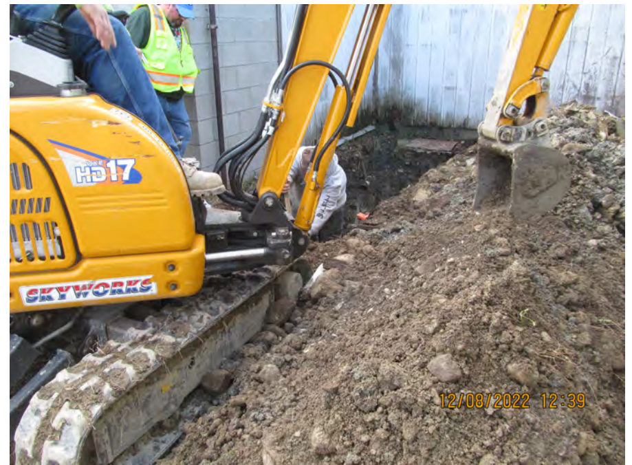
hand locating sewer pipe crossing cmp
