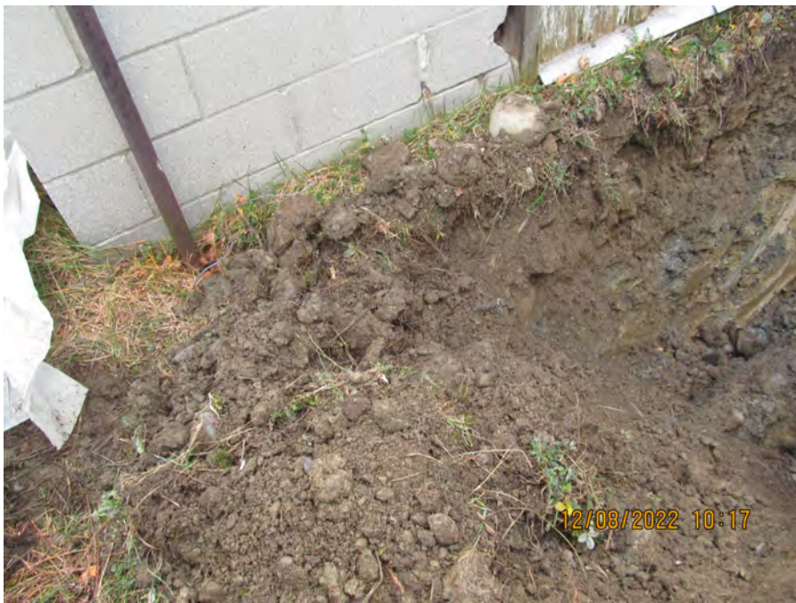
abandoned wires at CB08 location
