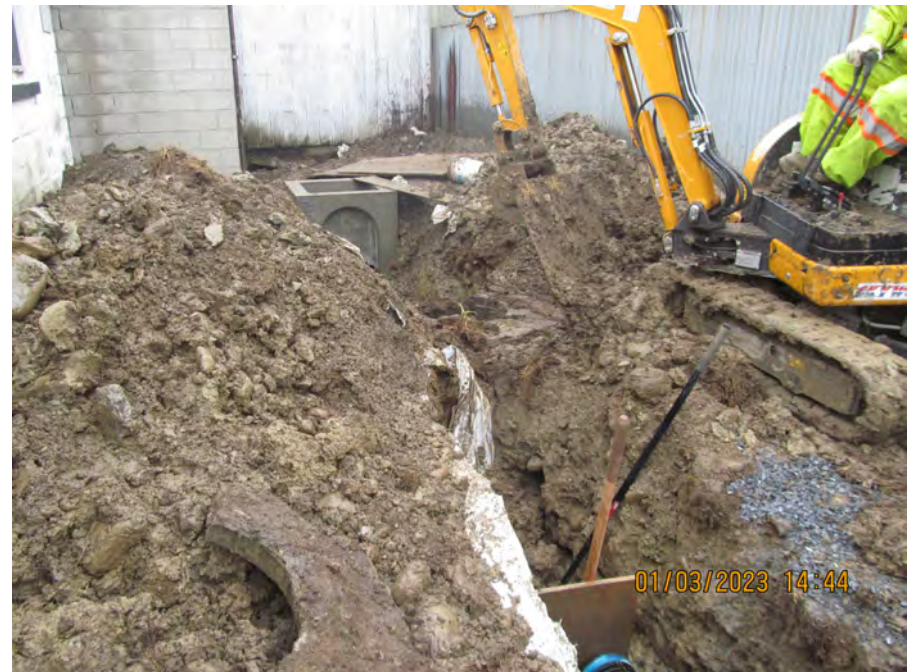
exist structure removal
