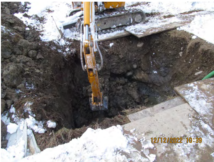
cleaning hole for cb7
