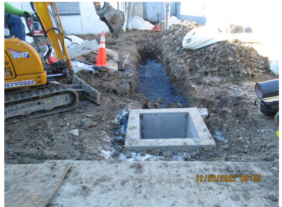
backfill stone
