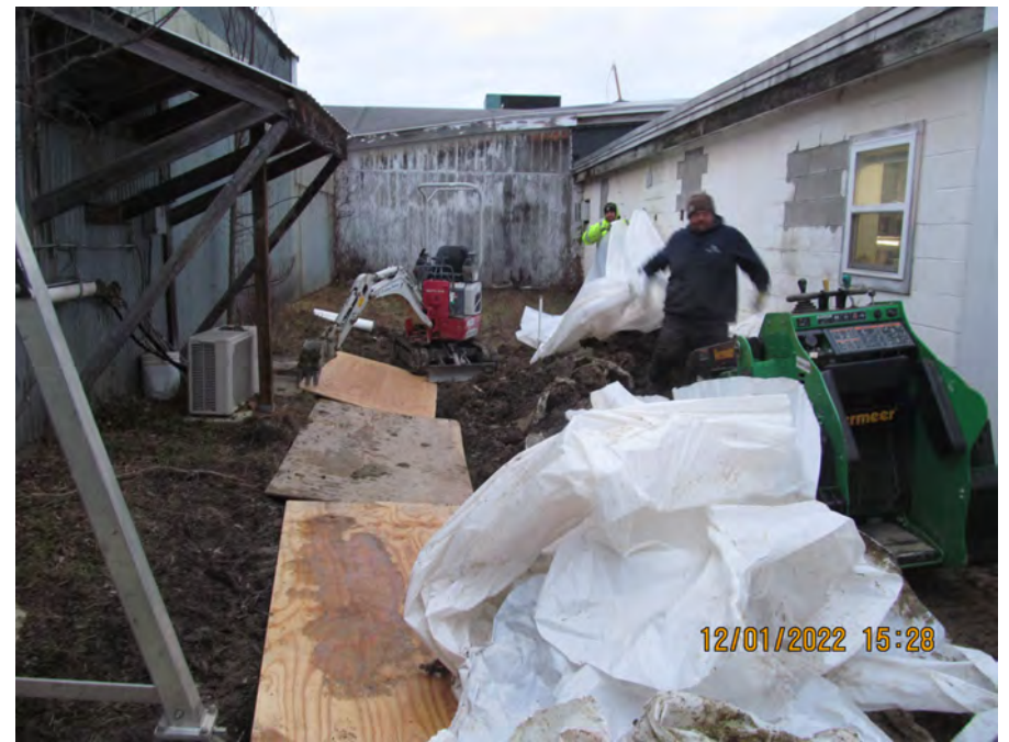
covering trench and pile
