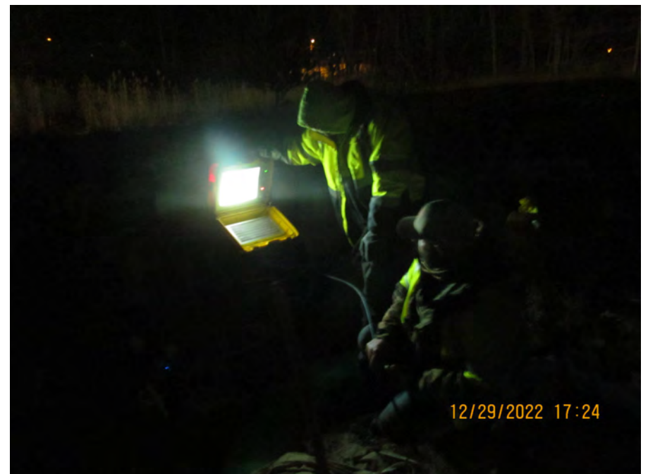
camera survey installed line
