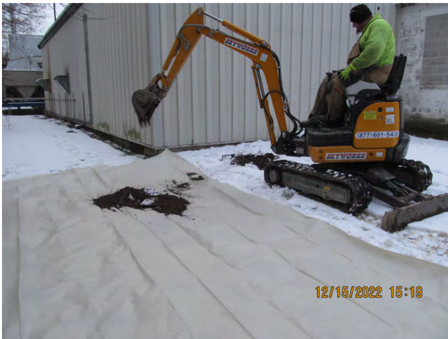
exc liner pit at bldg
