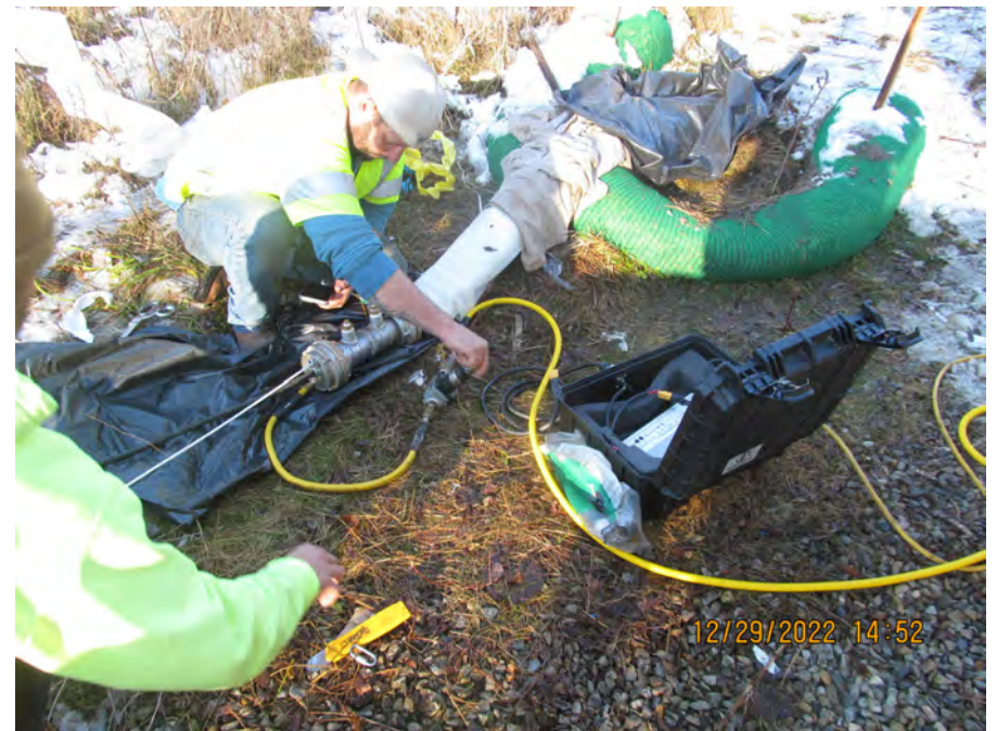
inflate liner to start curing
