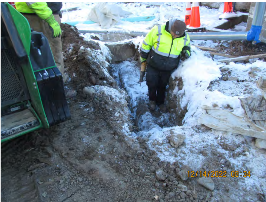
preparing to cut 12 inch cmp
