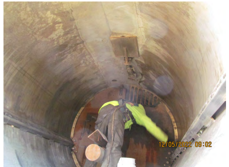
wash down vactruck decon
