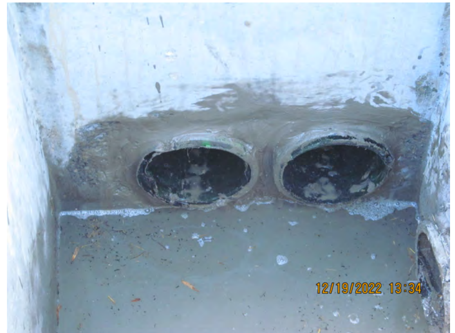
grouted outlet pipes cb7
