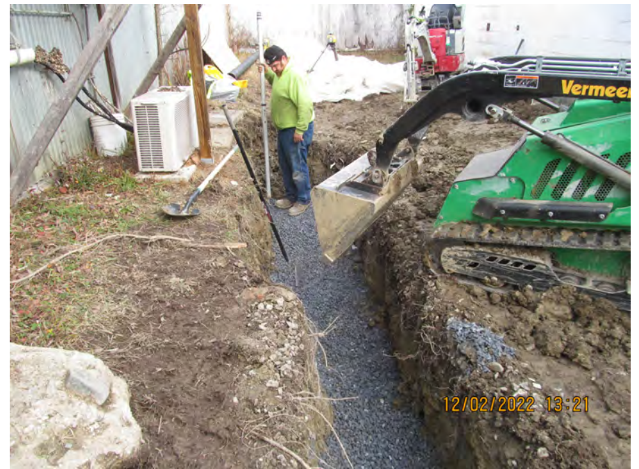
completing stone grade
