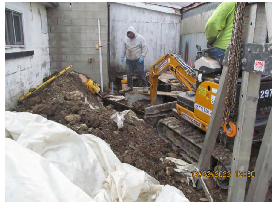
exc for cb8 inlet pipe coring
