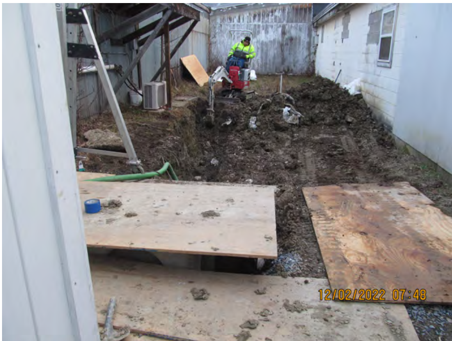
setting base grades
