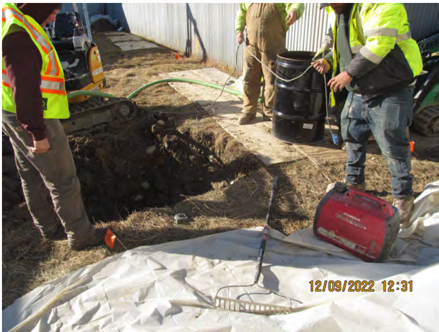
pump out water
