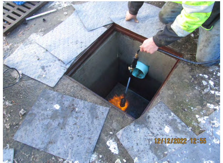
dry walls to check for leaks
