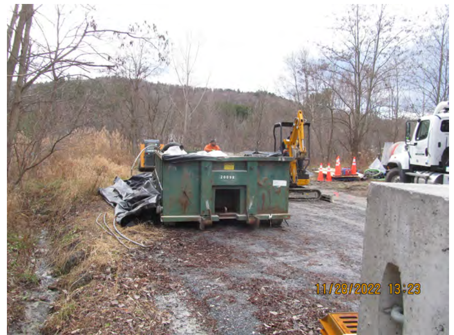
making room for vac truck in rolloff
