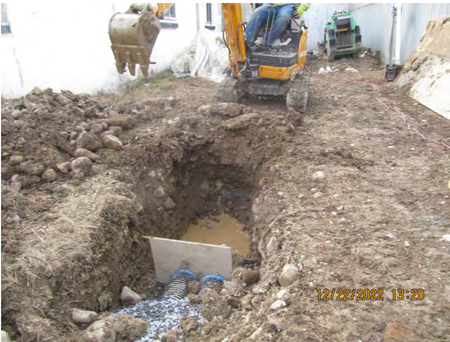
exc for twin 8 pipes from cb7
