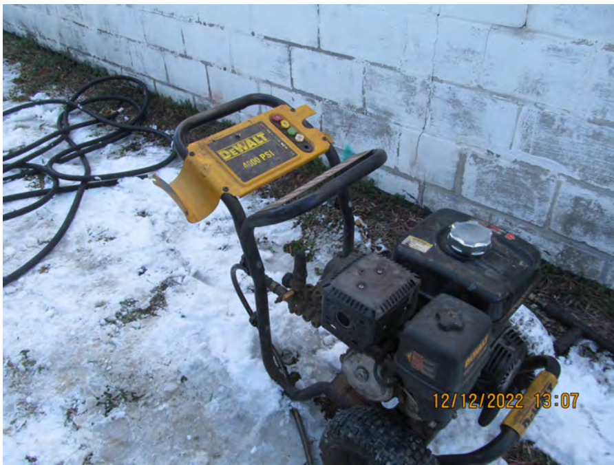
powerwash walls before application
