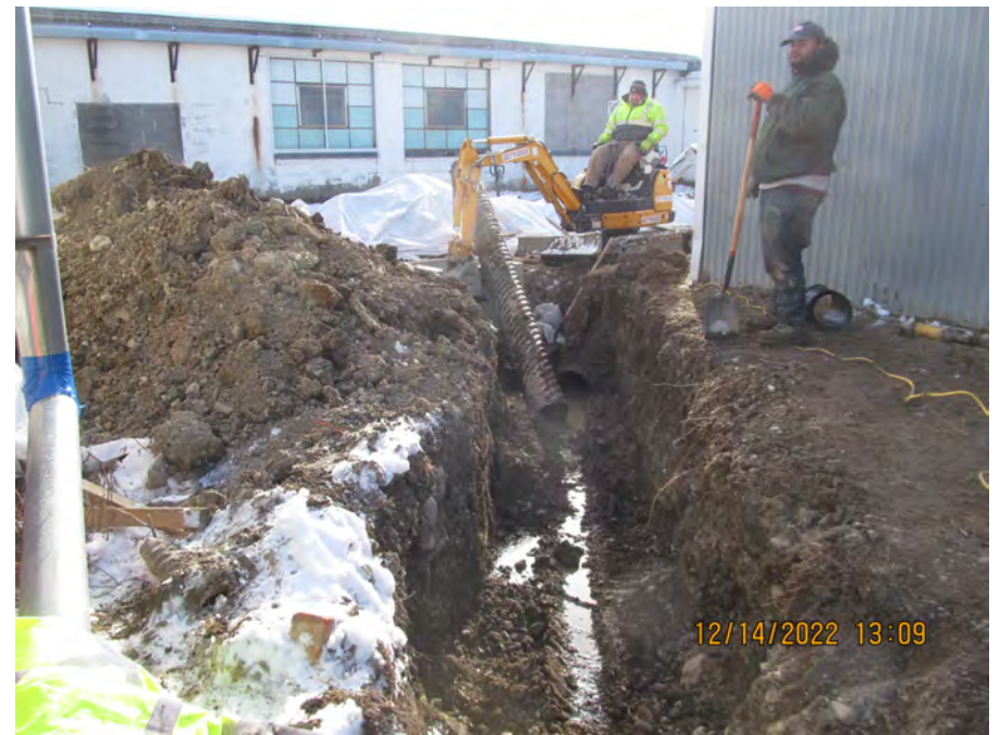
remove 12 inch cmp section
