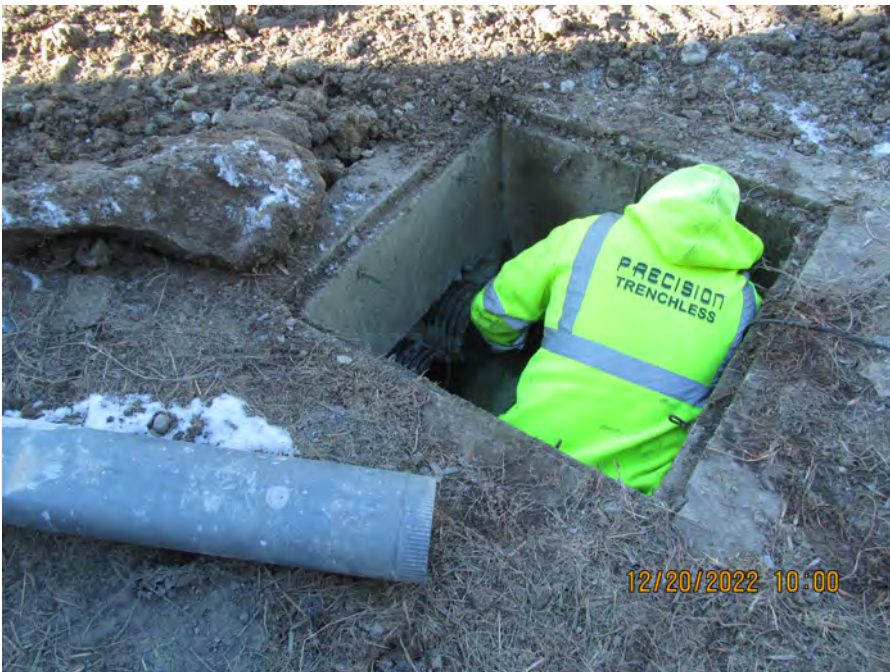
core leak hole to seal
