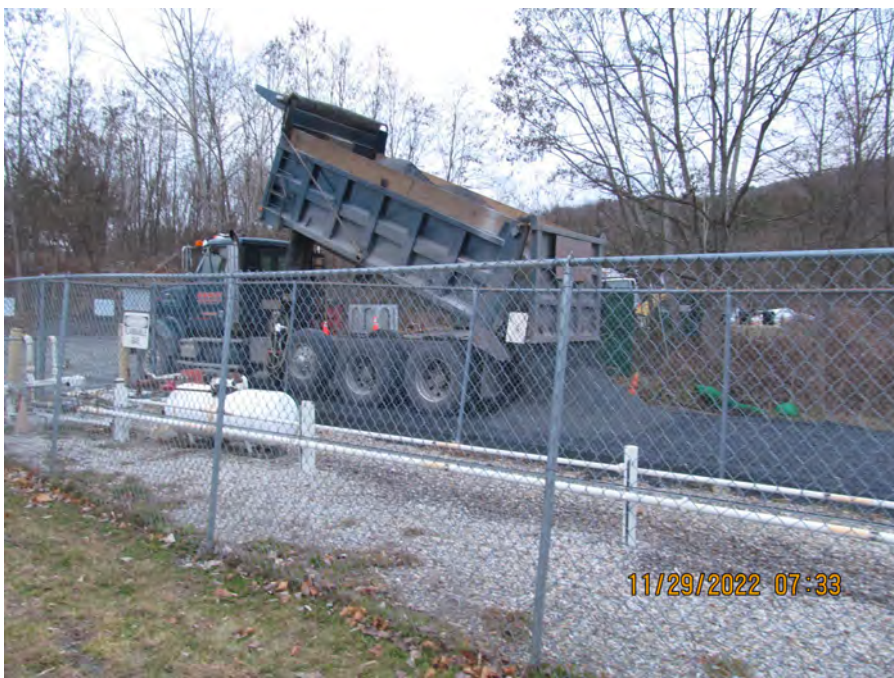
stone for culvert cover
