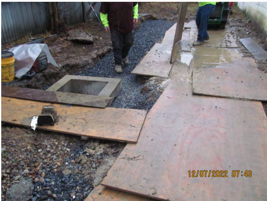
remove trench protection
