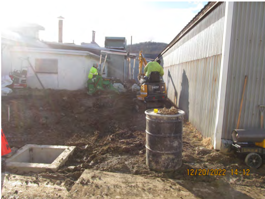
cleanup along building
