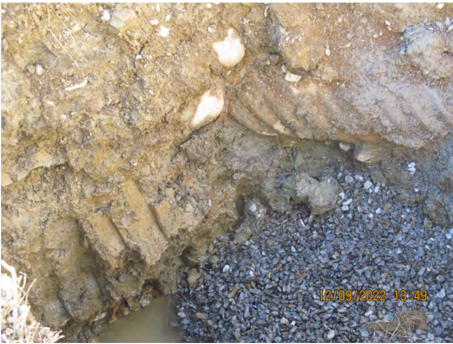
pipe cut back from exc
