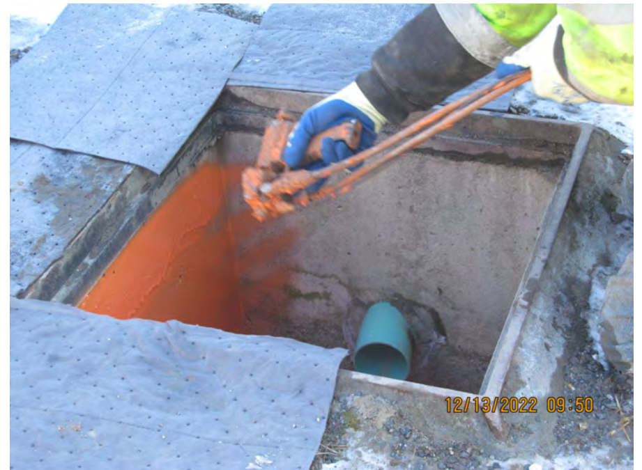
liner first coat
