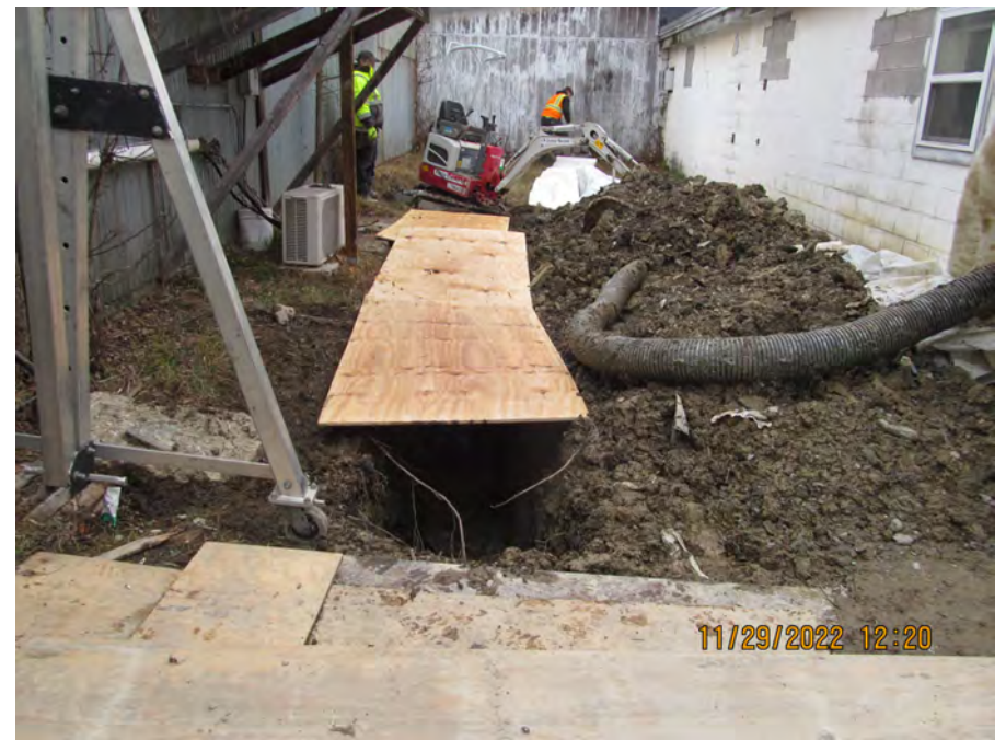
plugged hole and covered trench
