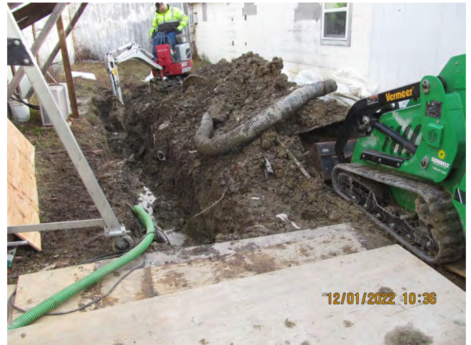
excavator helping with loadout of spoils
