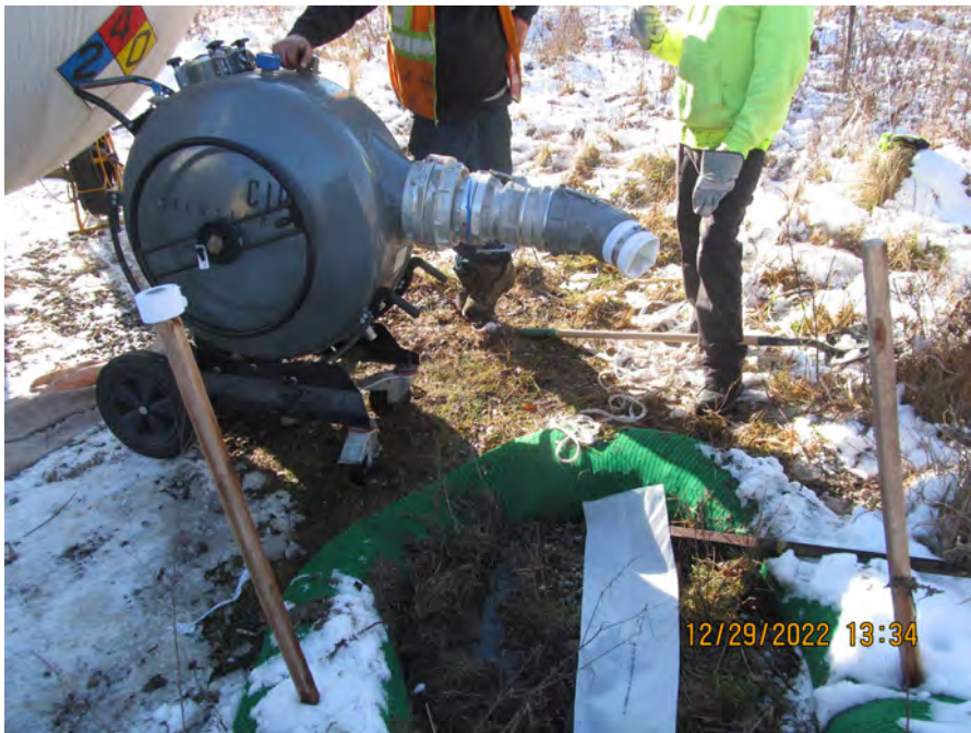
prep for liner install
