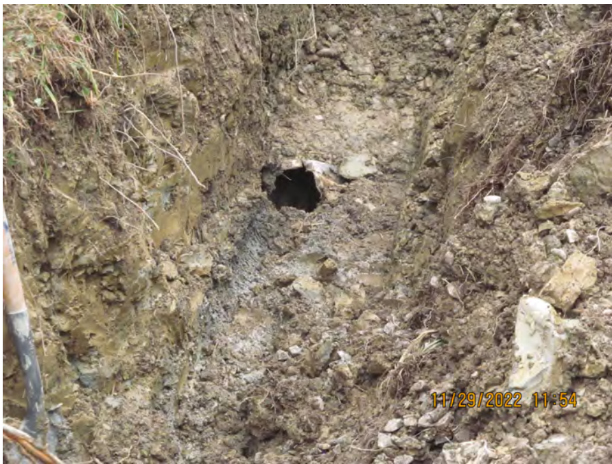
existing 6 inch line removed
