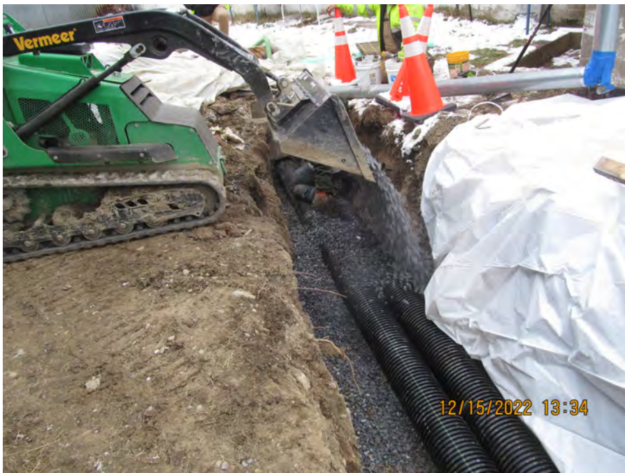
start stone backfill cu13
