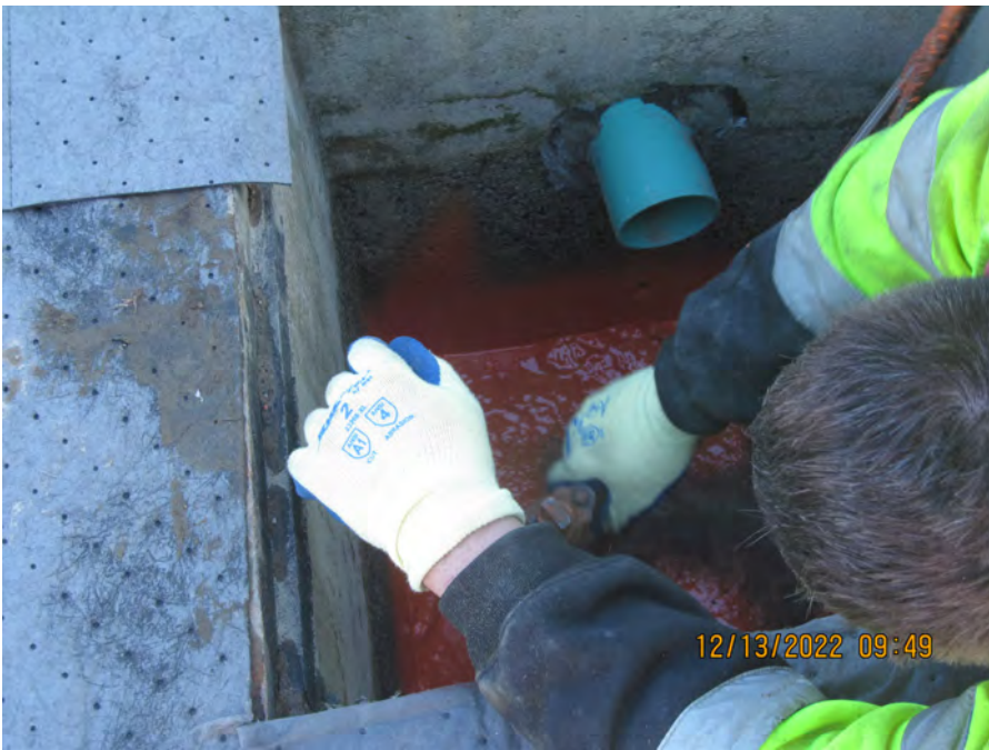
start liner first coat
