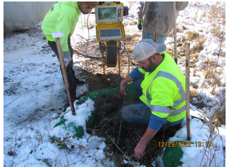
camera line survey for clean check
