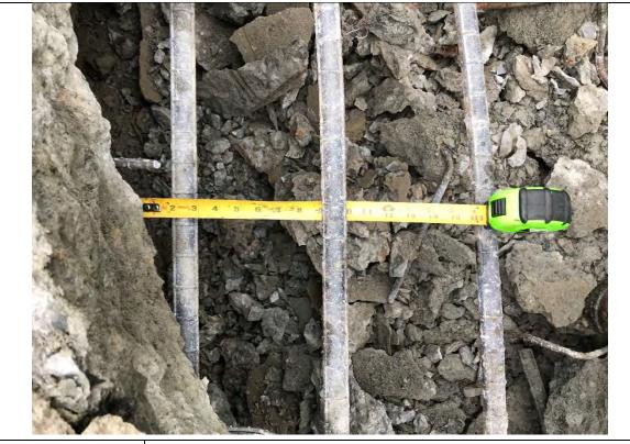
Photograph: 12 Steel rebar 6" apart maintain culvert roof structural integrity.
