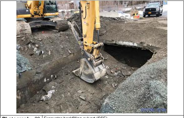
Photograph: 29 Excavator backfilling culvert (SSE).
