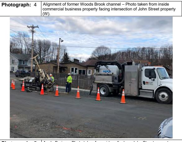
**Photograph:** 5 Angle Boring – Photo taken from sidewalk along John Street property as crew prepare angle soil boring beneath culvert (NNW).
