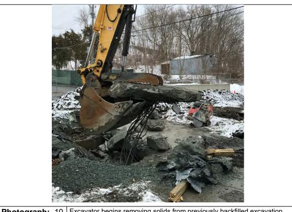
Photograph: 10 Excavator begins removing solids from previously backfilled excavation (SSE).
