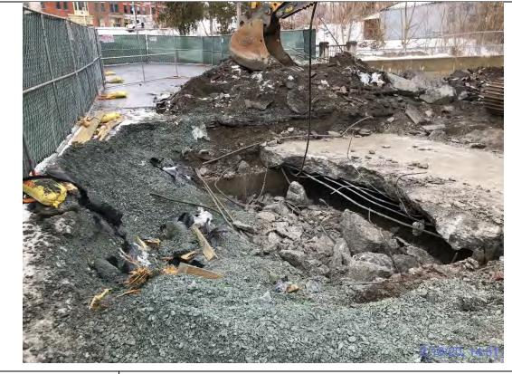
Photograph: 11 Debris being removed from previously backfilled excavation (SSE).
