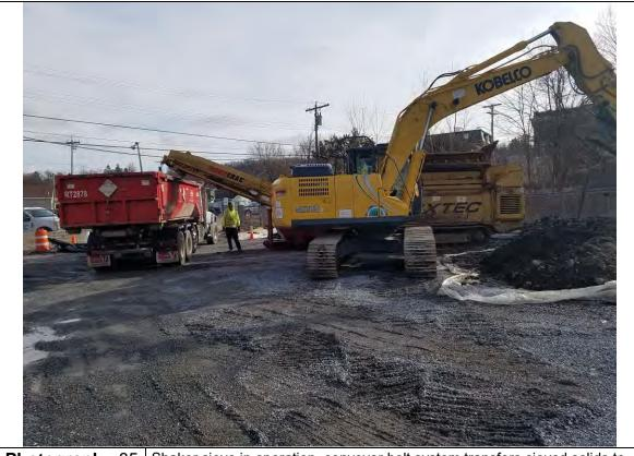
**Photograph:** 35 Shaker sieve in operation, conveyor belt system transfers sieved solids to roll-off container on truck (E).
