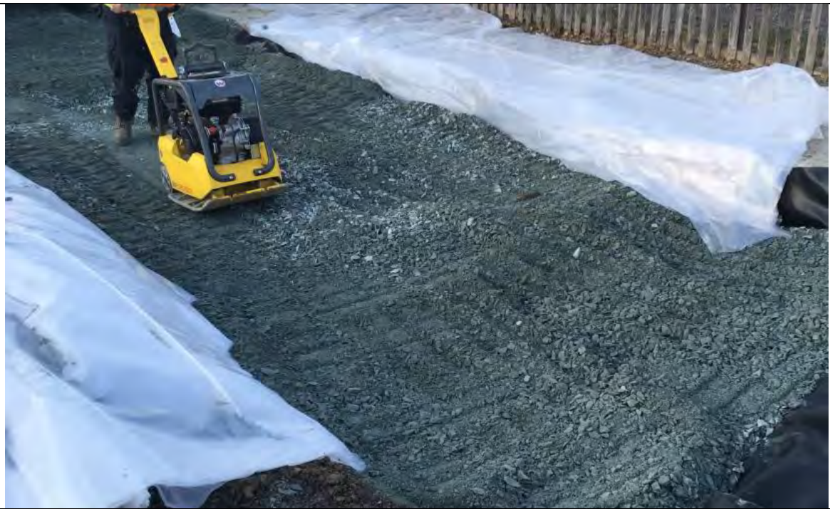
Photograph: 11 | Box Culvert – View facing northwest depicting infiltration liner fill compaction
