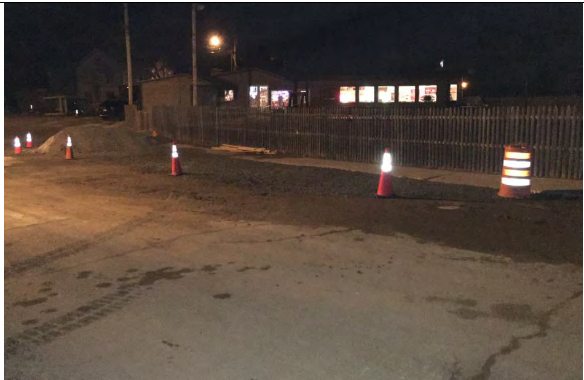
Photograph: 13 Box Culvert – View facing northwest depicting traffic cone protection, completed culvert fill area, and surplus crusher run stockpile.
