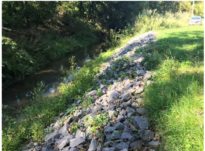
3. Vegetation is beginning to establish at the Seep 1 revetment.
