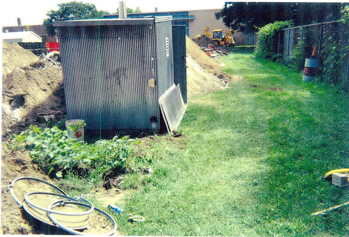
Photo 3: View of Ethylene Glycol Shed looking West
