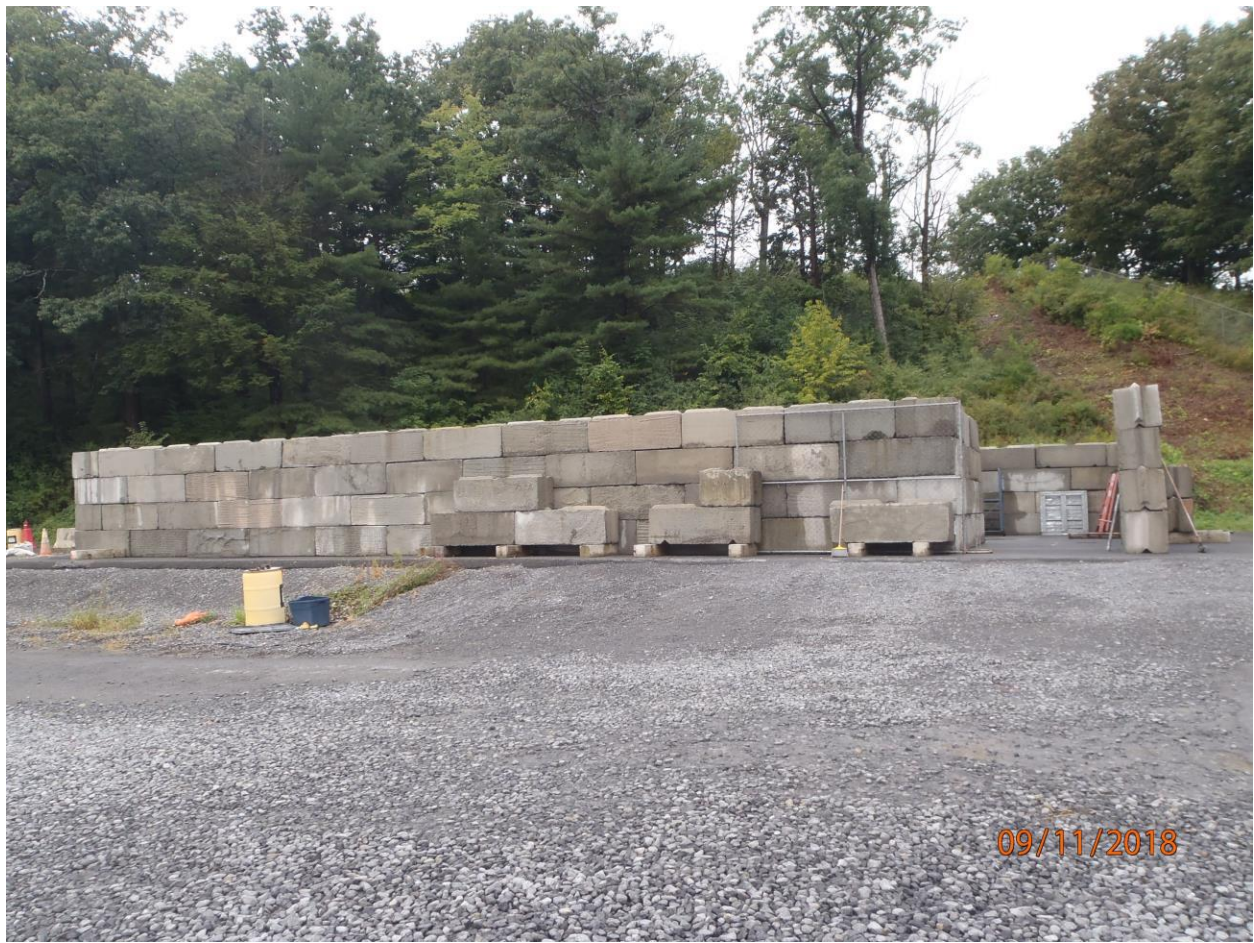
SWMU-085 SPRU Mixed Waste Storage Area (TAA-003), view looking South
