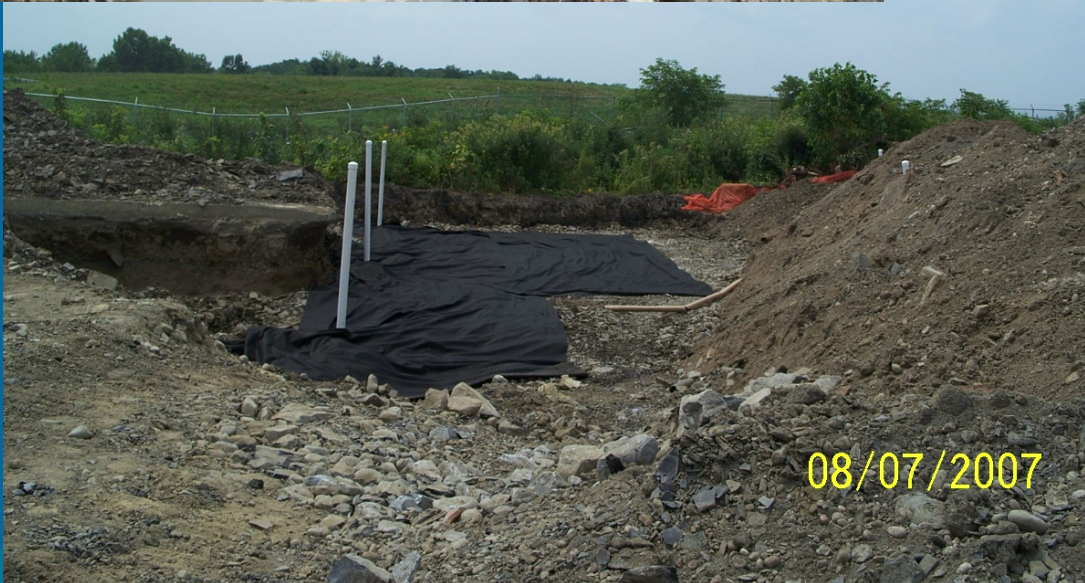
Horizontal well placed and covered with rock and filter fabric
