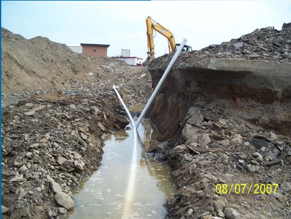
Length of horizontal well being placed
