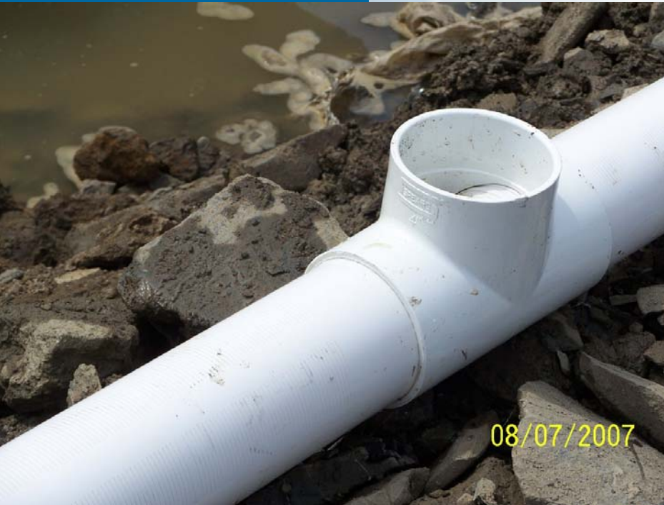
Well screen and Tee connection to riser (not shown)
