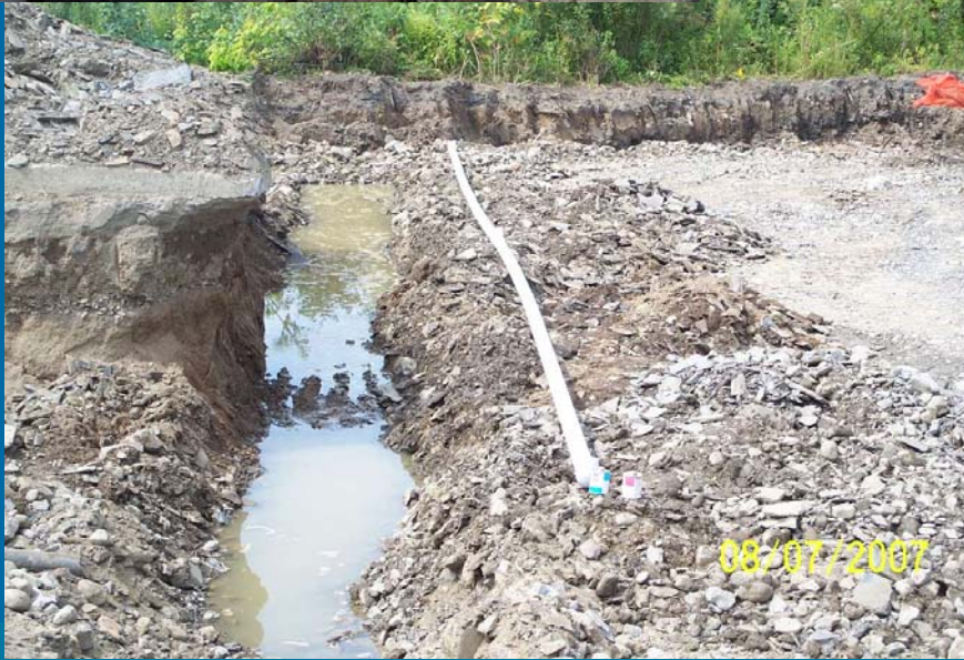
Length of horizontal well ready for placement
