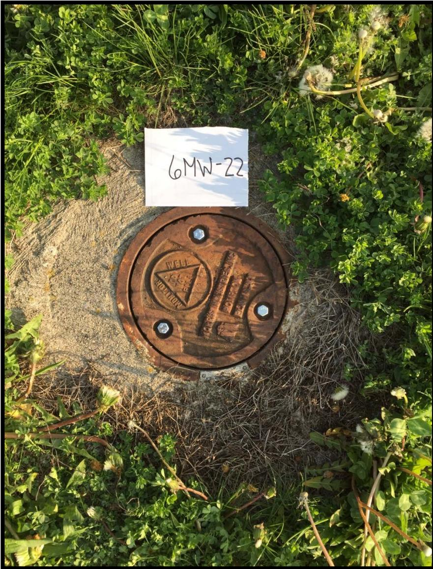
6MW-22 with replaced bolts (typical)
