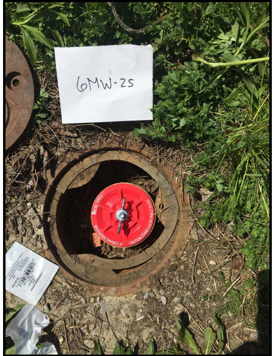
6MW-25 with new pipe plug
