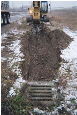
Excavating dry well DW-1: catch basin is in foreground.
