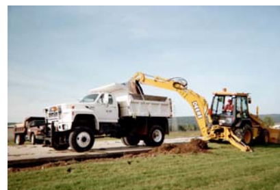
Loading excavated soils prior to disposal at Colonie Town Landfill.
