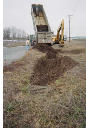
Backfilling dry well DW-1 excavation with native soil.
