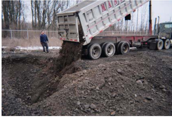
Backfilling DW-2 dry well excavation.
