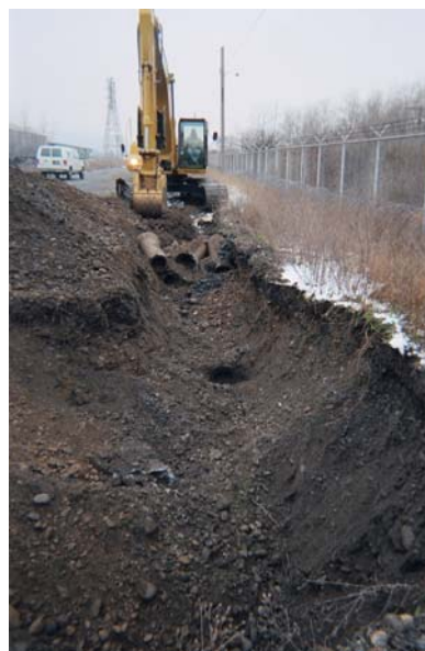
Excavating conduit leading to DW-2. This catch basin was also excavated and removed.
