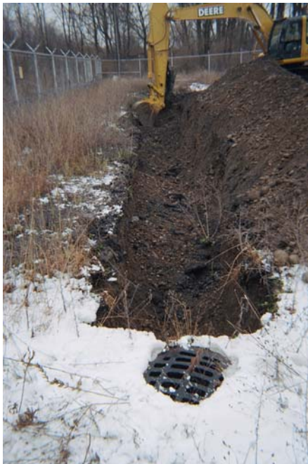
Excavating dry well DW-2.
