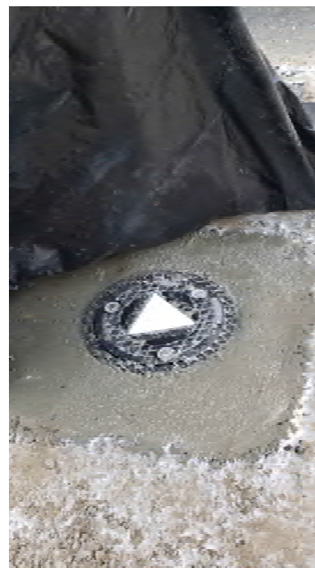
MW-8 After Repair
