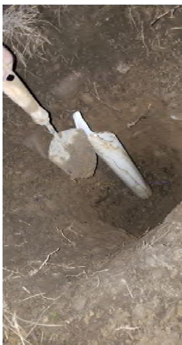
MW-22R Crack in PVC
