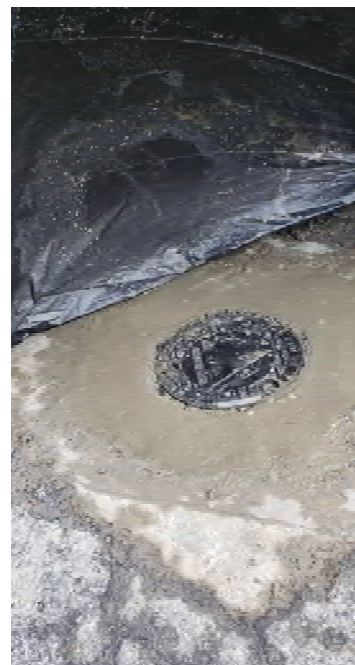
Injection Well After Repair
