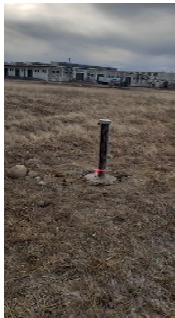
GEP-1 After Repair
