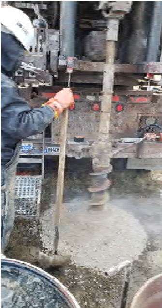
MW-12R Drill cuttings
