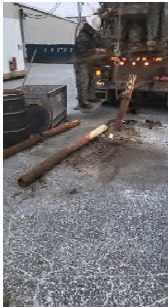
MW-8 During Repair
