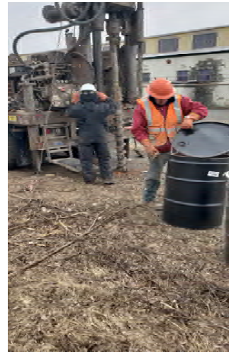
Drilling New MW-B-1R Location
