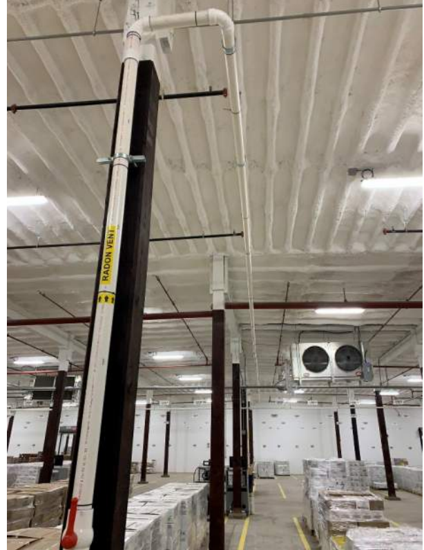
Photograph 4. PVC horizontal piping connecting the extraction point to the moisture discharge point.
