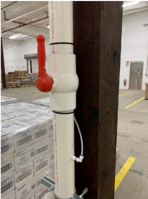
Photograph 3. Ball valve attached to Schedule 40 PVC pipe risers.
