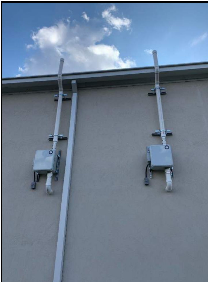
Photograph 9. Two RadonAWay HS5500 fan mounts on exterior wall of Building 403.
