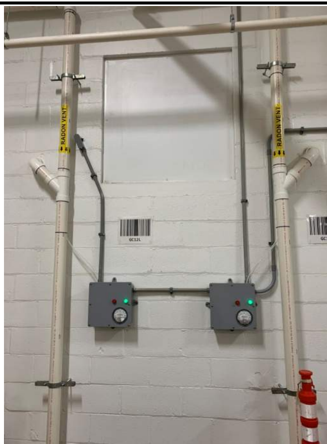
Photograph 6. Moisture discharge points and monitoring panels for two sub-systems.
