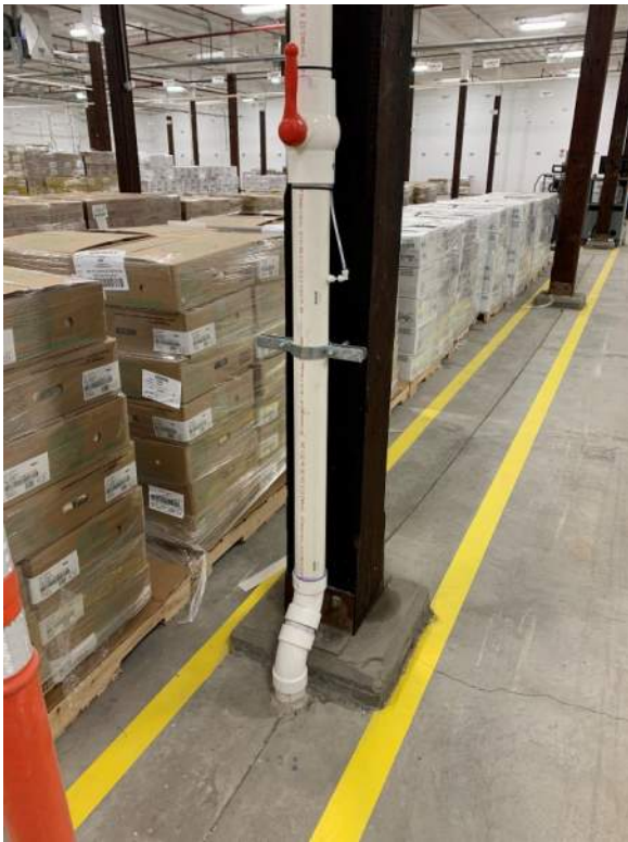
Photograph 1. One vapor extraction point at column footing.
