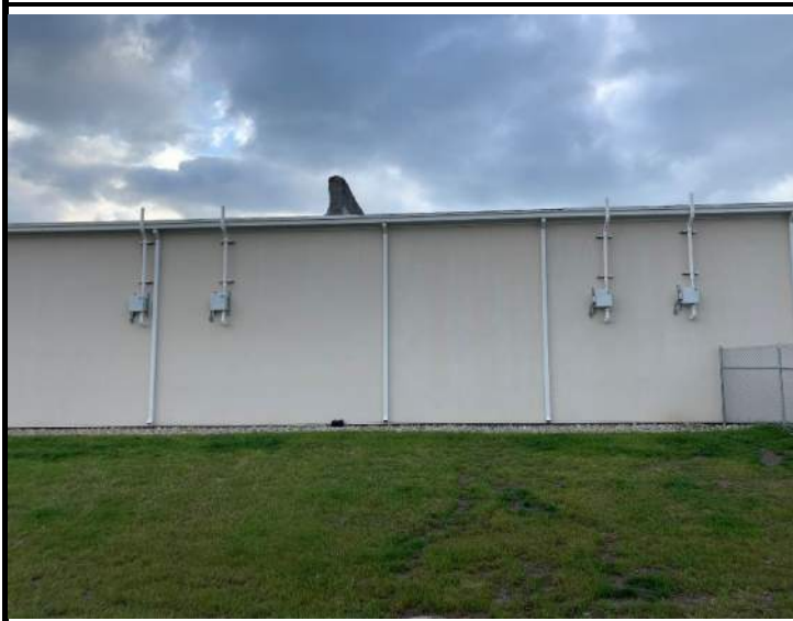
Photograph 7. RadonAway HS5500 fan mounts for Sub-Systems 1, 2, 4, and 5 on the exterior wall of Building 403 (north).
