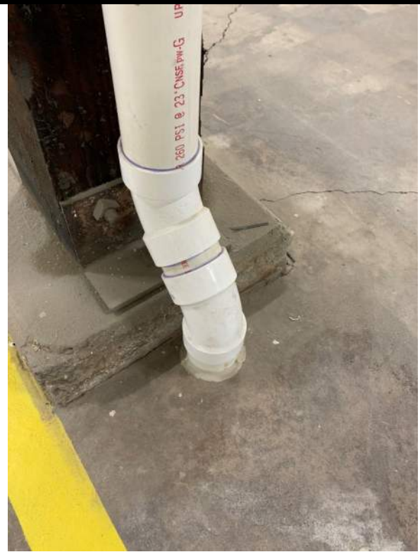
Photograph 2. One vapor extraction point at column footing.
