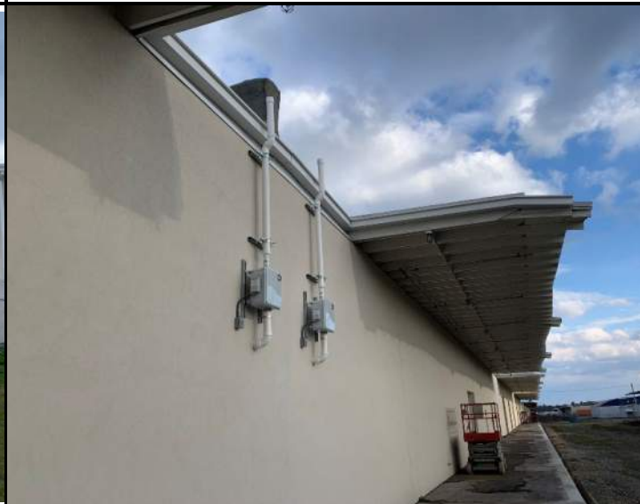
Photograph 8. RadonAway fan mounts extending above the roofline of Building 403 (south side).
