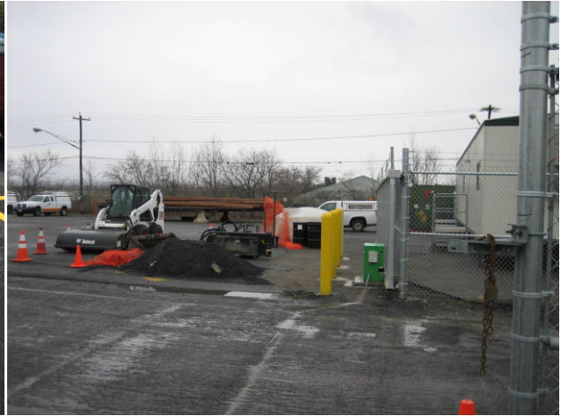
Relocated Main Security Gate 12/1-5/10
