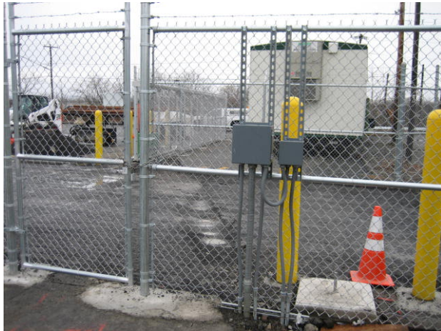
Relocated Main Security Gate 12/1-5/10
