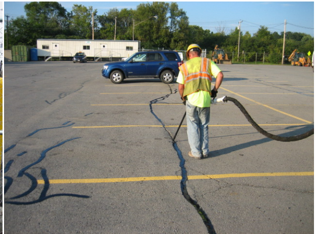
Asphalt Cap Repair on 9/12/11
