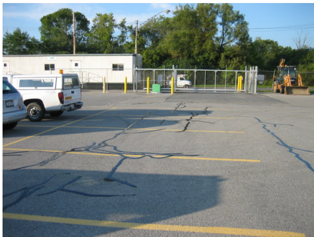
Asphalt Cap Repair on 9/12/11
