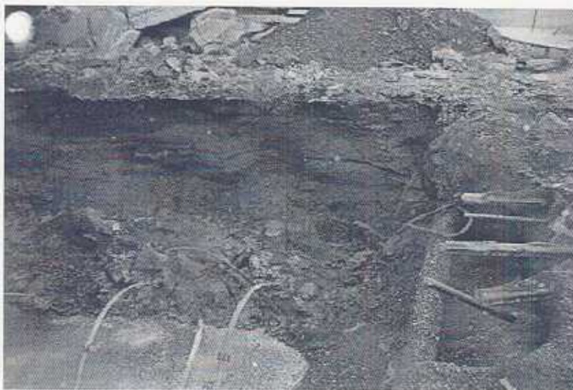
Photograph 4: View to Northeast along Southeast Side of Excavation. Note abandoned cast iron pipe, in right side of photograph, oriented northeast to southwest. Pipe is possibly related to former MGP operation.
