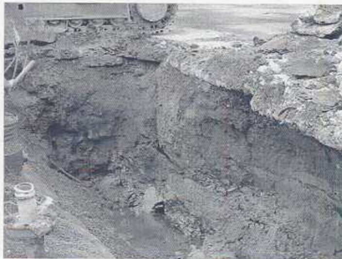
Photograph 2: View to North-Northwest. UST in place with vertical pipes visible. Encountered stained soils and soils with iridescent sheen in north-northwest corner of excavation. Groundwater visible to right of UST.
