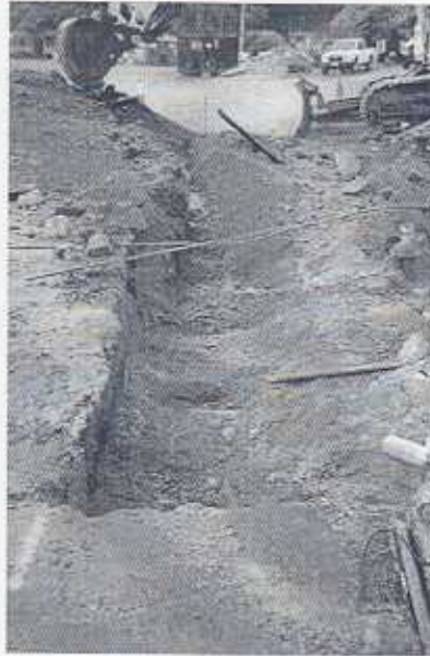
Photograph 1: View to Northwest. UST in place with vertical pipes visible. Abandoned cast iron pipes, possibly related to the former MGP, are visible in foreground (marked with orange paint).
