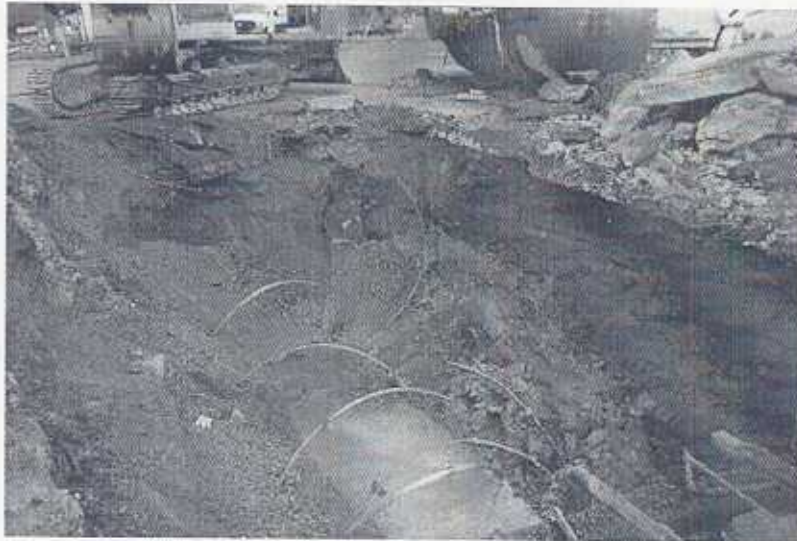
Photograph 3: View to North-Northwest. UST removed (removed tank is visible on upper portion of photograph). Tanks straps are visible within excavation. Stained soil and soil with iridescent sheen visible in north-northwest corner of excavation. Iridescent sheen in water.
