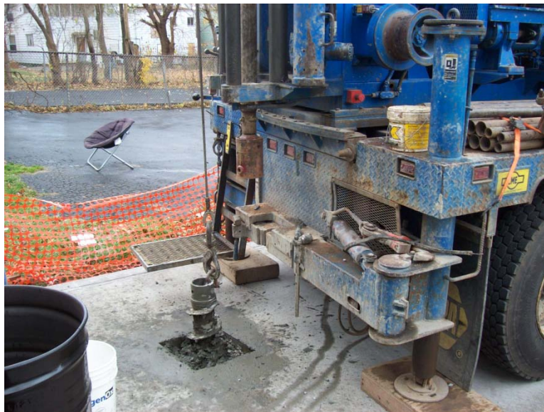
Pulling augers after completion of MW-1R
