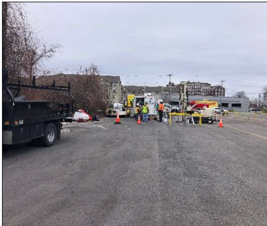
Photo 1: Injection area with Geoprobe and RRS trailer. Looking West.
