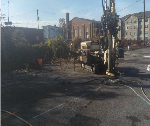
Photo 1: Direct Push Rig and injections ongoing on parking lot. Looking SW.
