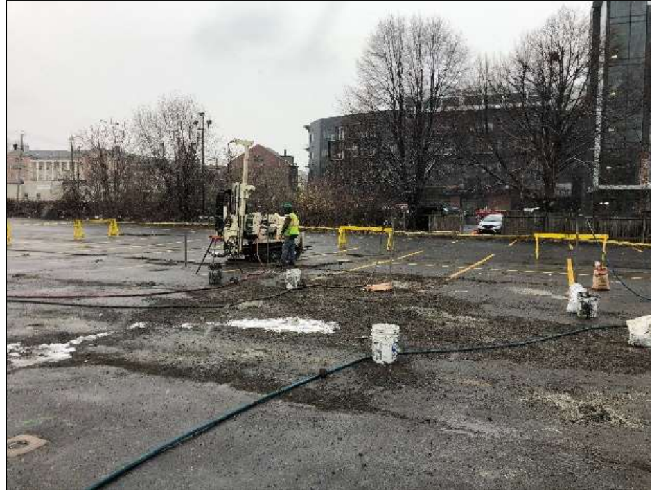
Photo 6: Injections around previous excavation. Looking North.
