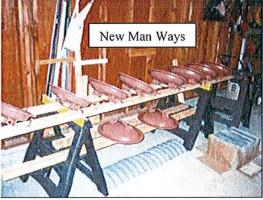
The mixing tank was completely drained and rinsed. The solids were removed. A new valve and flange was installed on the pressure relief valve. The man ways were sanded, primed, painted and re-installed with new gaskets.
