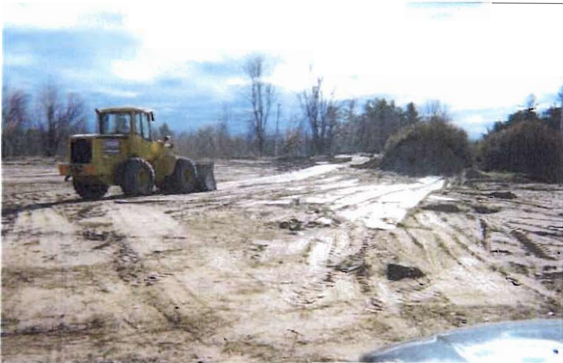
16. Stump Dump. Loader removing material and grading site.
