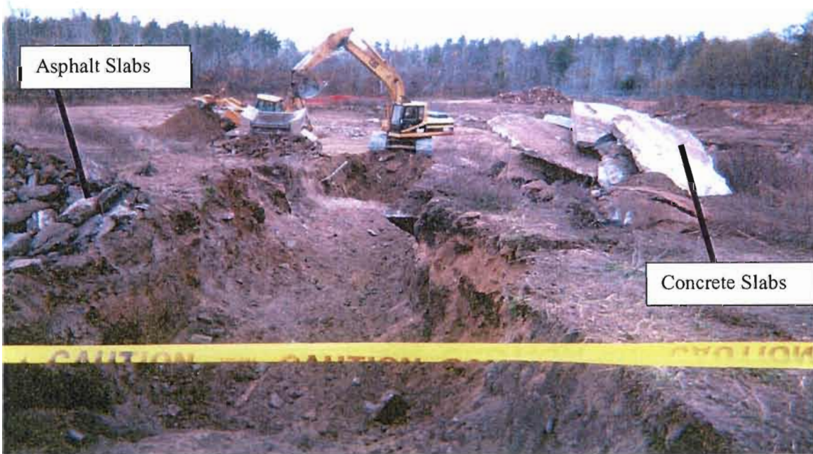
4. C&D Landfill. Excavation of Trench #4
