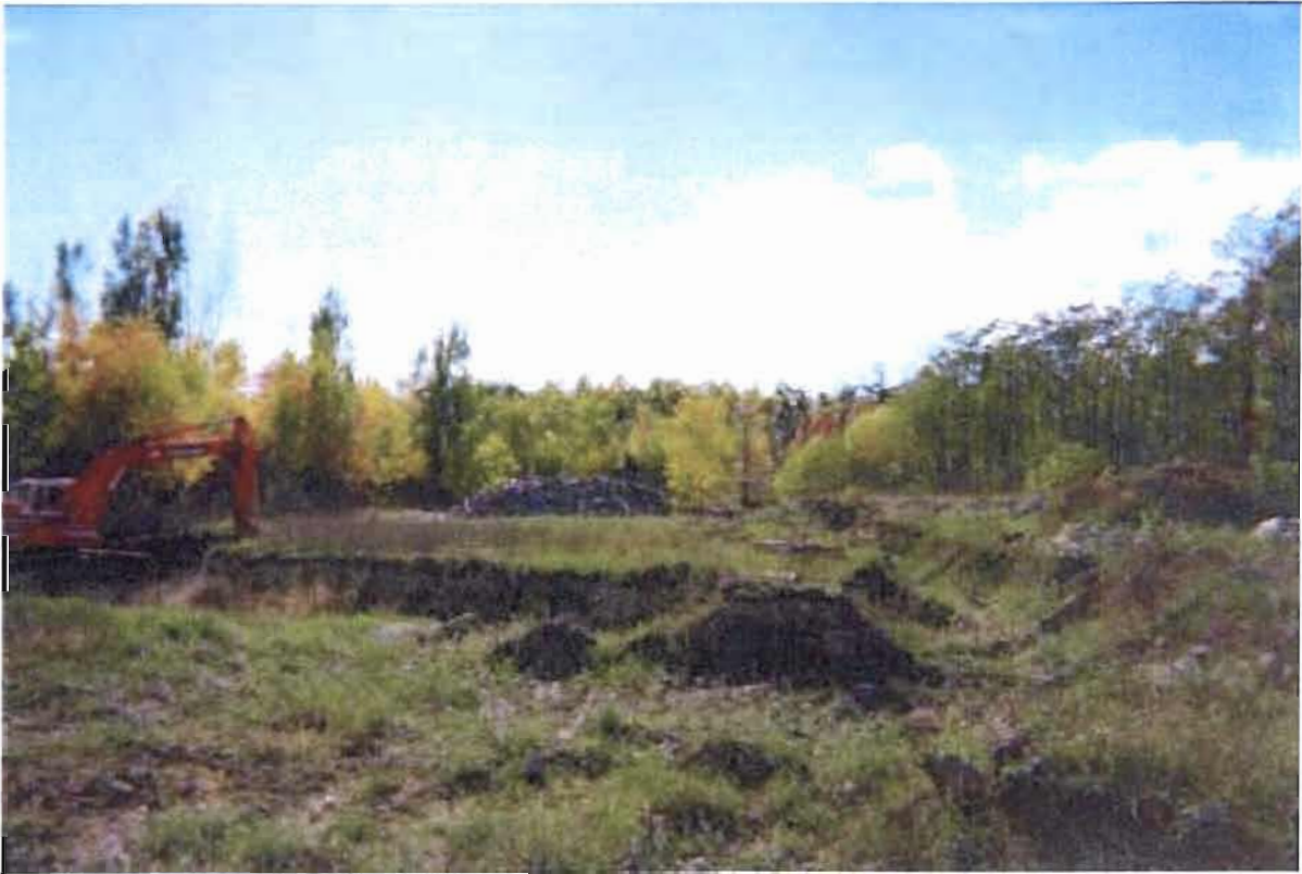
7. C&D Landfill. Excavator turning dirt at western wedge
