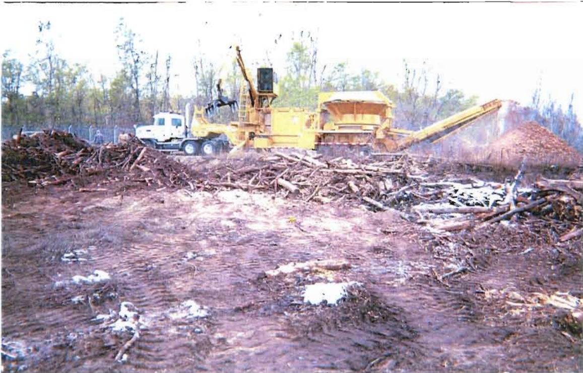
2. C&D Landfill. Tub Grinder chipping wood.
