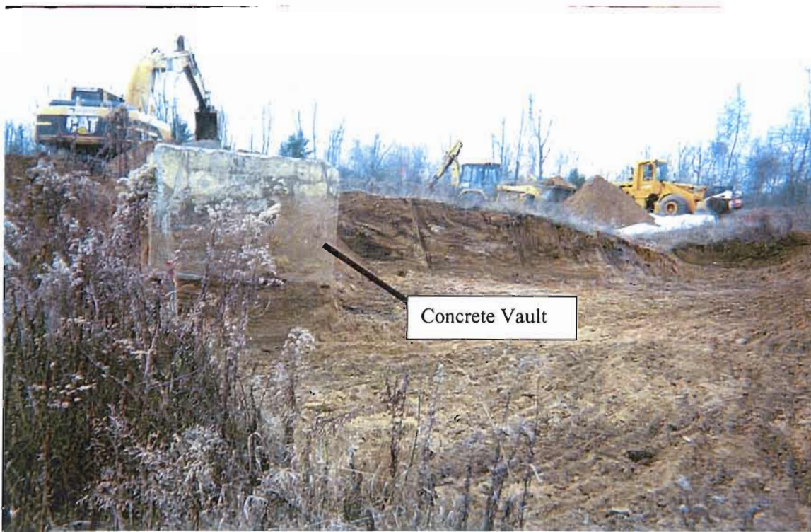
11. Stump Dump. Concrete vault during excavation of Area 1.
