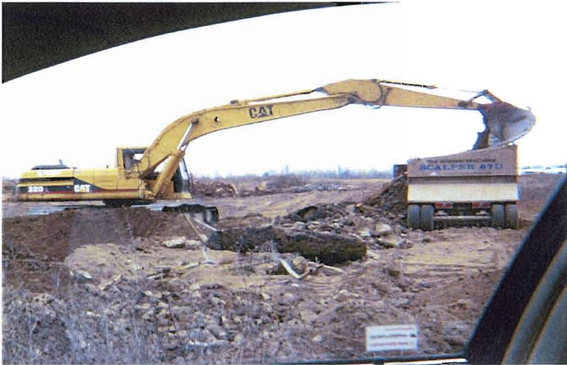
1. C&D Landfill at beginning of excavation.
