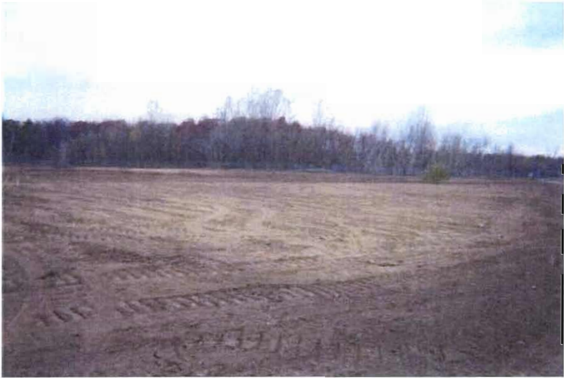
19. C&D Landfill. Site restoration complete.
