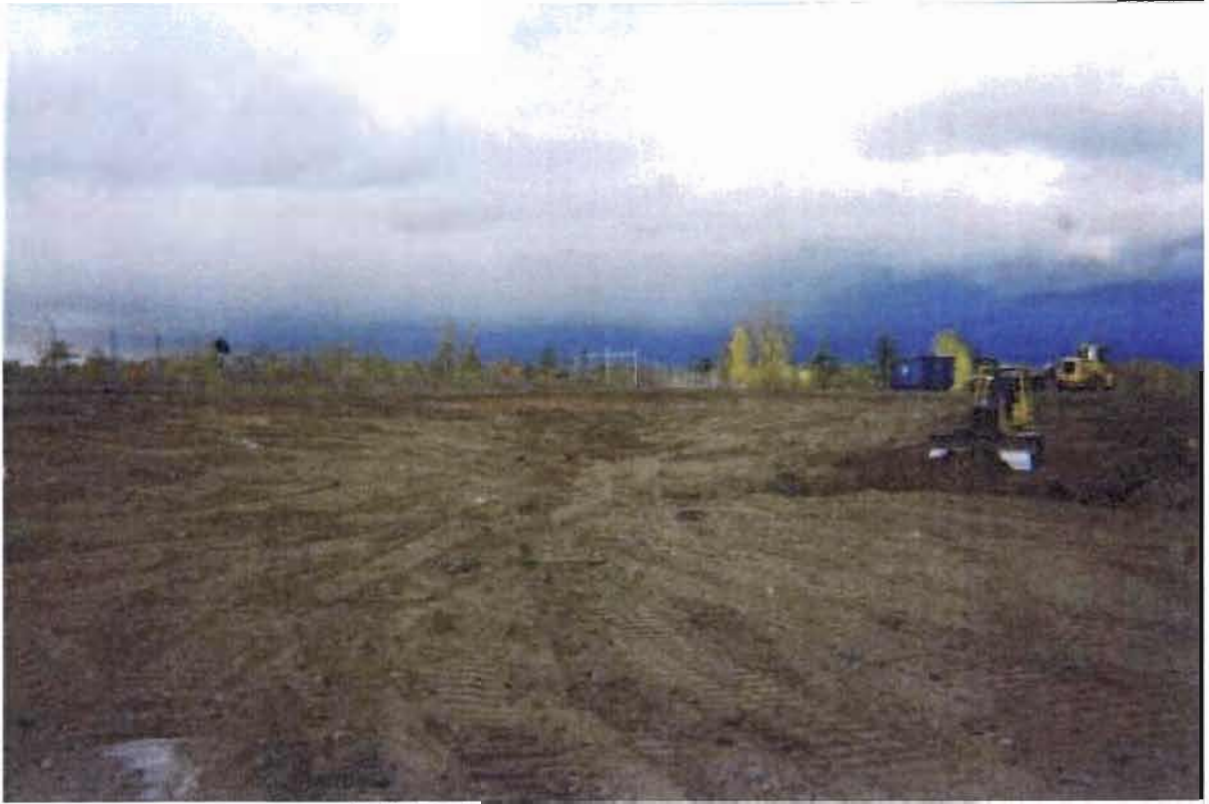
9. C&D Landfill. Bulldozer grading.
