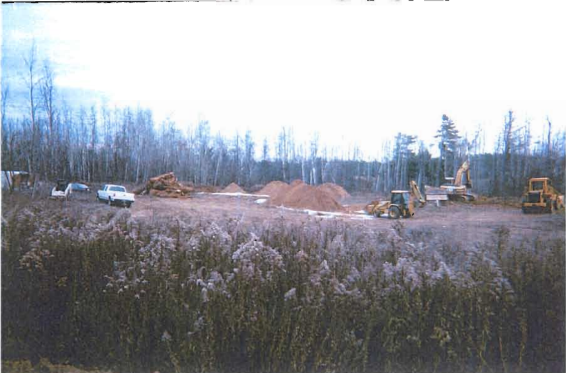
10. Stump Dump. Excavation of Area 1.
