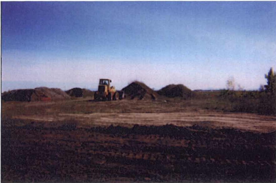
6. C&D Landfill. Loader staging soil piles.
