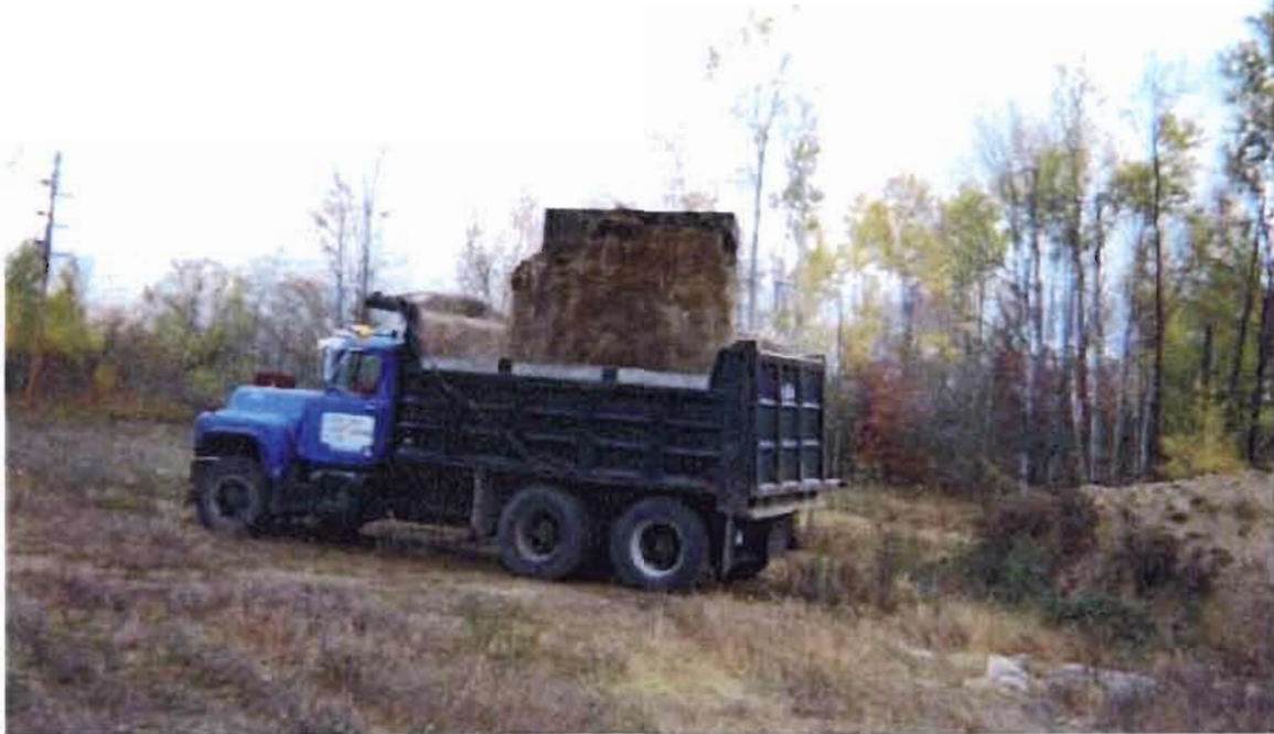
17. Stump Dump. Loader loading soil to dump truck.
