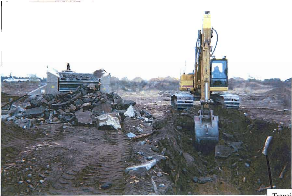
3. C&D Landfill. Field operations at the initial excavation area.
