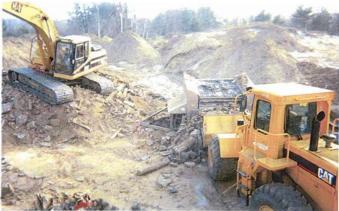
12. Stump Dump. Excavator, Loader, and Shaker Screen during excavation of Area 2.
