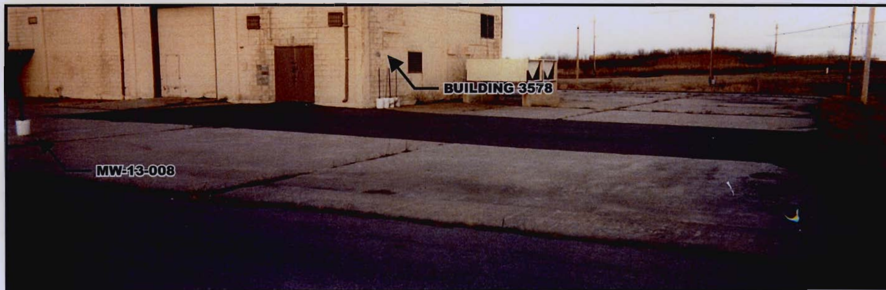
Photo 2: Asphalt pavement patch at completion of OHM UST-3578-A-2 soil removal.
