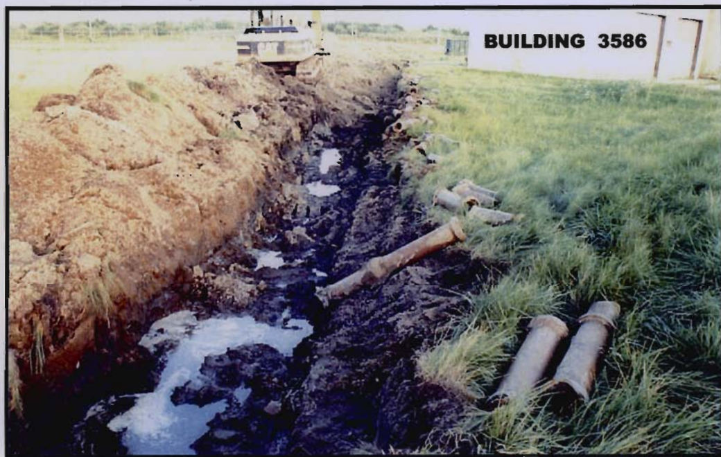
Photo 7: Eastward view from paved access road of vitrified clay pipe removal between septic tank and Building 3580 (September 1996).
