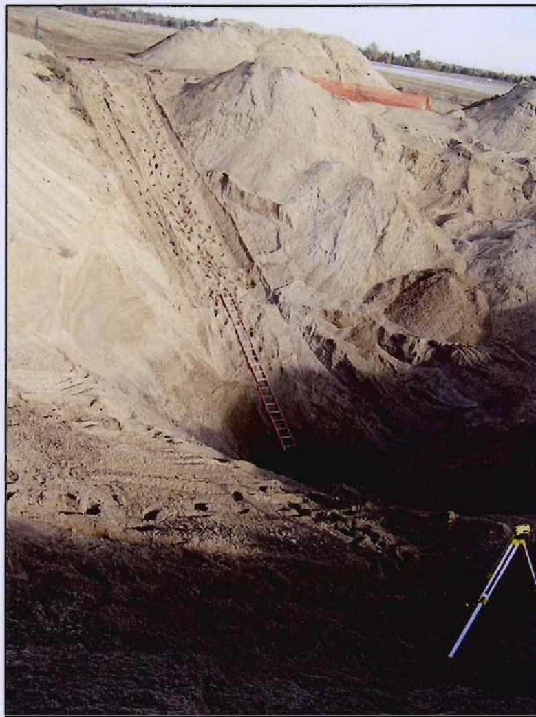
Photo 8 – Extent of excavation at conclusion of third soil removal action. Groundwater is present at the bottom of the excavation at 32.7 ft below ground surface (20 OCT 2004).
