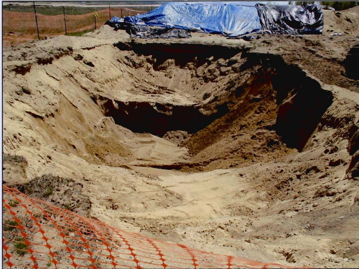
Photo 4 – Extent of excavation at conclusion of second soil removal excavation (12 MAY 2004).
