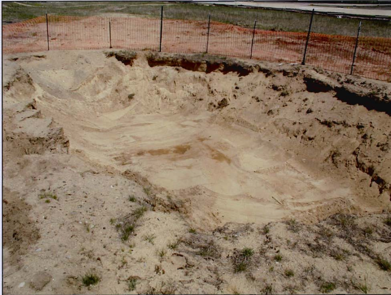
Photo 3 – Stained soil at base of second soil removal excavation (12 MAY 2004).
