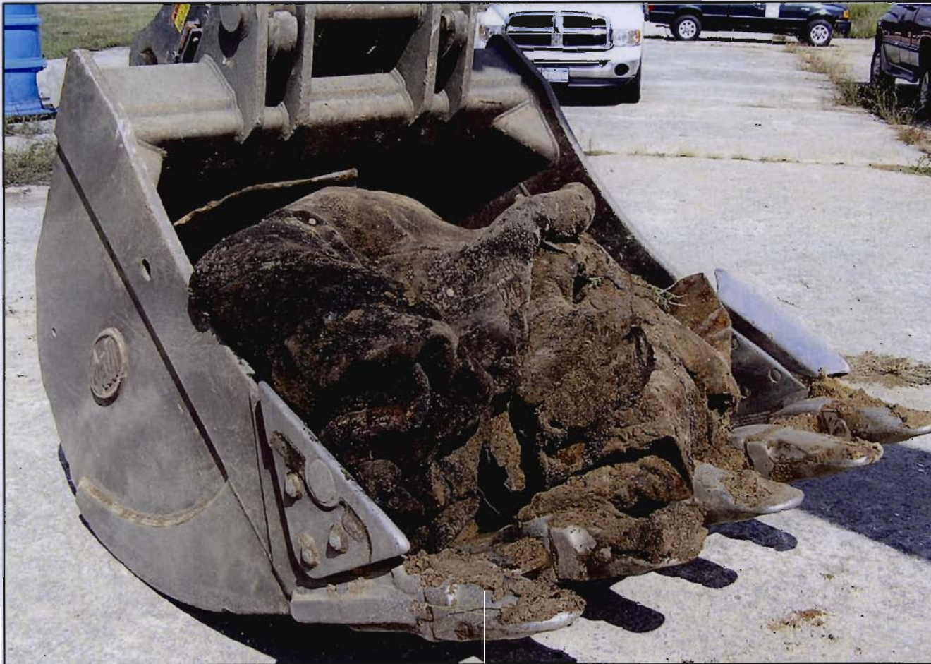
Photo 10 – Examples of tar mats and drum fragments recovered during the second removal action. Note the cohesive nature of the recovered tar mat with adhered soil. (01 SEP 2005).
