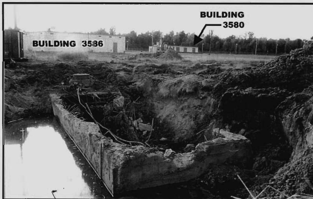
Photo 4: Westward view of excavated 7,500 gallon septic tank and excavation of piping leading from septic tank to Building 3580 (September 1996).
