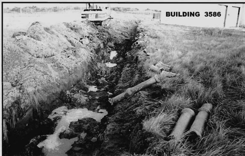
Photo 5: Eastward view from paved access road of vitrified clay pipe removal between septic tank and Building 3580 (September 1996).
