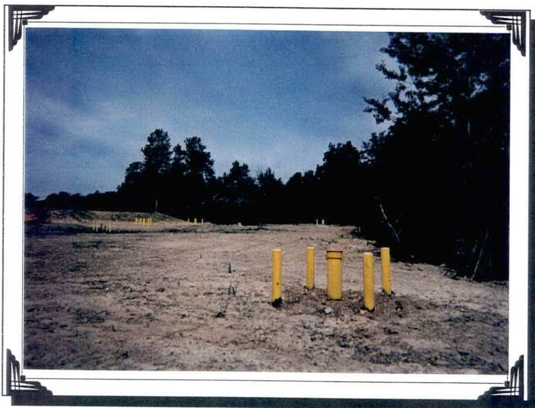
Collection Trench Cleanout (foreground) Leachfield (background, left)
