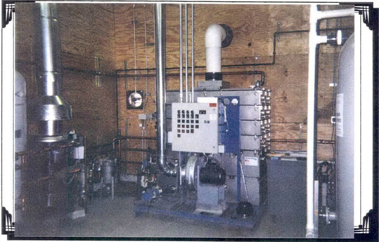
Shallow Tray Air Stripper and Control Panel
