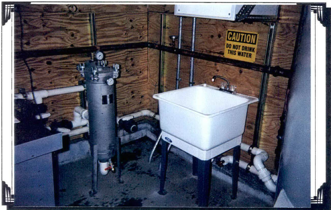
Primary Bag Filter and Wash Sink
