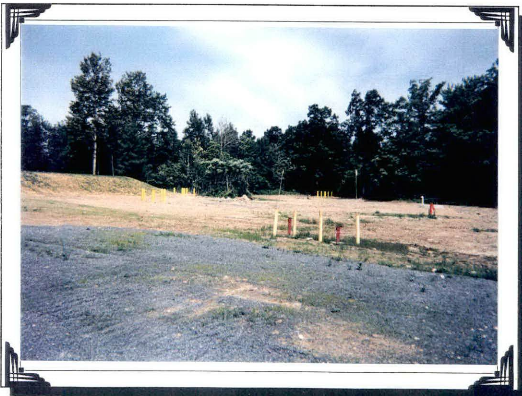
Groundwater Monitoring Wells (foreground) Collection Trench Cleanouts and Leachfield (background, left)
