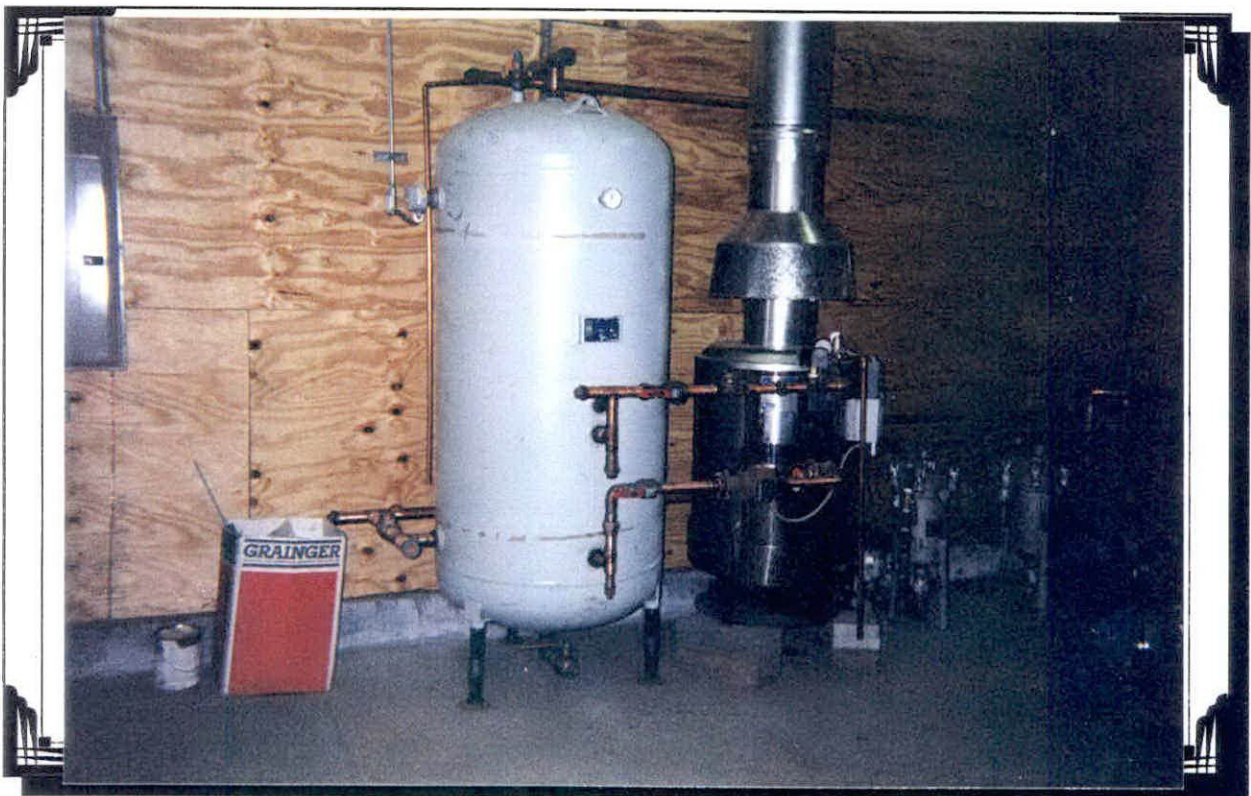
Boiler and Storage Tank
