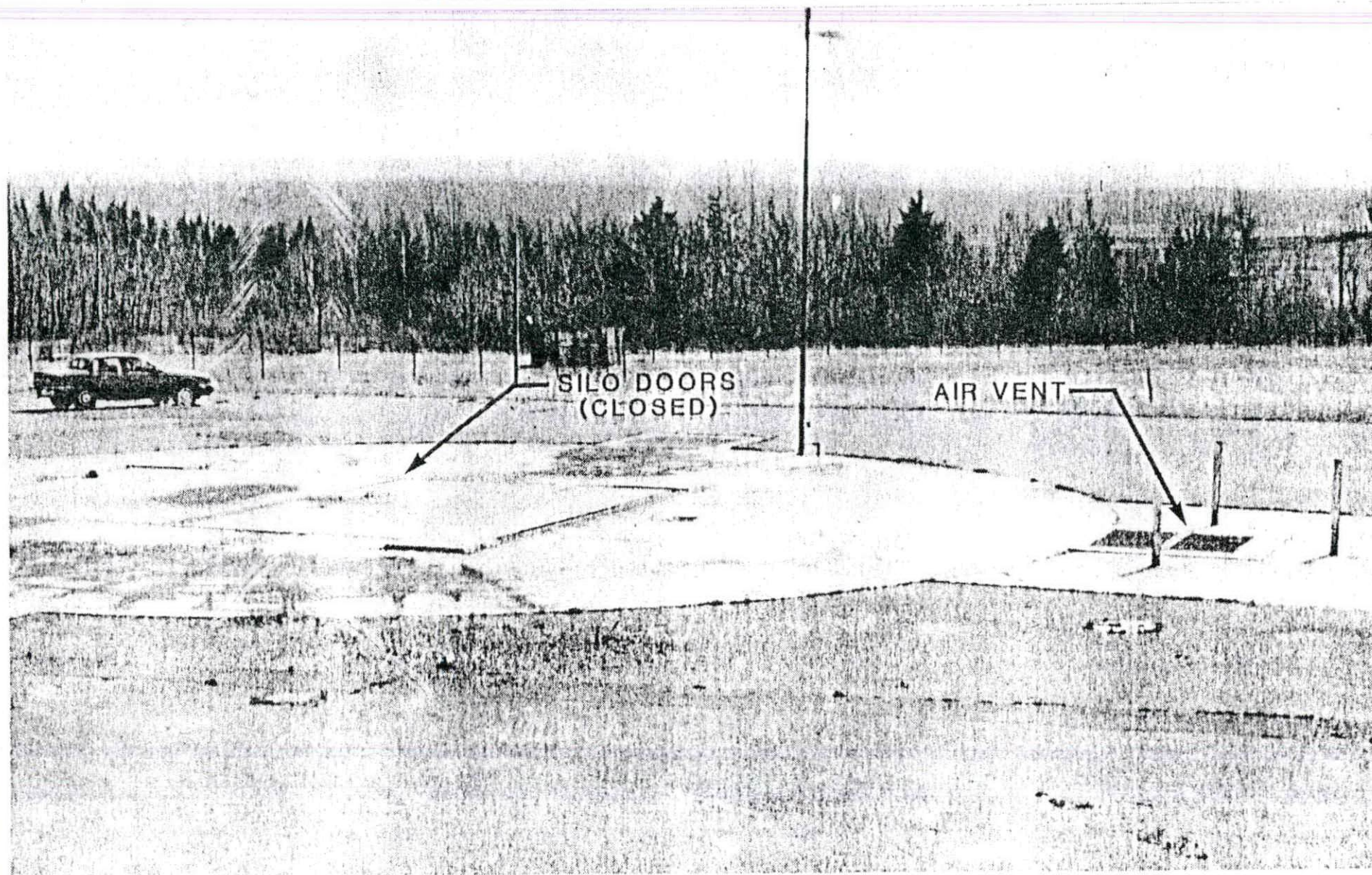
FIGURE 2-3 SILO DOORS AND CONCRETE PAVEMENT ATLAS SITE S-11 - ELLENBURG, NEW YORK
