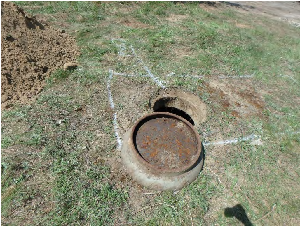
Photo 7 – Small concrete vault, May 2018
