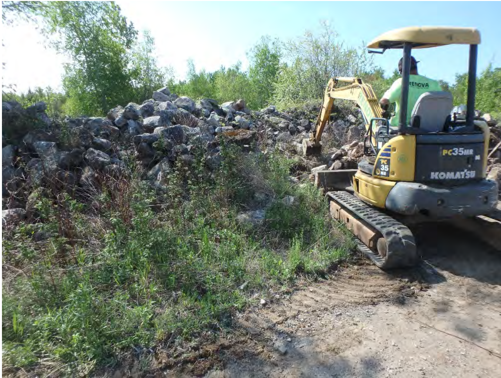
Photo 5 – Renova performing as much clearing as possible, May 2018
