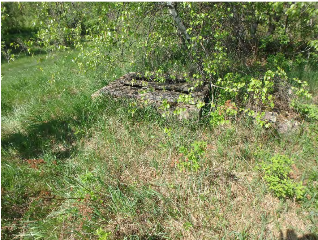
Photo 6 – Large concrete vault, May 2018
