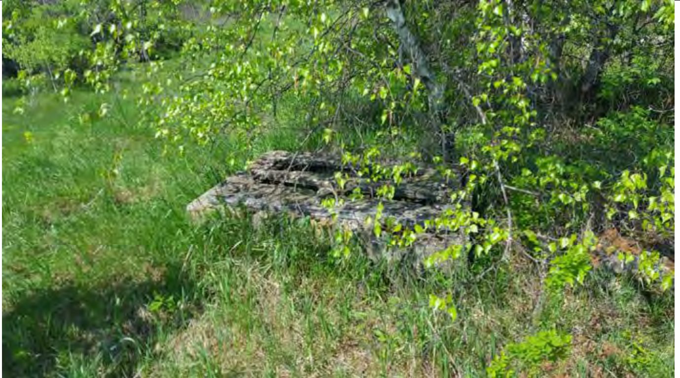
A concrete vault located east of and outside of the survey area appears to be the destination of the metal pipe in Photos 5-8. The pipe enters this vault at a depth of around 6'.
