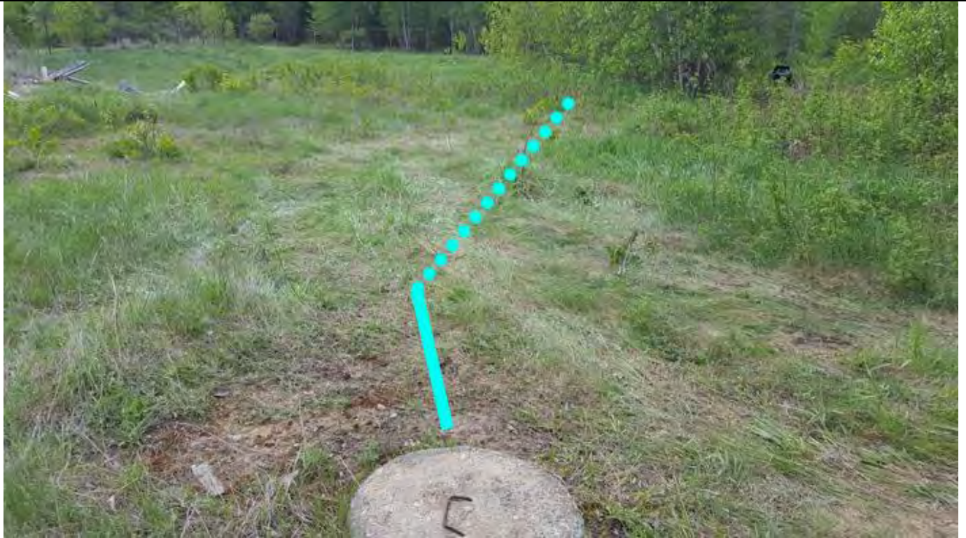
South facing view showing the trace of a metal pipe leading from one concrete vault to another.
