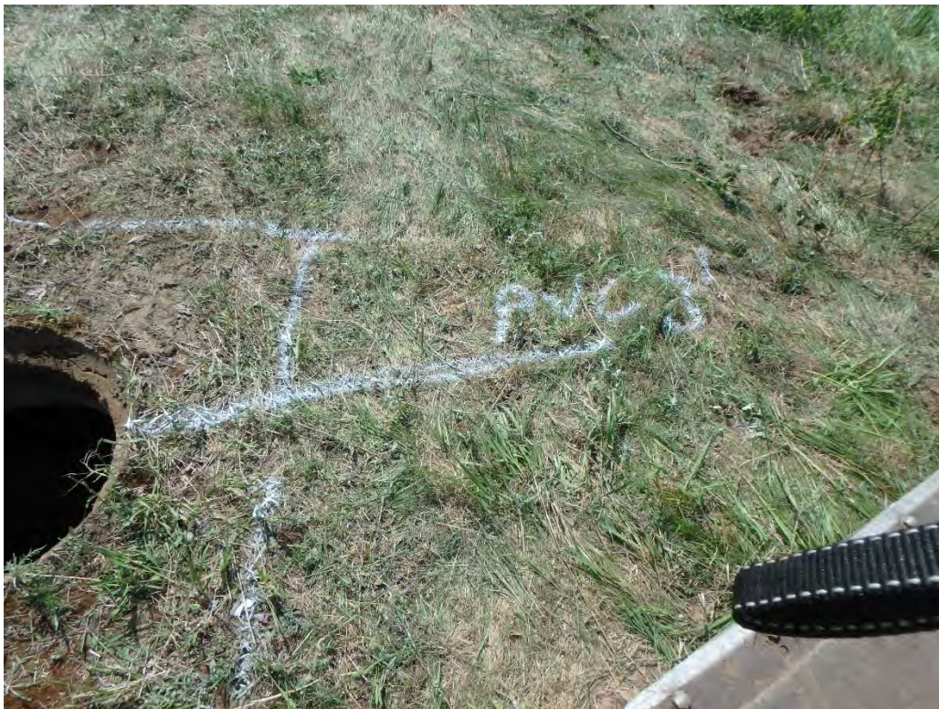
Photo 10 – PVC piping identified during GPR survey, May 2018
