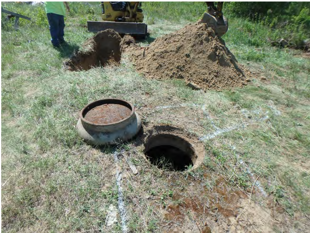
Photo 14 – Metal pipe excavation in relation to small concrete vault, May 2018
