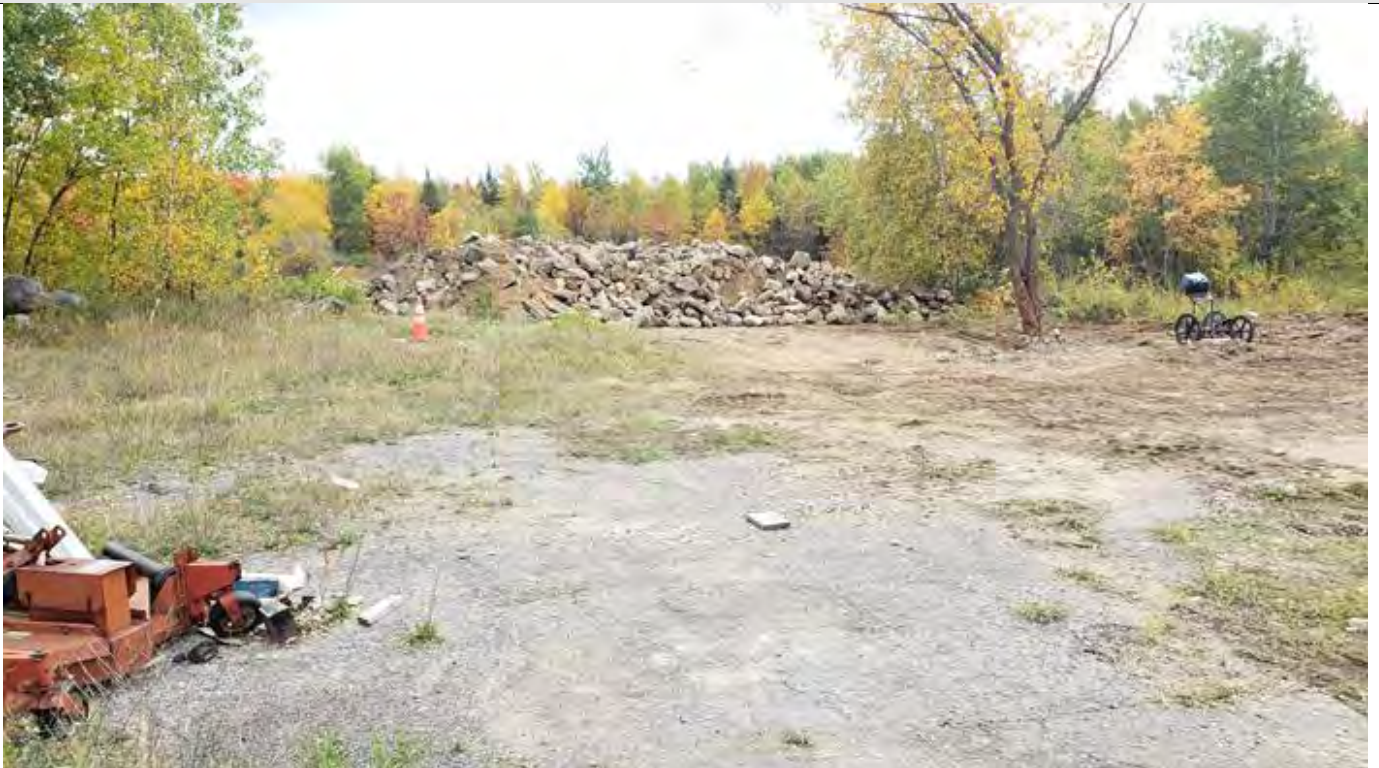
Southeast facing photo shows the project area cleared of rock piles. The orange cone marks the manhole associated with the concrete vault.
