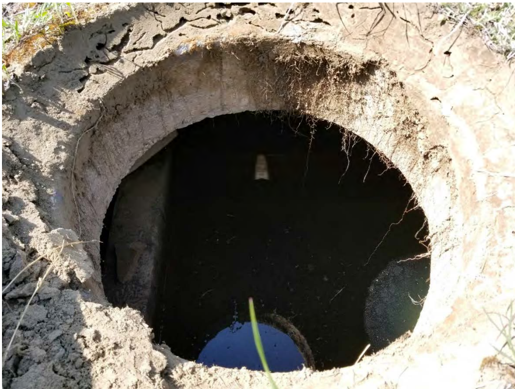
Photo 8 – Small concrete vault interior, May 2018
