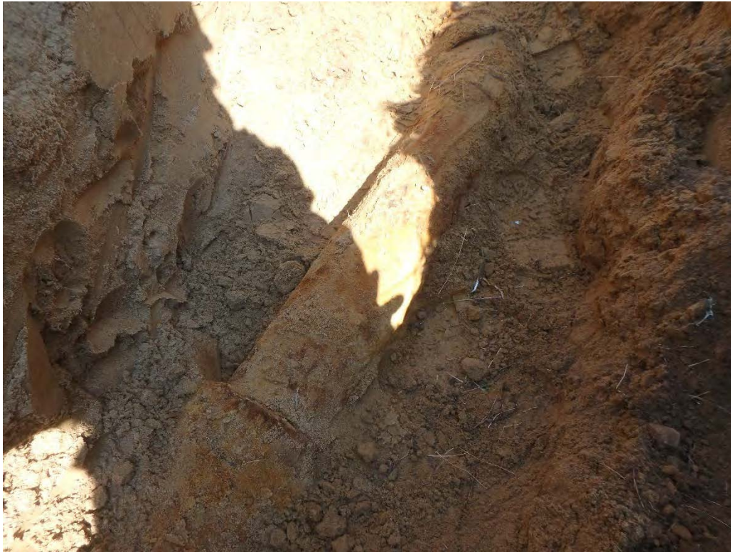
Photo 13 – Test pit activities reveal 8” metal pipe, May 2018
