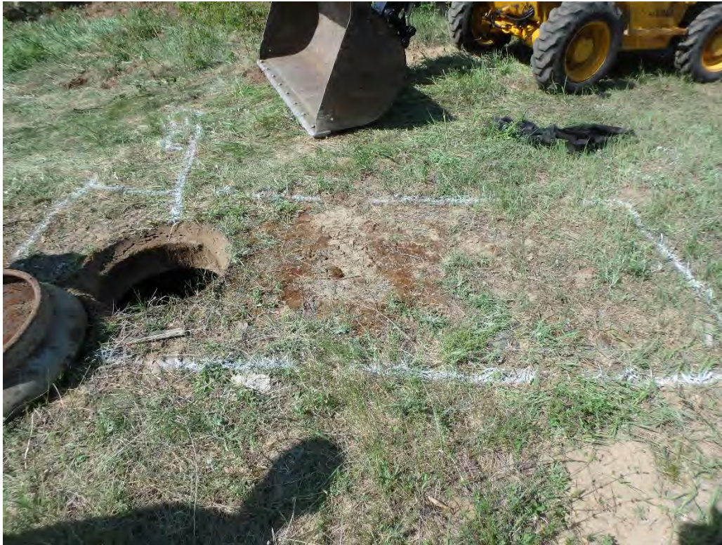
Photo 11 – Estimated limits of small concrete vault, May 2018
