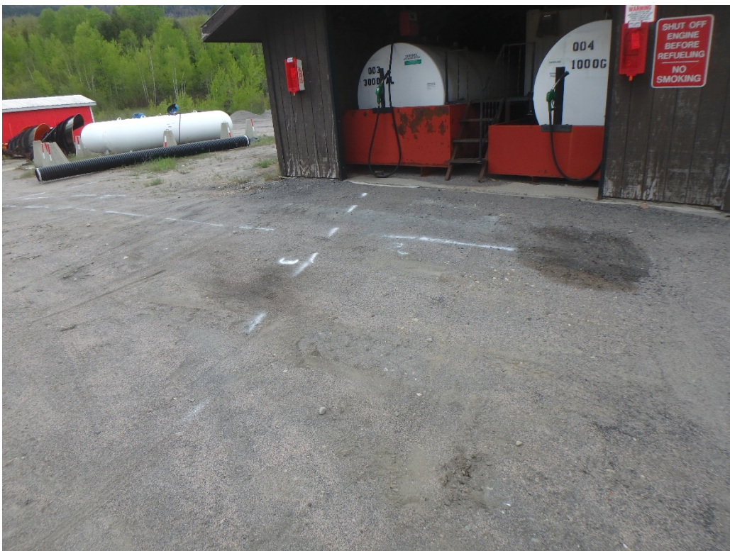
Photo 4 – Underground utilities leading to township fueling station
