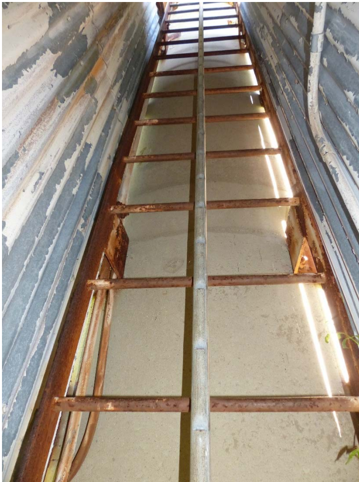
Bolt steel plate across bottom ten feet of tower access ladder. (typical for three towers)
