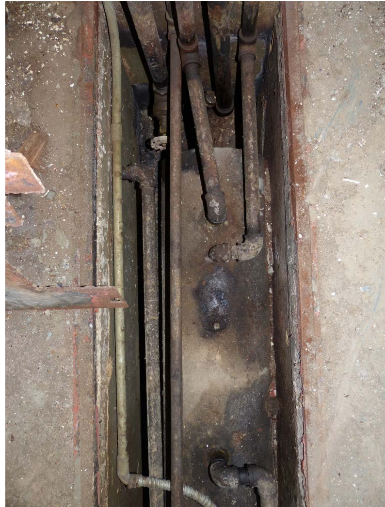
Tank located in trench in building floor slab. Portions of the associated fuel piping are shown.
