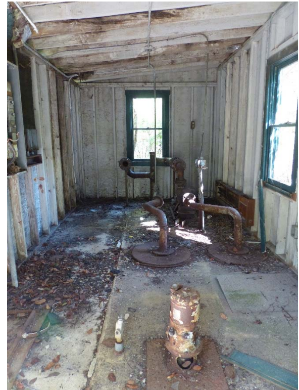
Interior view of Pump House shows pump and much of the remaining piping.
