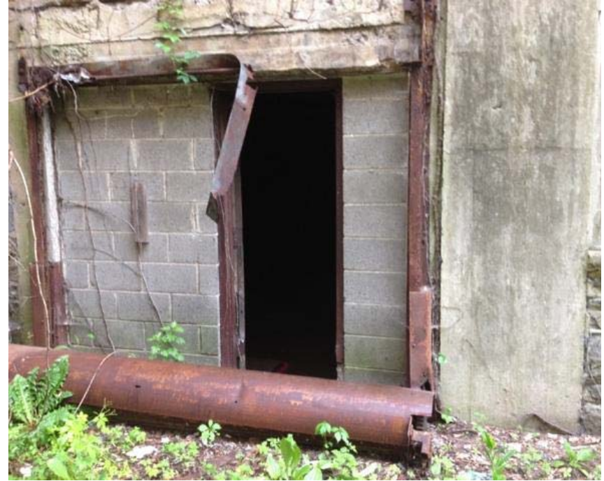
Basement doorway opening must be enlarged and debris cleared to facilitate removal of the transformers.
