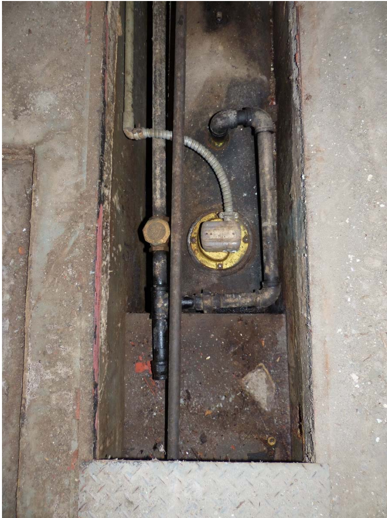
Tank located in trench in building floor slab. Portions of the associated fuel piping are shown.
