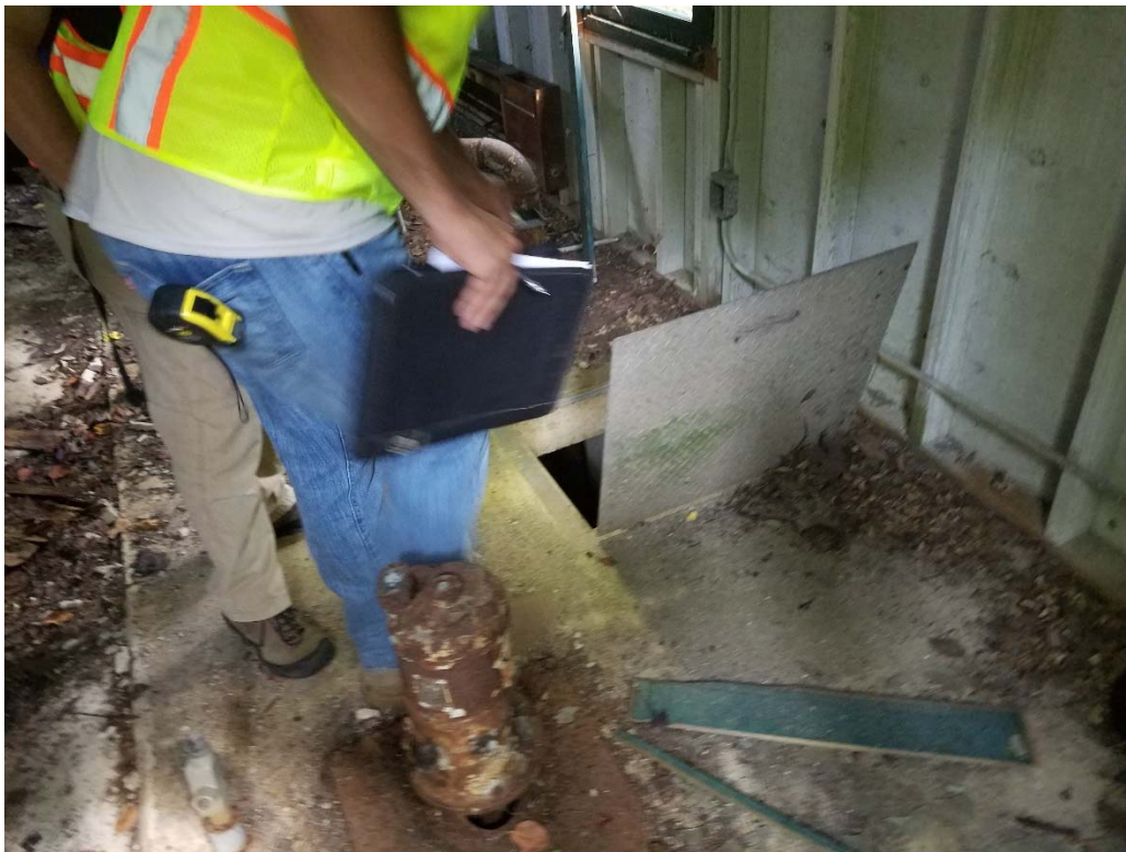
Pump chamber hatch
