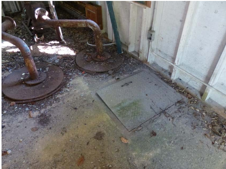
Place clean fill in Pump House chamber to fill completely to grade.
