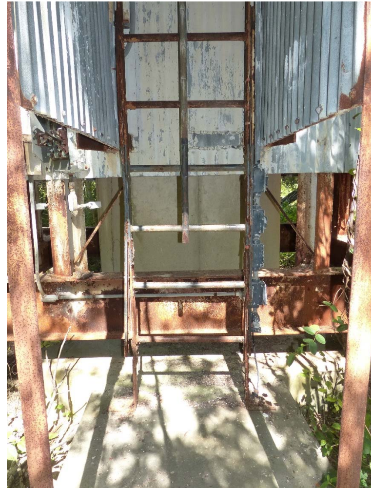
Radar Tower access ladder (typical for four towers).
