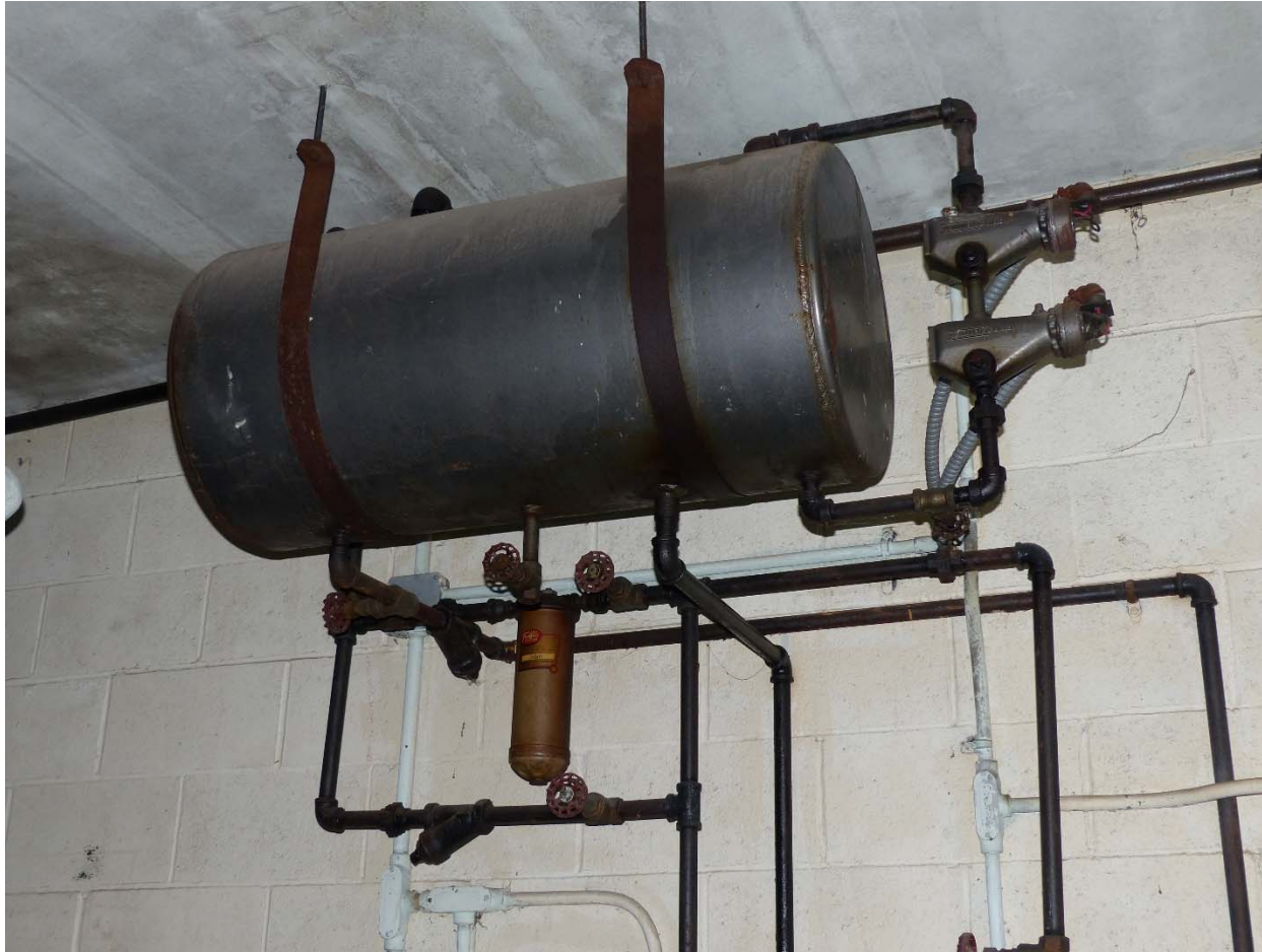
Day tank hung from ceiling. Portions of the associated fuel piping are shown.
