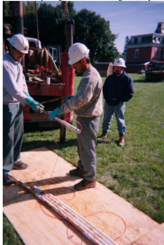
Photo 8: Disposing of PVC from Angle Well packer.
