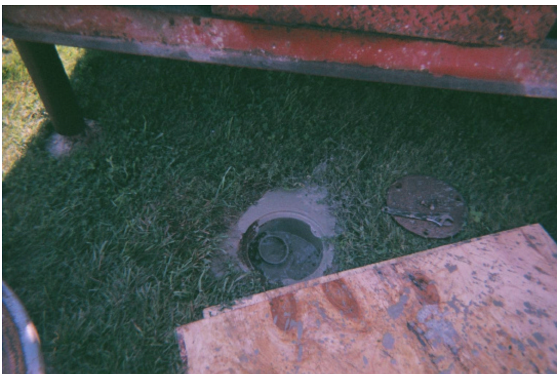
Photo 14: Angle Well after grouting.
