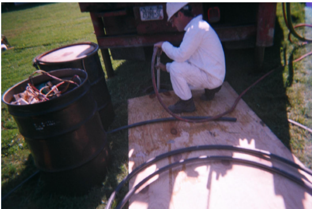
Photo 13: Grouting up Angle Well.
