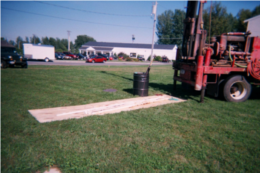
Photo 1: Angle Well packer removal.
