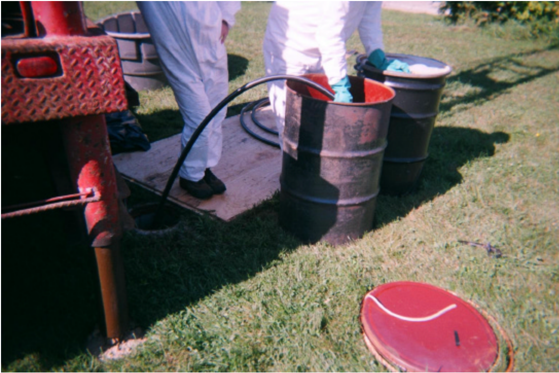
Photo 10: Purge out standing water in Angle Well.
