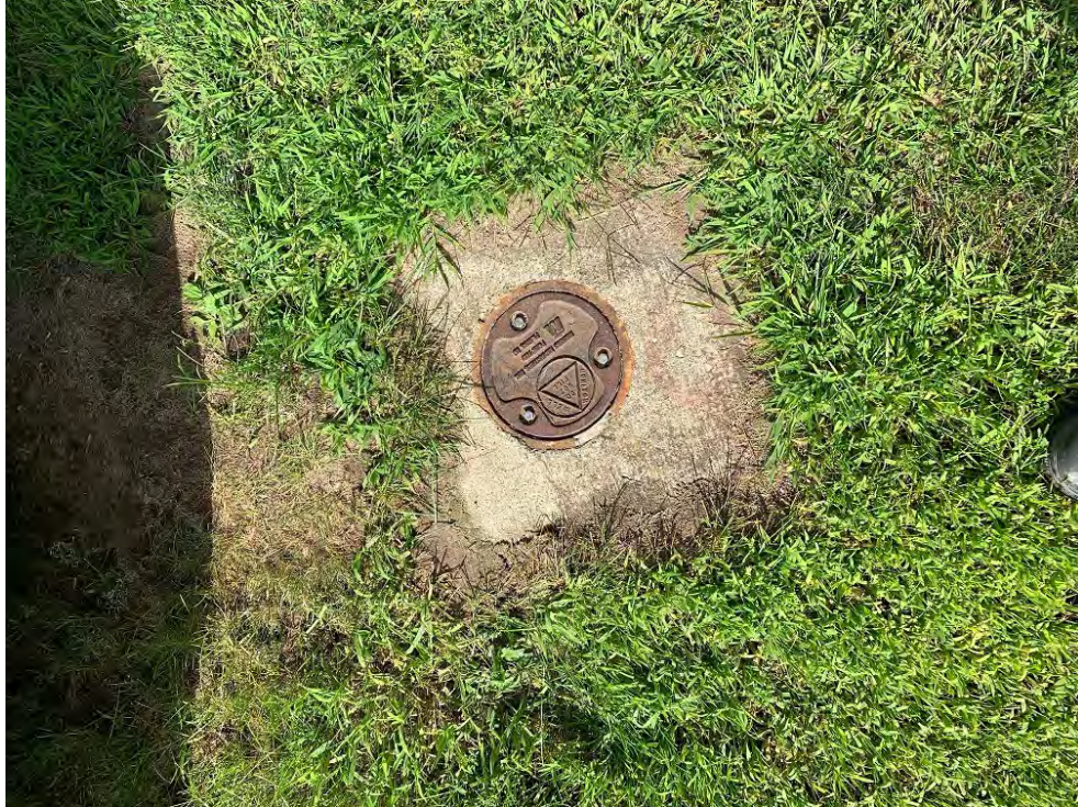
Photo 3: On-Site Groundwater Monitoring Well MW-9B
