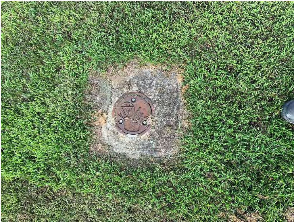
Photo 2: On-Site Groundwater Monitoring Well MW-7BD
