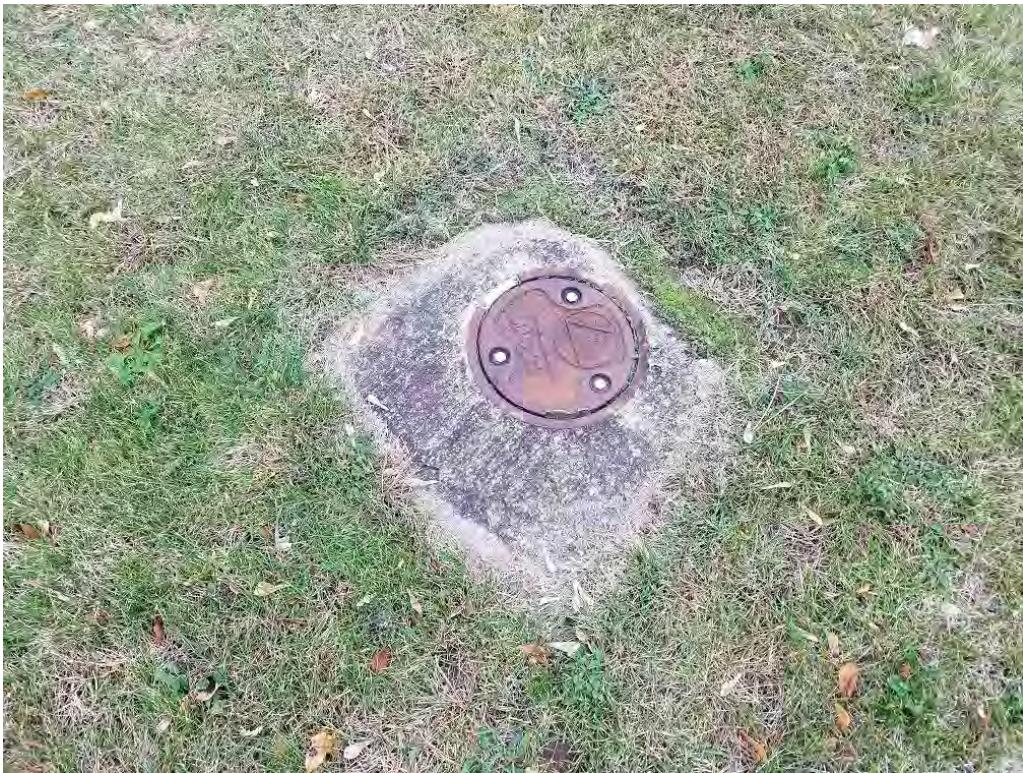
Photo 2: On-Site Monitoring Well Example (MW-7BD)
