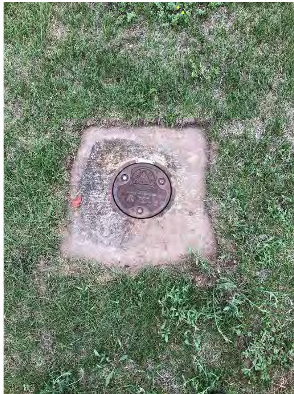
Photo 2: On-Site Monitoring Well Example
