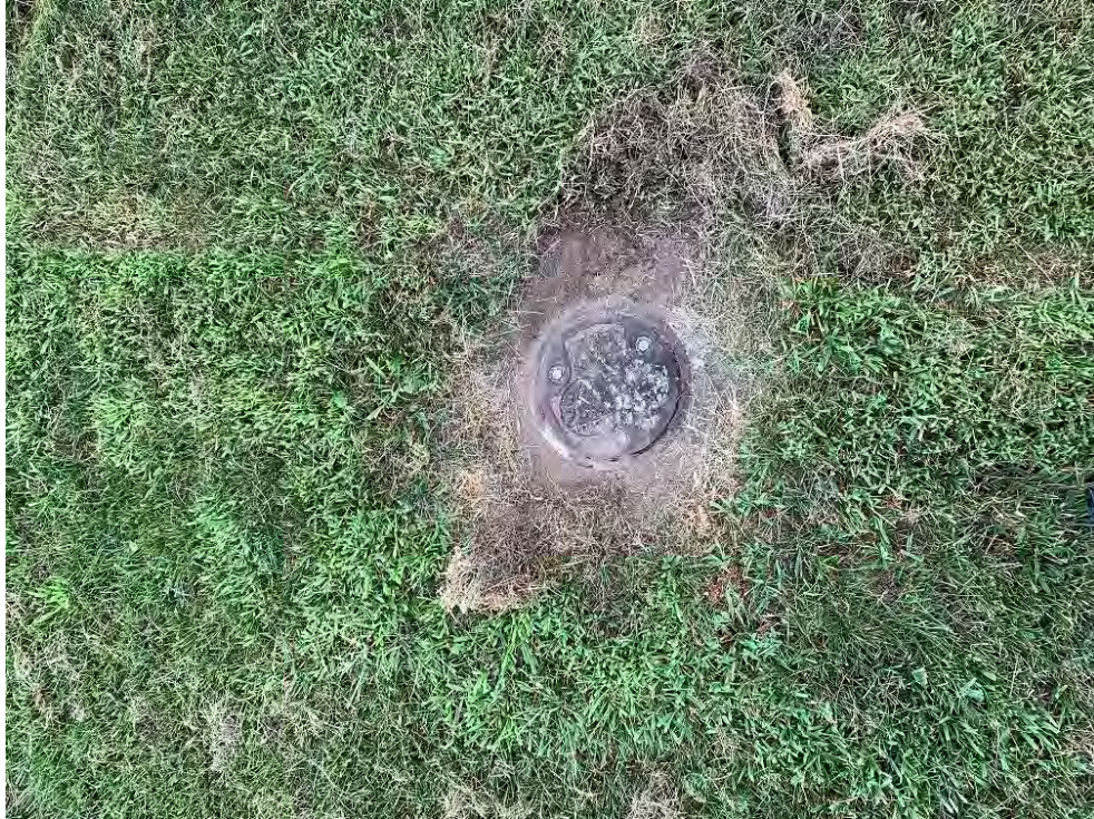
Photo 9: On-Site Groundwater Monitoring Well MW-2B
