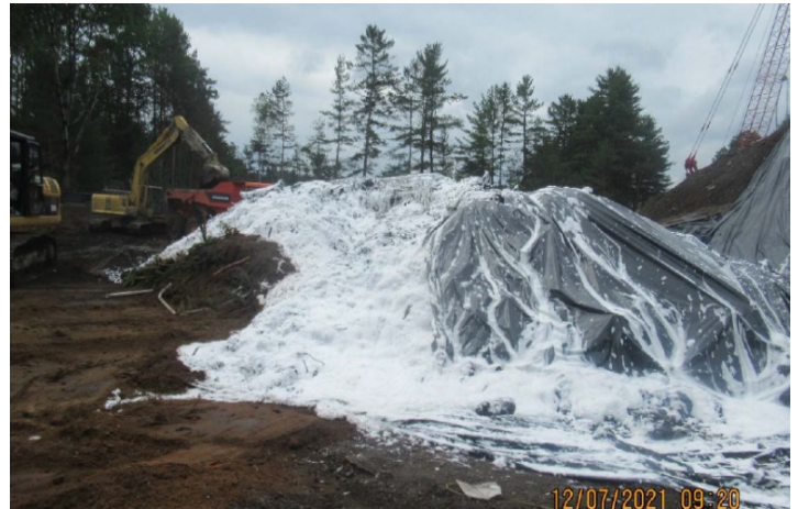
Foam being applied to the stockpiled material.
