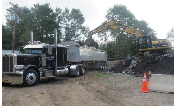
Loading impacted soil for off-site disposal.
