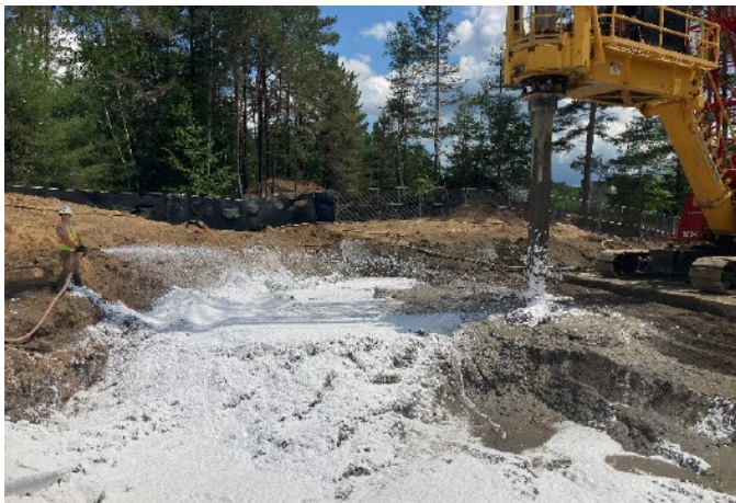
Foam being applied during ISS.
