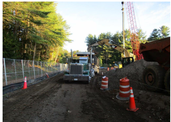
Loading Impacted Soil for Off-site Disposal.
