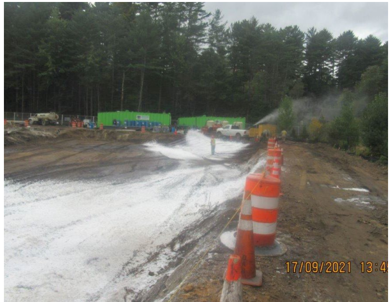
Spraying Foam on Exposed Areas that have been prepared for ISS.
