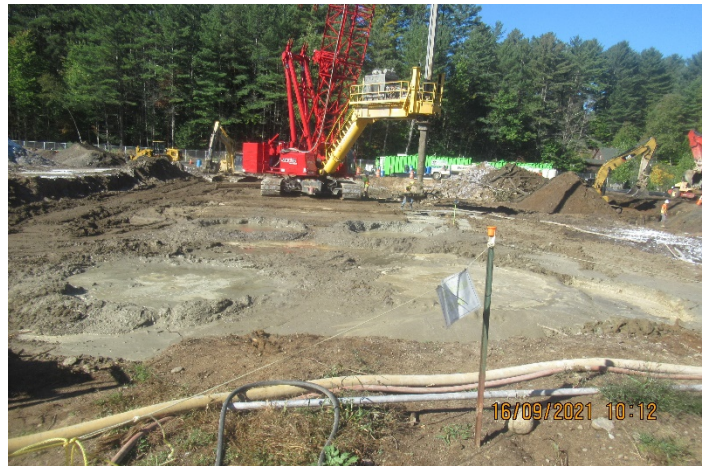
Completed ISS Columns Prior to Curing.
