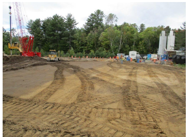
Area Where ISS is Complete with First Layer of Re-Usable Soil Compacted.
