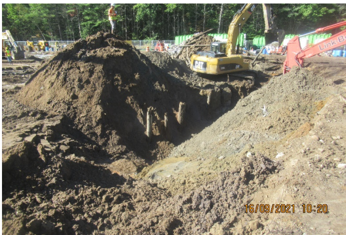
Excavating Demolition Debris Including Wooden Piles Located Beneath an 80-foot Diameter Concrete Foundation.
