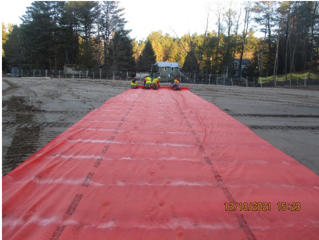
Soil and placement of demarcation fabric to construct the cover over the ISS Area.
