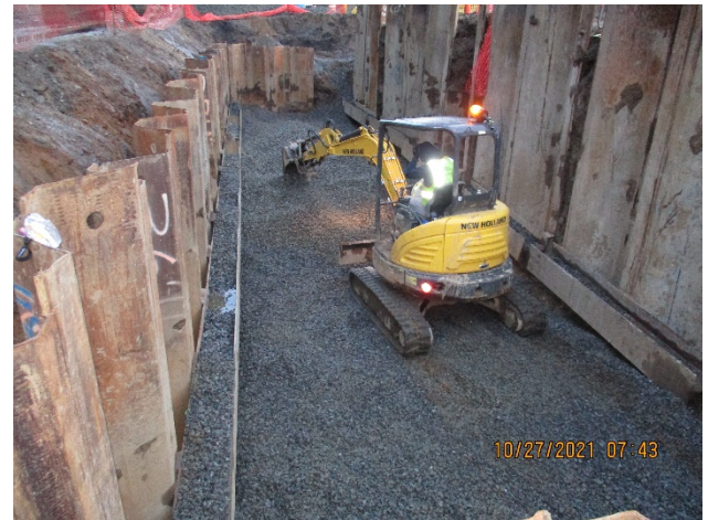
Backfilling an excavation on the southeast side of the site
