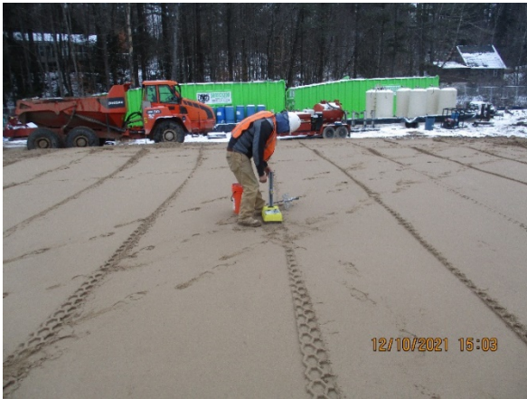
Compaction testing of reusable soil
