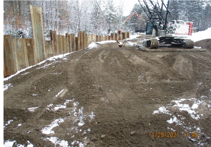
Removing sheet piles from excavation adjacent to Brandy Brook.
