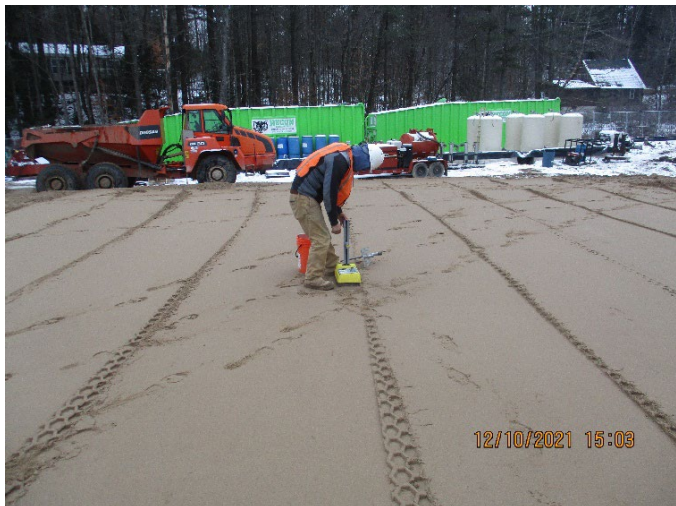
Compaction testing of imported soil and placement of demarcation fabric to construct the cover over the ISS Area.
