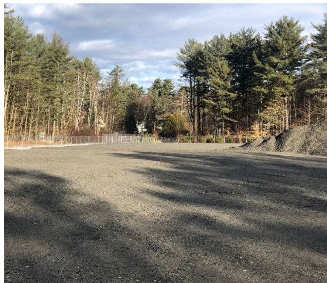
Photo from the March 21, 2022 Site Inspection.
