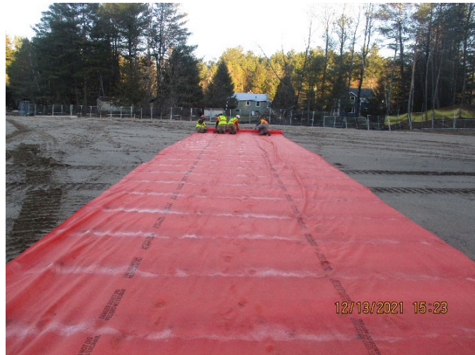
Compaction testing of imported soil and placement of demarcation fabric to construct the cover over the ISS Area.
