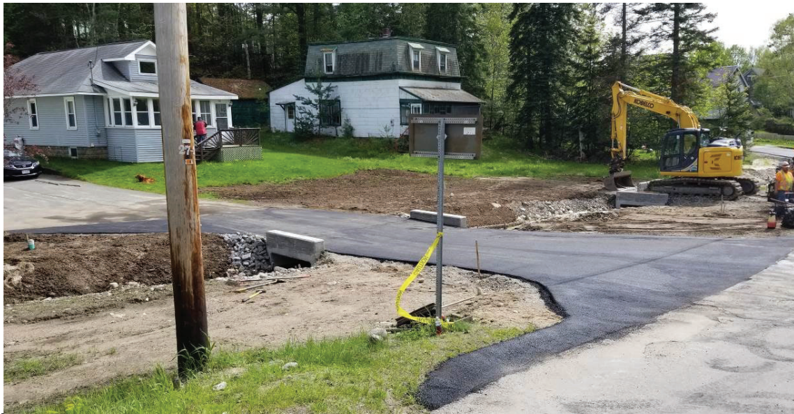
FO14-01 Existing driveway with new curbing at 38 and 42 River Street
