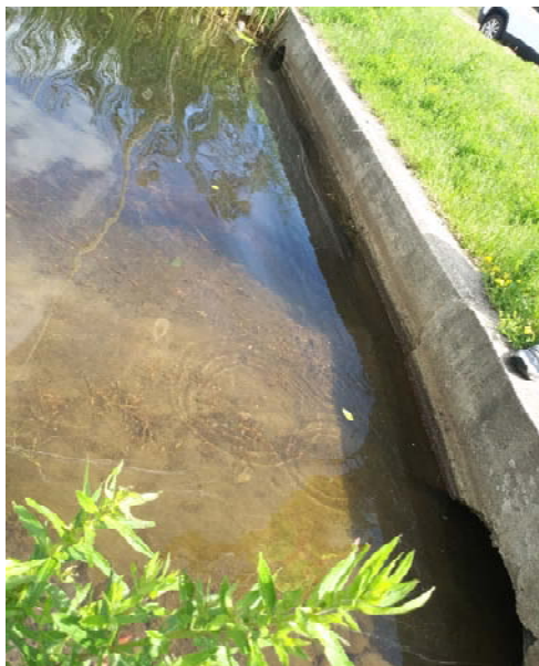
Sedimentation at downstream end of culvert entering Pontic Bay
