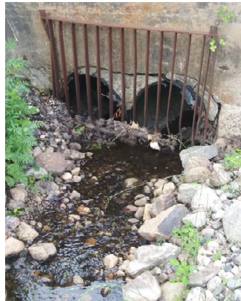
Debris at upsteam end of culvert entering Pontiac Bay
