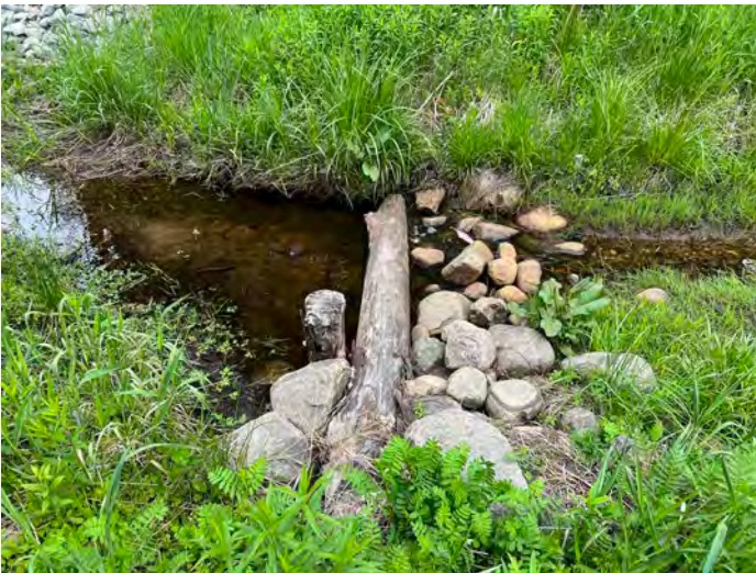
Photograph 35: Drop log structure within the restored stream channel within Monitoring Area Wet-2.
