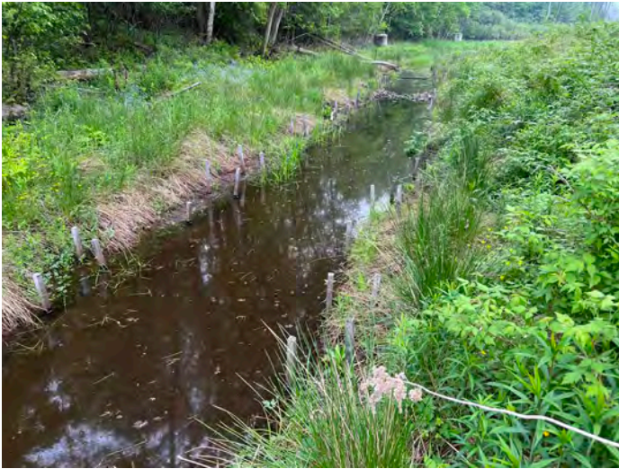
Photograph 25: View of stable stream channel bank with core log structure along Area BB-2.
