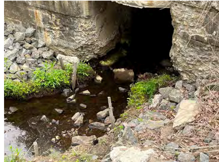
Photograph 20: Erosional deterioration of historic culvert on the northern end of Monitoring Area BB-2.
