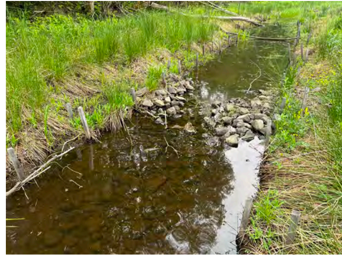
Photograph 26: Stable rock vane structure within Brandy Brook within Monitoring Area BB-2.
