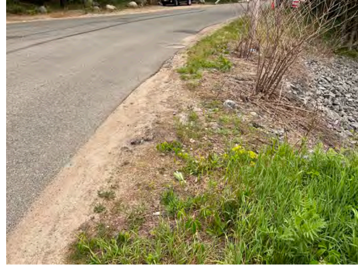
Photograph 18: Area of street runoff along the top of banks of Brandy Brook at the northern portion of BB-2.
