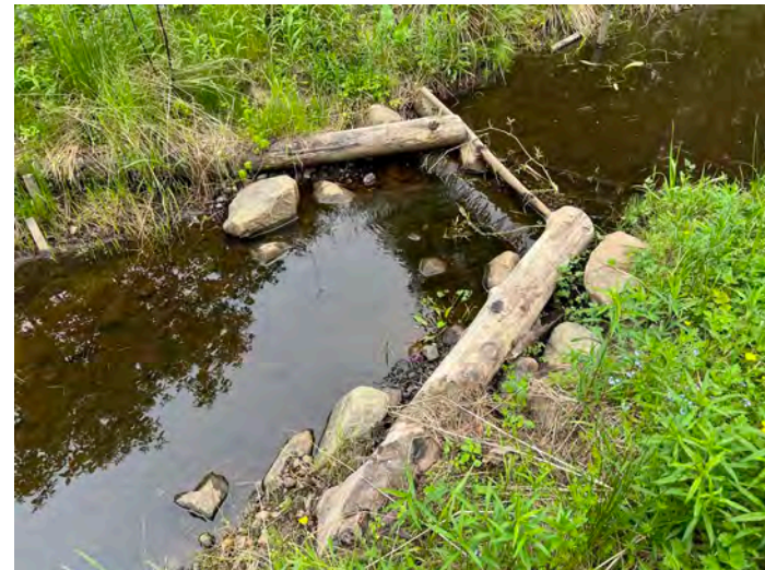
Photograph 24: Stable drop log structure observed along Brandy Brook within Monitoring Area BB-2.
