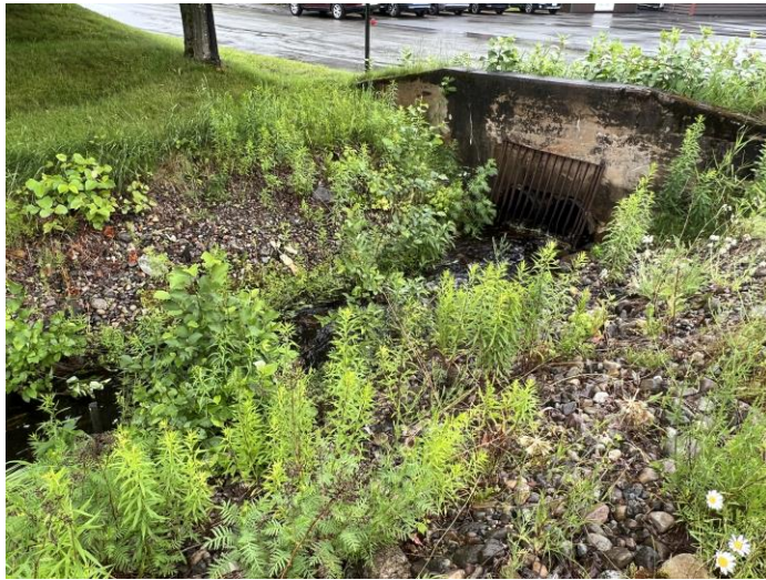
Photograph 13: Rip rap bank and partially vegetated areas at the northwestern portion of Brandy Brook.
