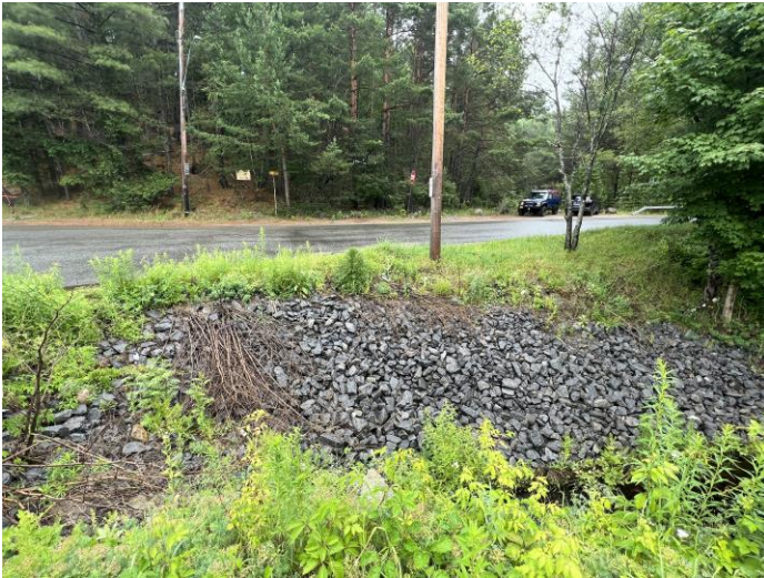
Photograph 19: Rip-rap slope of Brandy Brook at the northern end of BB-2 along Brandy Brook Avenue.
