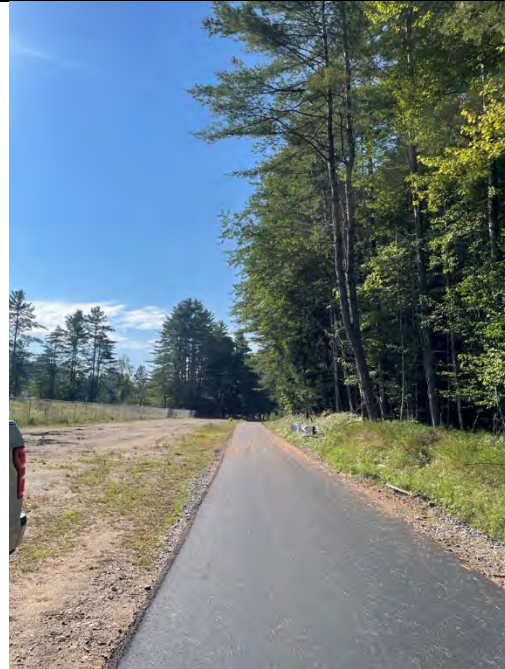
Newly paved rail trail – facing south
