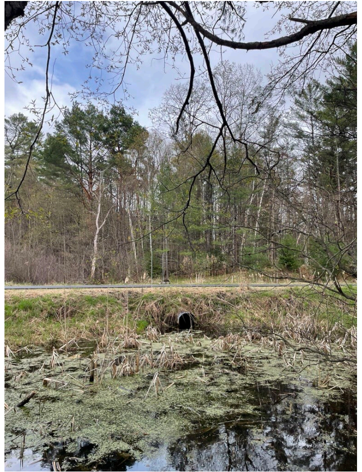
Unobstructed outfall (behind PZ-301)
