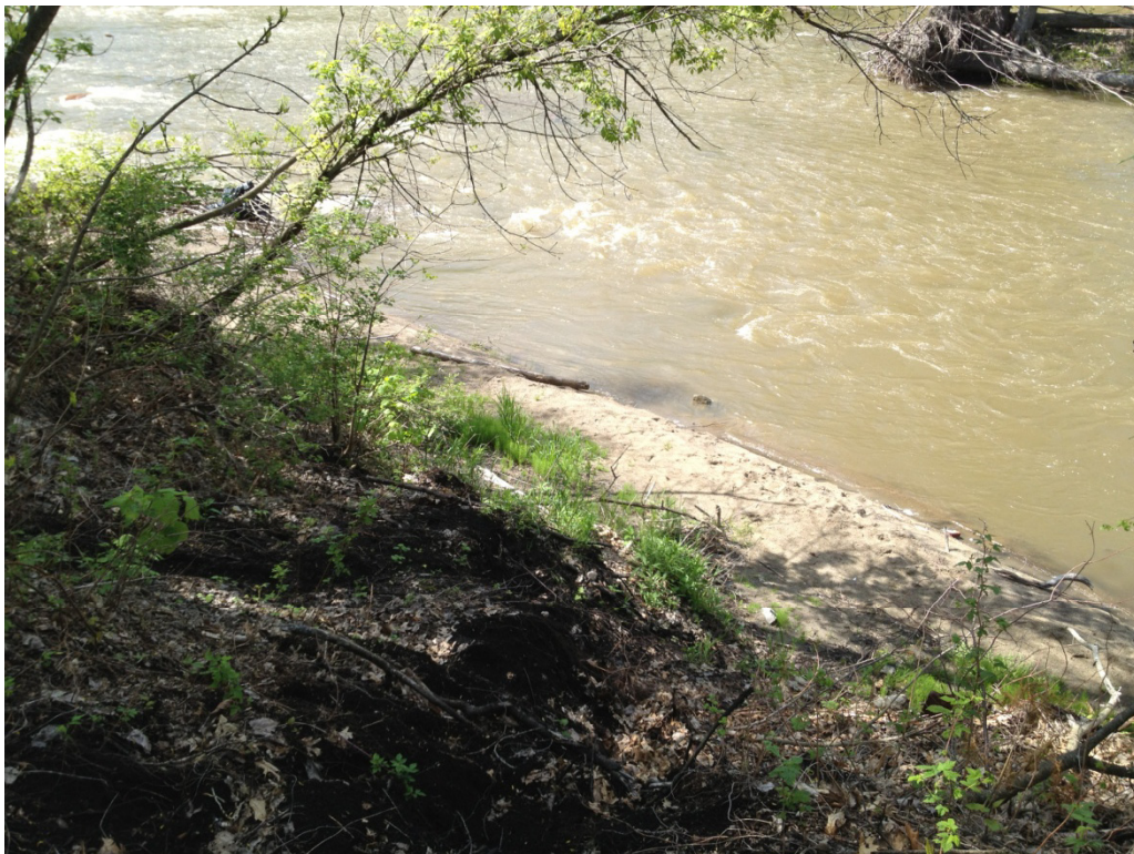
Photo 6: Looking north-northwest from on top of berm near Section 8+00.
