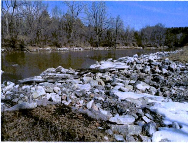
Picture # 4: View of inlet/outlet (exterior)
