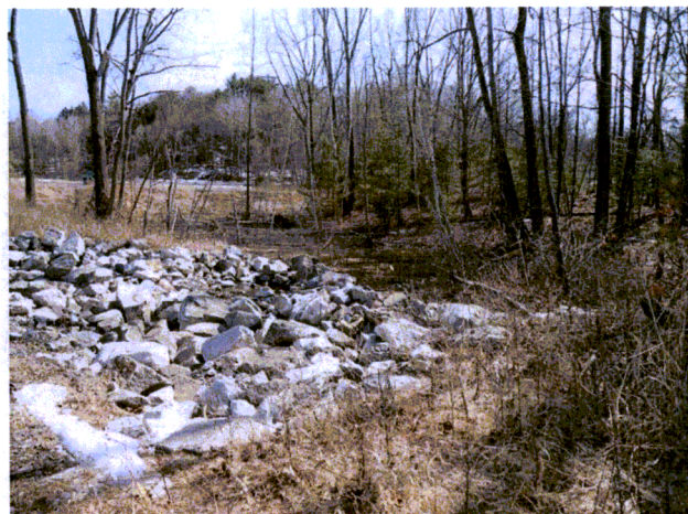
Picture # 3: View of inlet/outlet (interior)
