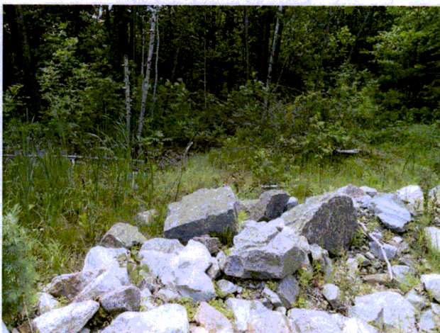
Picture # 12: View of interior inlet/outlet
