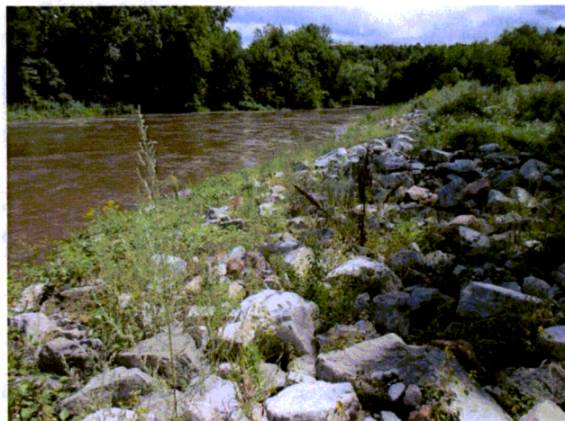
Picture # 9: View of riprap from inlet/outlet looking downstream
