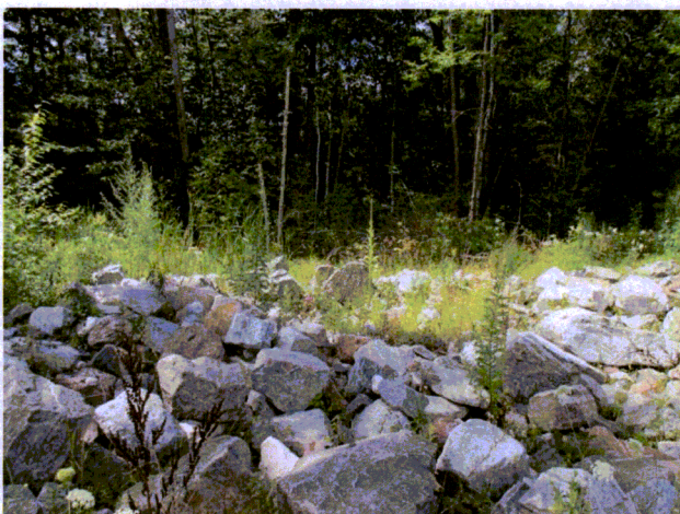
Picture # 12: View of growth and riprap at interior side inlet/outlet
