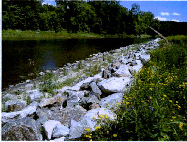
Picture # 4: View of deposition on riprap and growth on slope and in riprap
