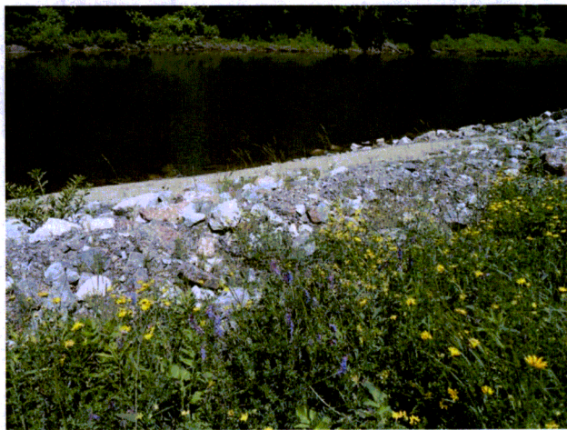
Picture # 8: View of edge at inlet/outlet
