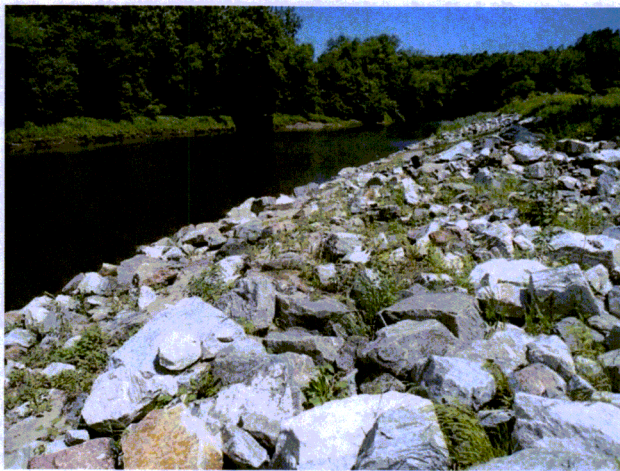
Picture # 11: View of perimeter edge looking downstream from inlet/outlet
