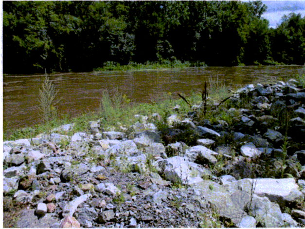
Picture # 7: View of exterior inlet/outlet
