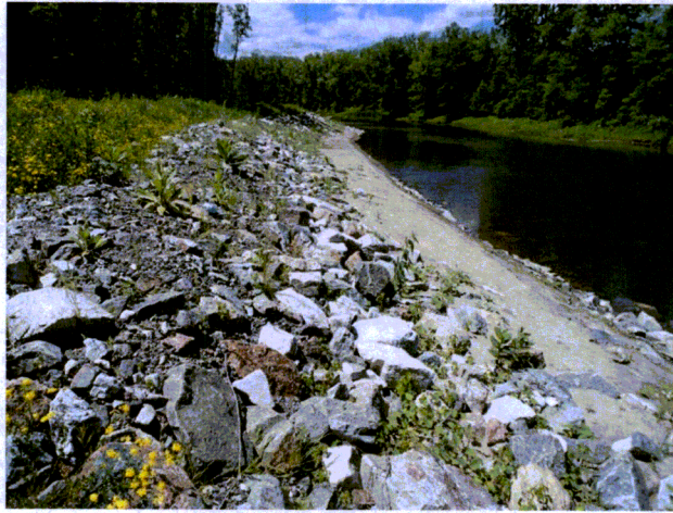
Picture # 10: View of perimeter edge looking upstream from inlet/outlet
