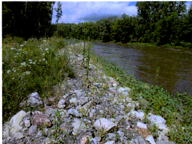
Picture # 8: View of riprap from inlet/outlet looking upstream
