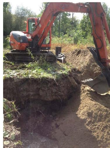
Figure 1-3 Backfilling IRM excavation with clean fill
