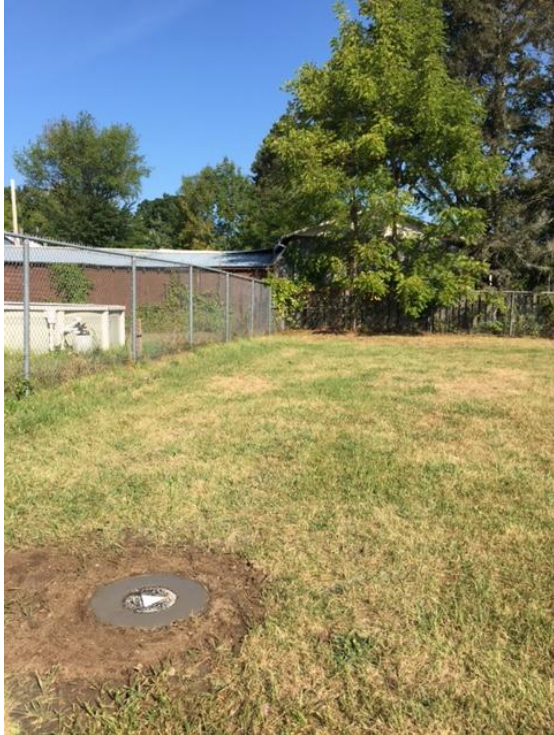
5) MW-22 completed installation – 9/16/15.
