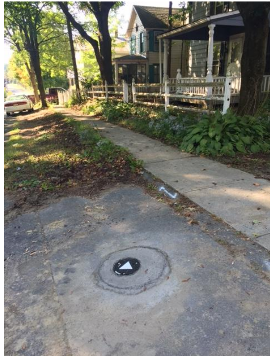
2) MW-19 completed installation – 9/15/15.
