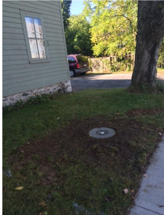
4) MW-21 completed installation – 9/15/15.
