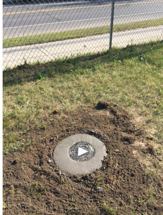
6) MW-23 completed installation – 9/15/15.
