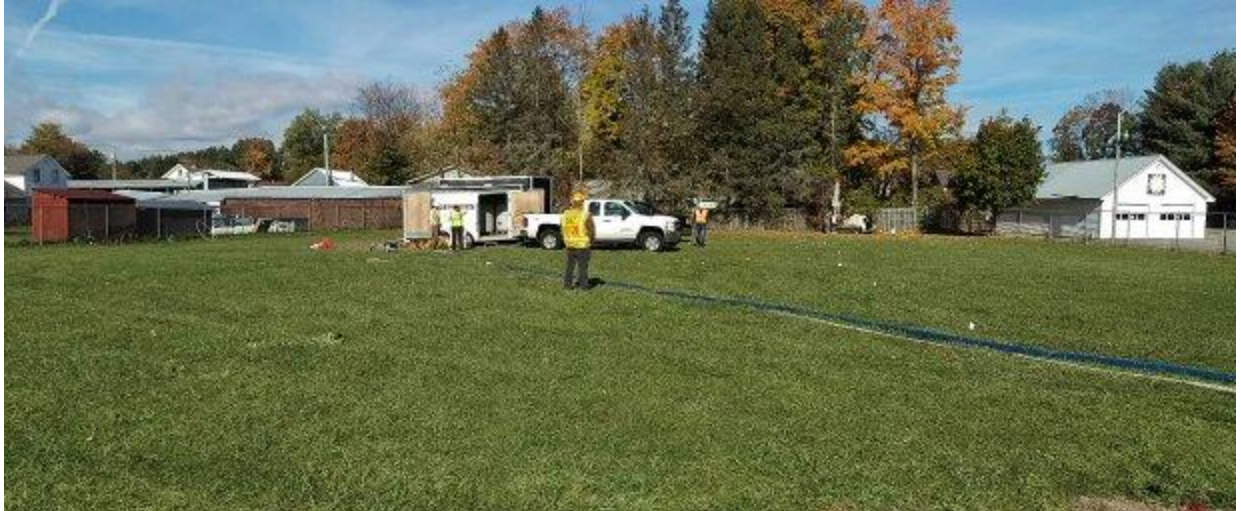
8) View on site to northeast during ISCO injection work – October 20, 2015.
