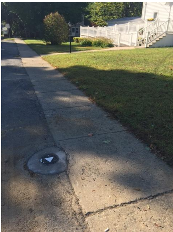
3) MW-20 completed installation – 9/15/15.
