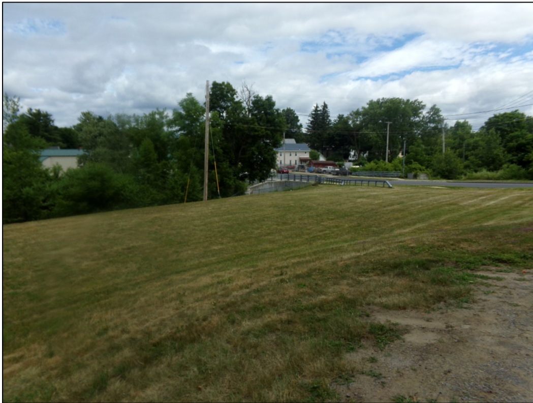
Site Conditions – July 8, 2025
