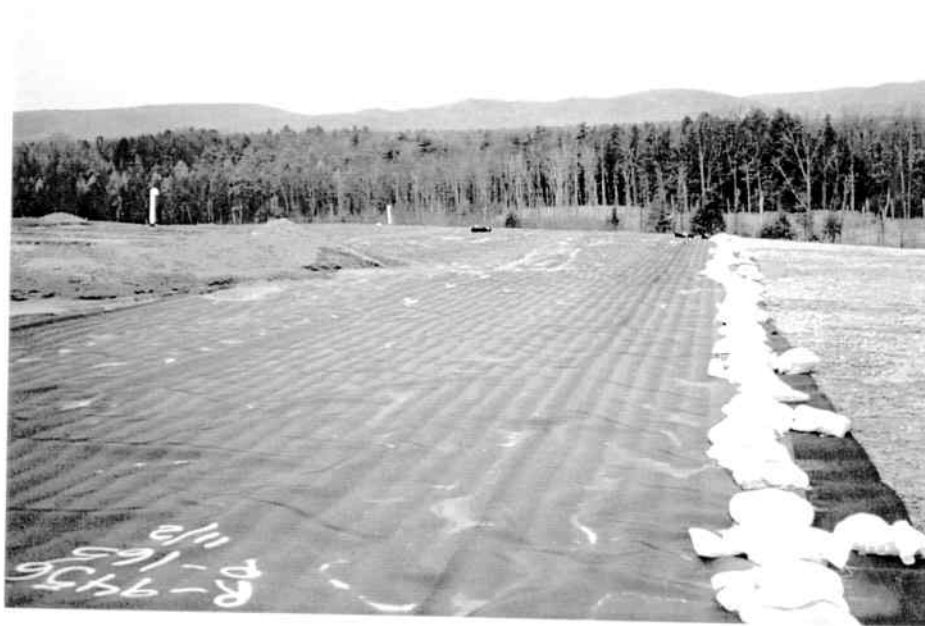
Geomembrane panel P-165 at West slope
