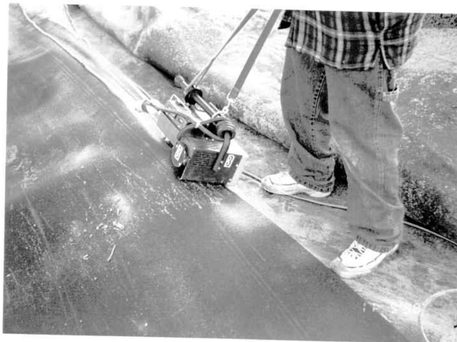
Dual Hot Wedge Seamer – welding two geomembrane panels together
