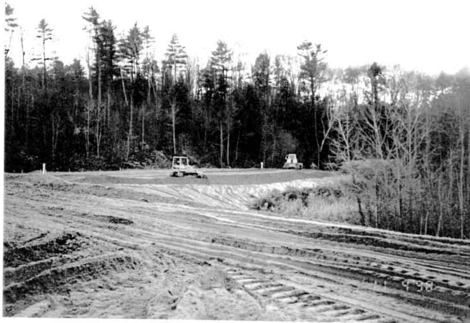
Placing barrier protection material at SW corner of landfill
