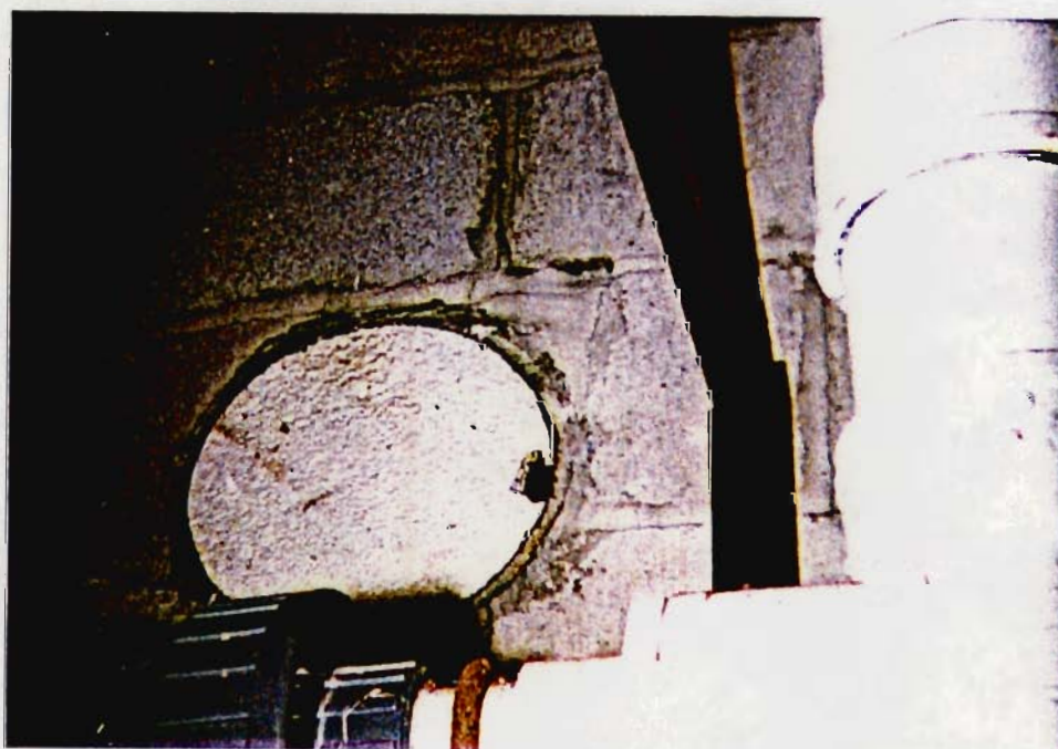
Photograph 12: Southwest interior wall of Building 15. This is an exhaust port for the heating furnace. The port enters the brick chimney. The furnace, now removed, was located below the port. Fuel feed lines entered the building below ground surface and through floor.
