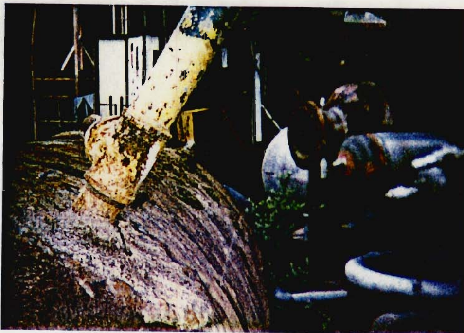
Photograph 19: Top of Tank 1 (3,000 gallon gasoline tank).
