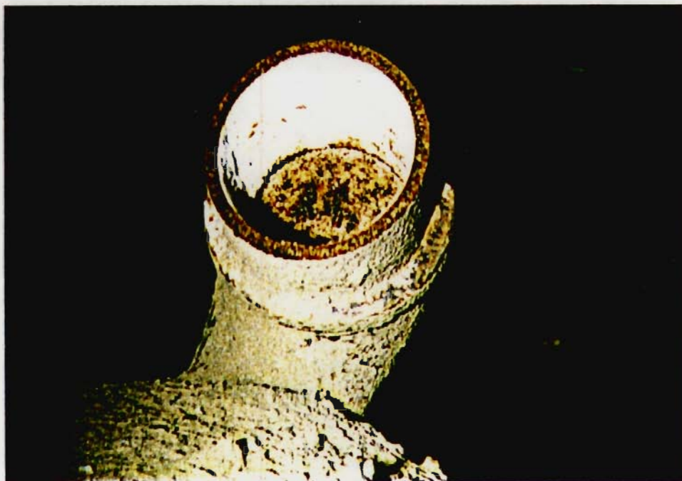
Photograph 23: Fill pipe at top of Tank 1.
