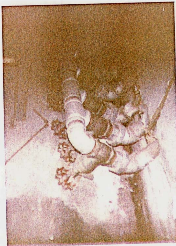
Photograph 16: Northwest interior wall of Building 28. Fuel oil pipes from Tanks 4 and 5 connected to one line leading to a furnace in Building 28H.
