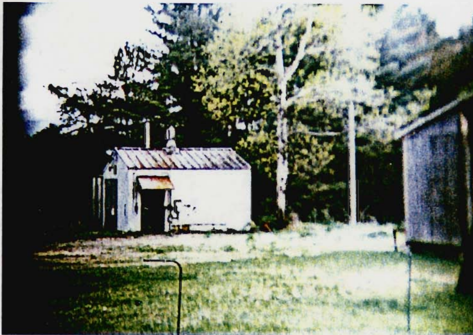
Photograph 13: Building 28 and 28H (center) and northeast wall of Building 10 (right edge of photo). This was the site of the two 6,000-gallon, fuel oil tanks (Tanks 4 and 5).
