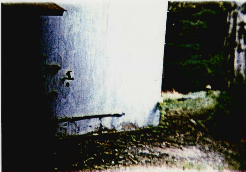
Photograph 15: Northwest wall of Building 28. Fuel oil pipes from Tanks 4 and 5 entered the building through the holes at the base of the wall.
