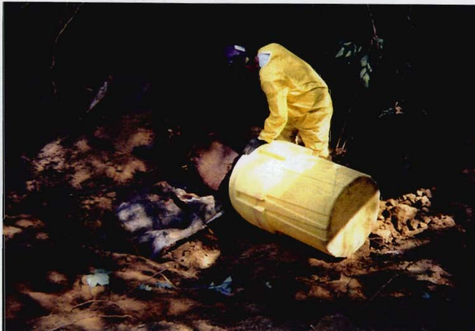
Photo 24 - Overpacking of stainless steel drum containing liquid and sludge, Area S-1 South.
