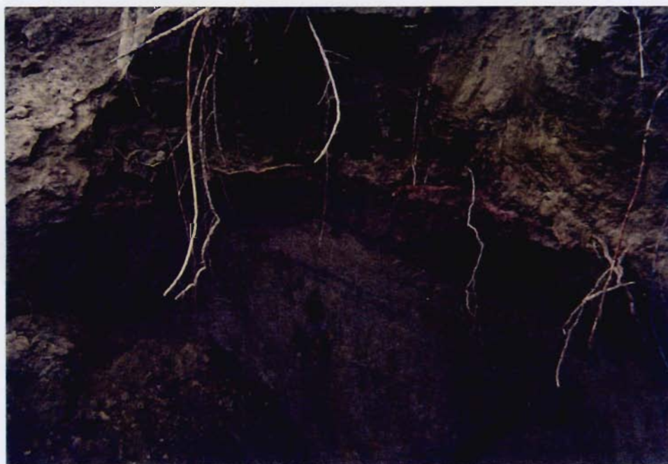
Photo 8 - Area D-1 Excavation.
