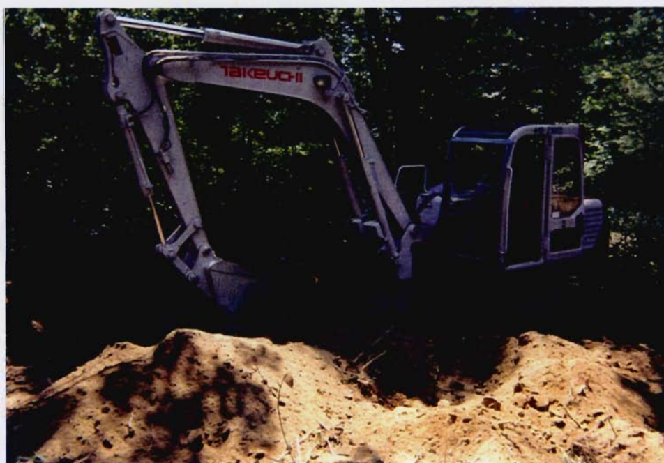
Photo 22 - Drum removal in Area S-1 South.
