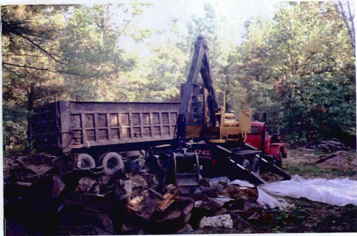
Photo 34 - Loading crushed drums for transportation off-site.
