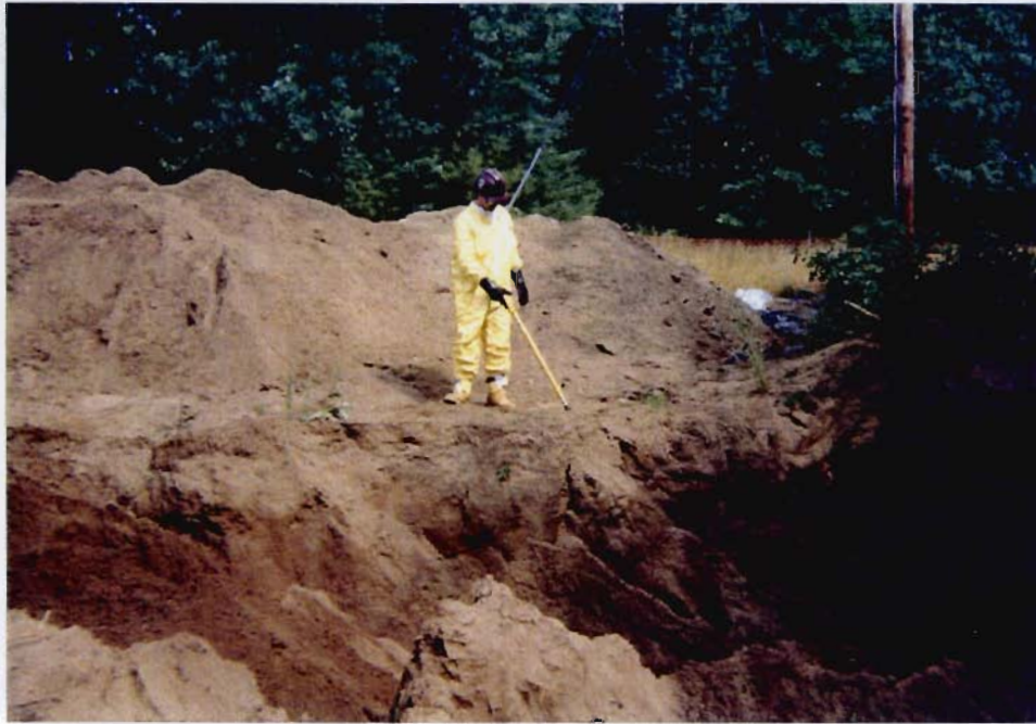
Photo 5 - MC Environmental Services worker screening Area D-1 excavation with metal detector.
