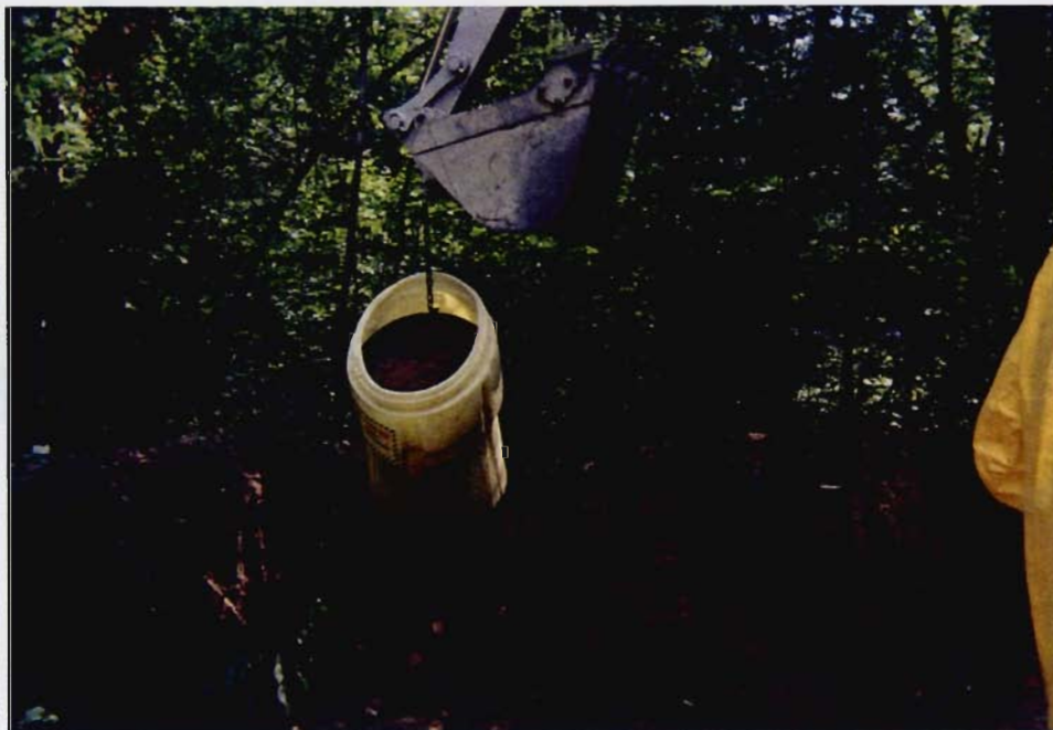
Photo 26 - Staging overpacked stainless steel drum containing liquid and sludge, Area S-1 South.
