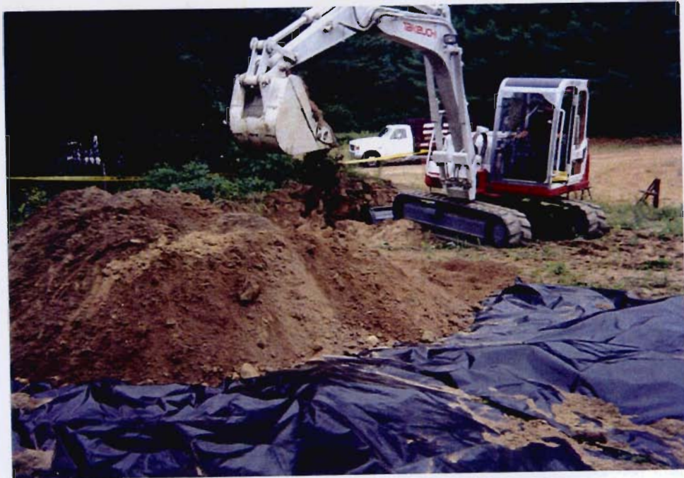
Photo 1 - Excavating in Area D-1.
