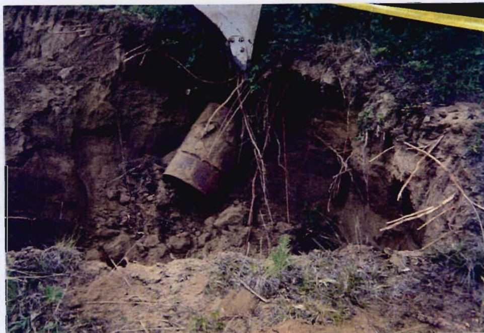
Photo 2 - Drum in Area D-1 excavation.
