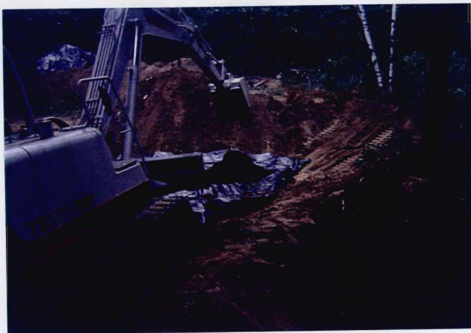
Photo 27 - Staging soil from area where stainless steel drum containing liquid and sludge was found, Area S-1 South.
