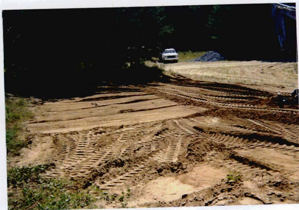
Photo 12 - Area D-1 backfilled.
