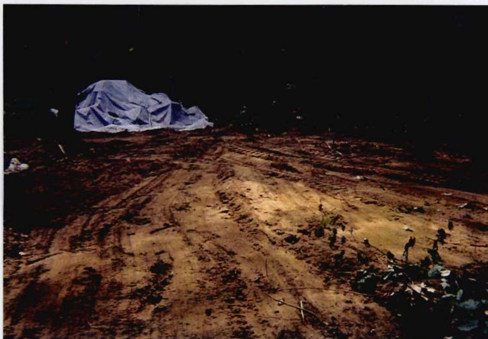
Photo 32 - Area S-1 South backfilled.
