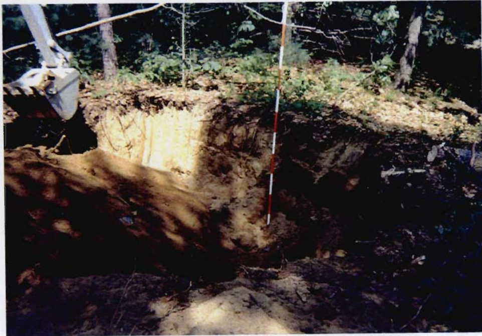
Photo 13 - Excavating in Area S-1 North.
