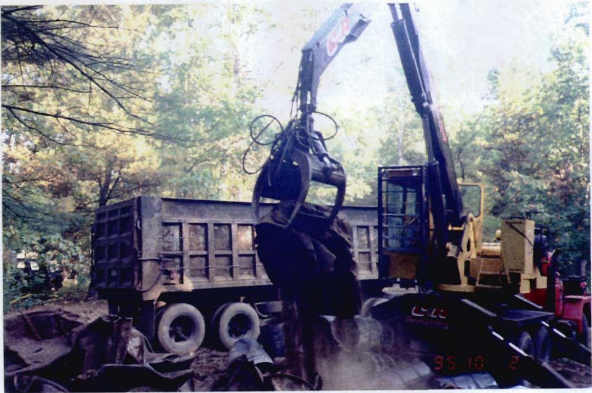
Photo 33 - Loading crushed drums for transportation off-site.
