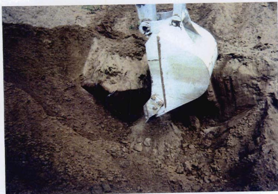
Photo 4 - Drum removal in Area D-1.
