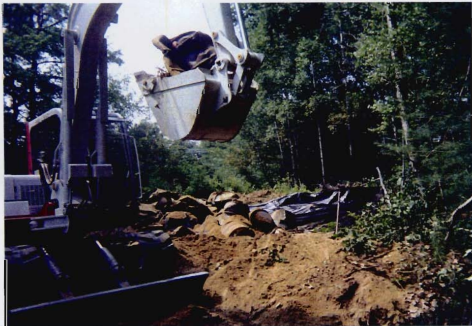
Photo 14 - Drum removal in Area S-1 North.
