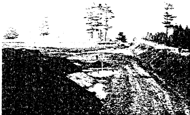
PLATE III. Placement of dredged spoil. In foreground, left to right: spoil material; monitoring well; interior clay dike.
