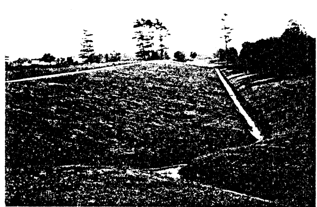
PLATE IV. Completed side slopes with asphaltic concrete paved drains.
