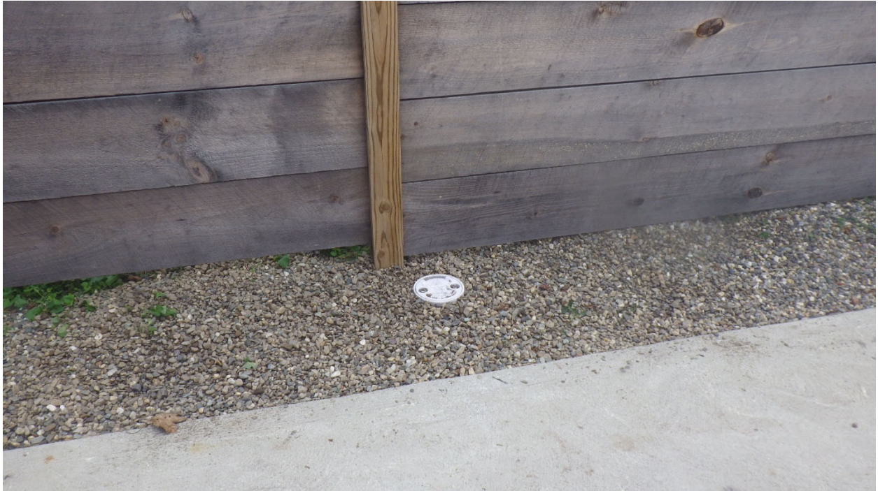
Picture 3: Raise Flushmount MW-04
