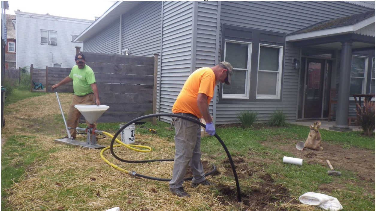
Picture 10: Install New Flushmount MW-03
