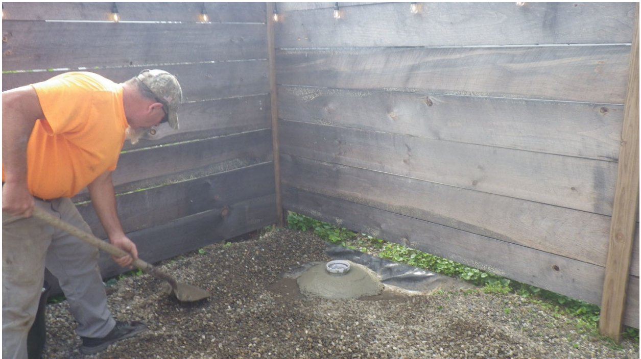
Picture 10: Install New Flushmount MW-03
