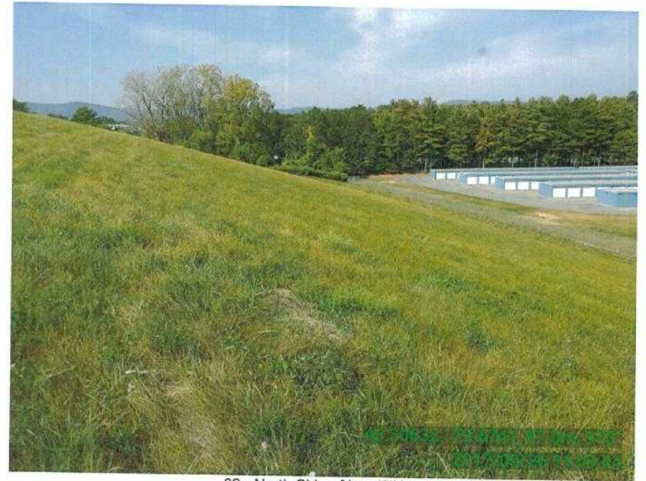
02 - North Side of Landfill.jpg
