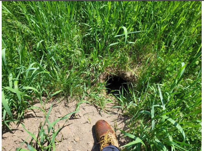
Photo 16: Photo of an animal burrow along the northern perimeter of the landfill cap. Looking south.
