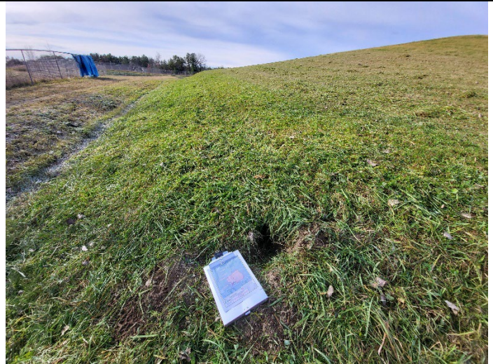
Photo 8: Photo of a small animal burrow near the south-central portion of the landfill cap area, facing west.
