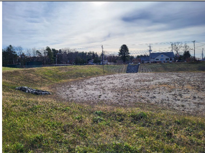
Photo 11: Photo of the retention pond area to the southwest of the landfill, note pond is dry and there is stressed vegetation present. Facing south.
