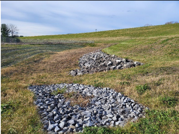
Photo 7: View of the drainage swales near the south-central portion of the landfill, which were dry during the inspection. Facing west.
