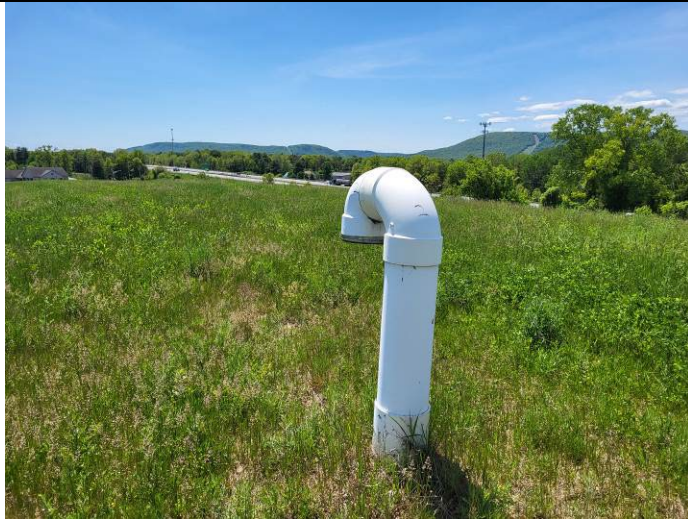
Photo 11: Photo of a passive landfill gas vent. Looking south.
