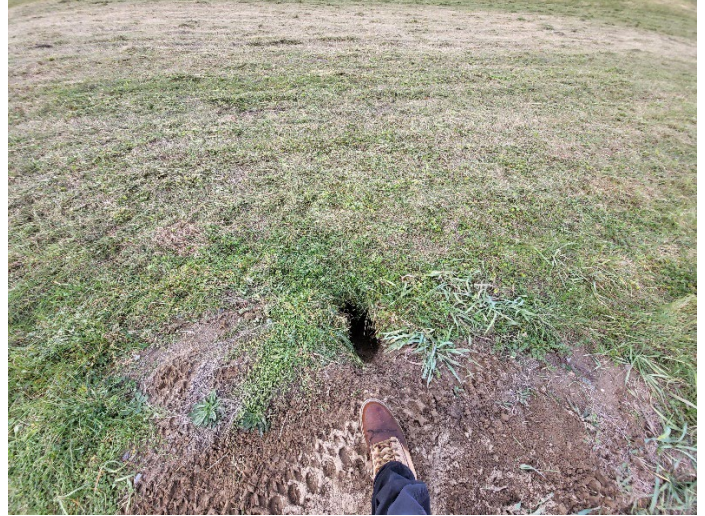
Photo 14: Photo of a small animal burrow, located on the central portion of the landfill cap area. Facing north.
